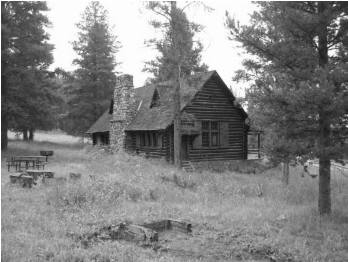
Photo 2. View of the east and south sides of the building.
