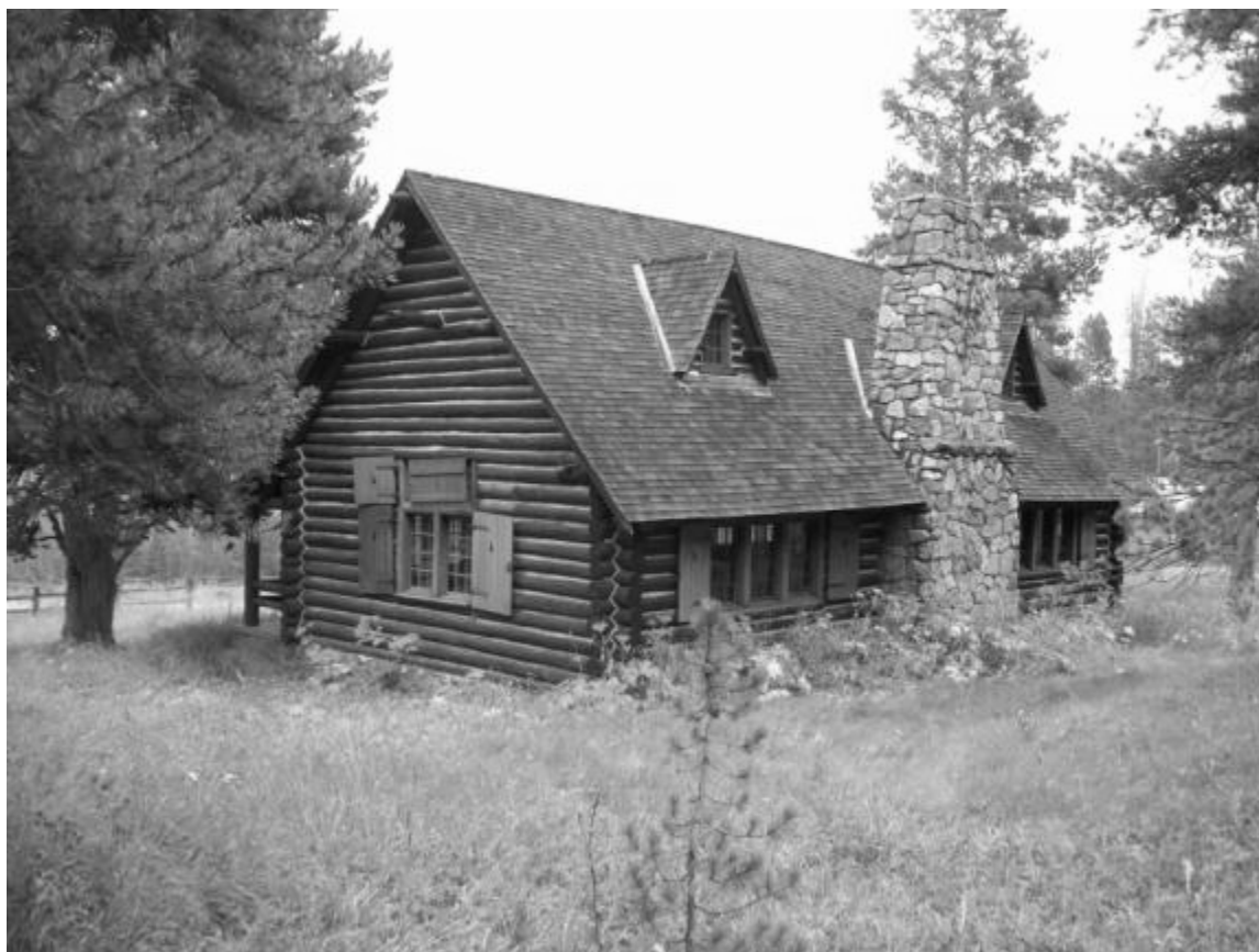
Photo 3. View of the south and west sides of the building.
