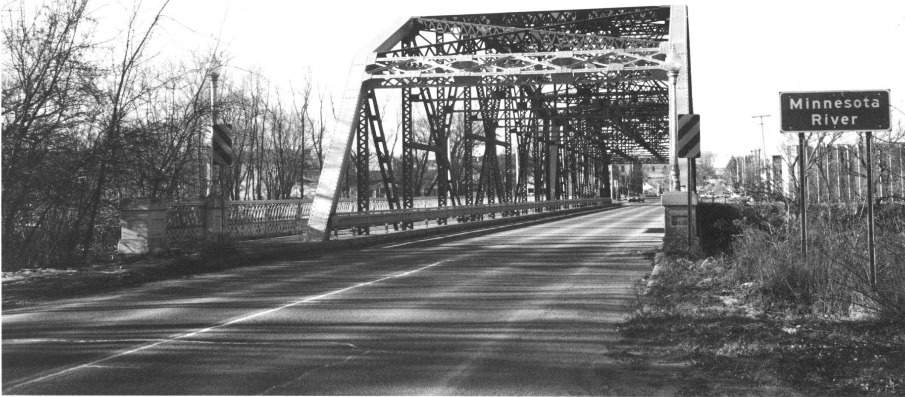
BROADWAY BRIDGE (BRIDGE NO. 4930) LESUEUR and NICOLLET COUNTIES, MN 012838-10A-11
