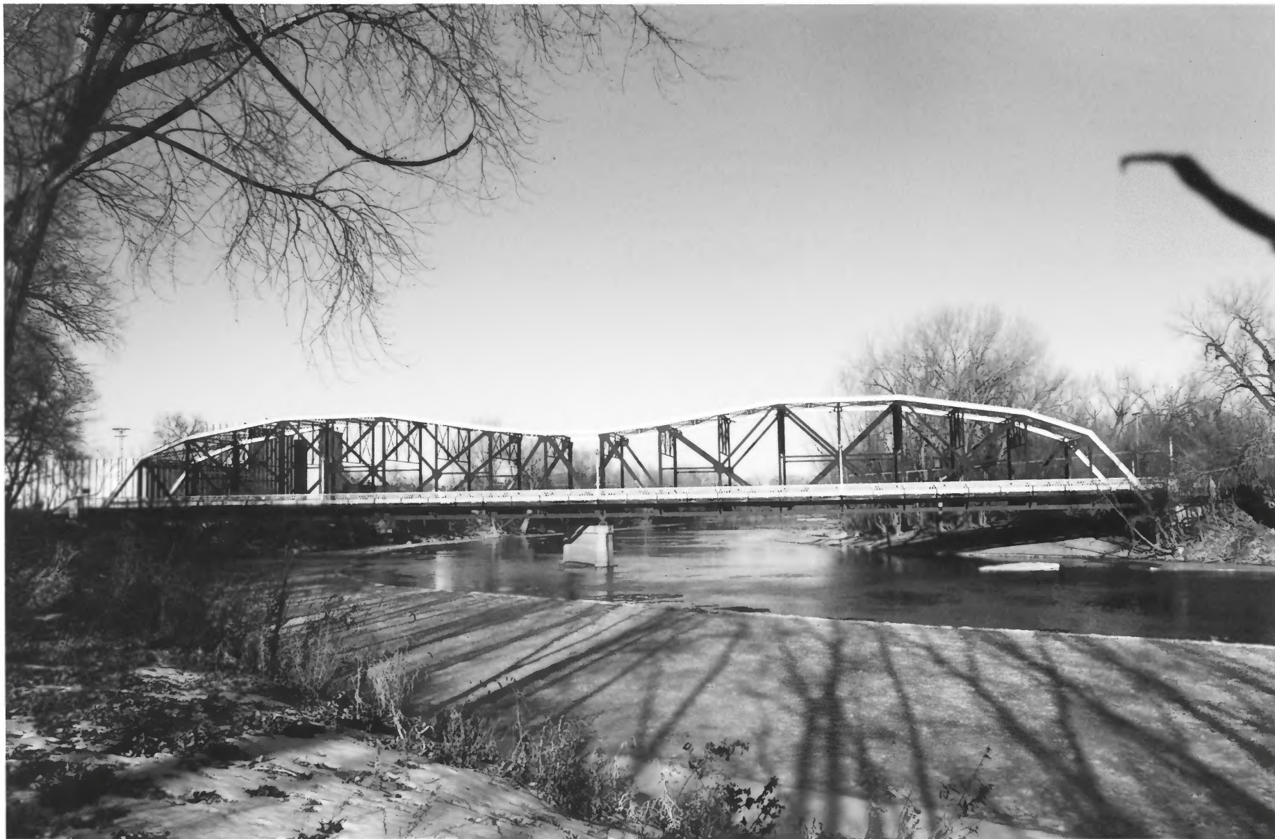
BROADWAY BRIDGE (BRIDGE NO. 4930) LESUEUR and NICOLLET COUNTIES, MN 012838-20A-21
