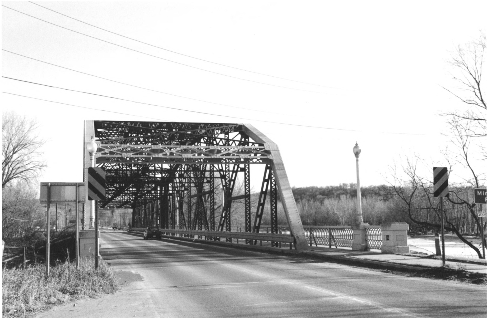
BROADWAY BRIDGE (BRIDGE NO. 4930) LE SUEUR AND NICOLLET COUNTIES, MN 012838-15A-16
