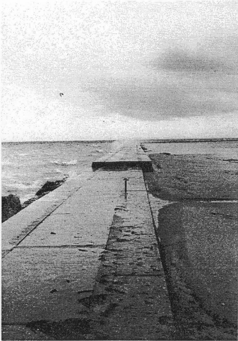
1. South Breakwater, Manistee County, Michigan
