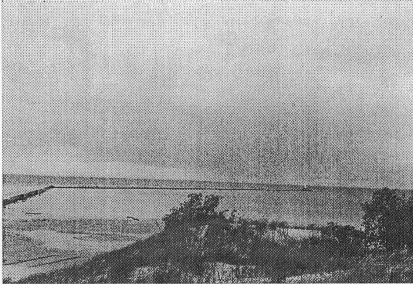
2. South Breakwater, Manistee County, Michigan
