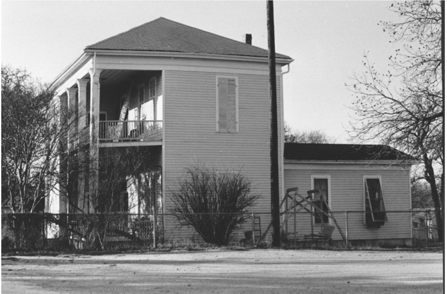
Figure 5: The one-story east wing, added in 1903, is clearly visible in this c. 1980 photo. Note how it is slightly offset from the original house. From the Texas Historical Commission survey files.
