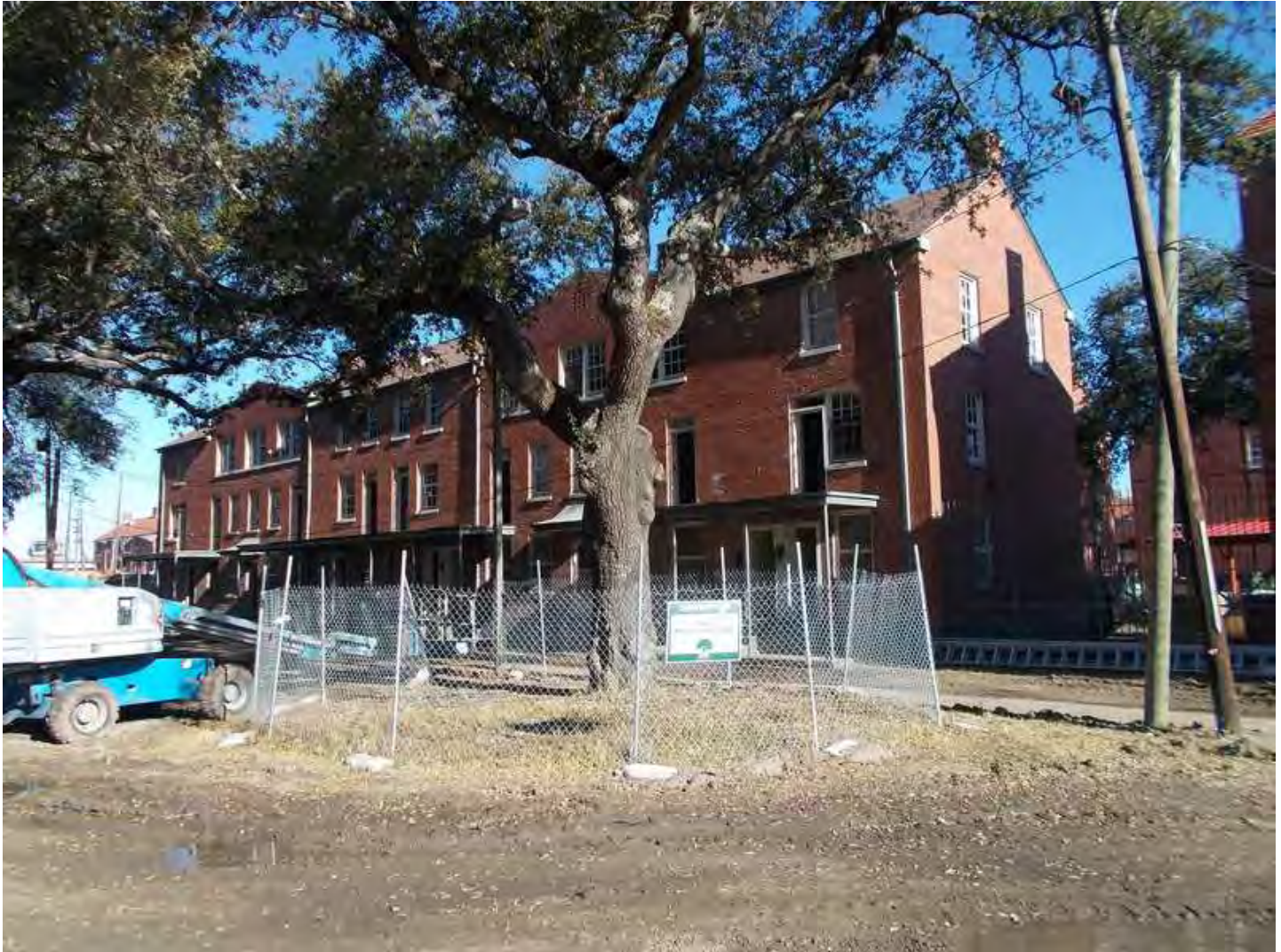
Figure 13. Building #19. Photograph dated: January 29, 2014. Image courtesy of Roderick A. Fifield, AIA.
