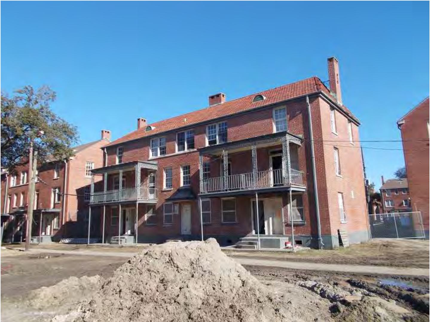
Figure 9. Building #18. Photograph dated: January 29, 2014. Image courtesy of Roderick A. Fifield, AIA.
