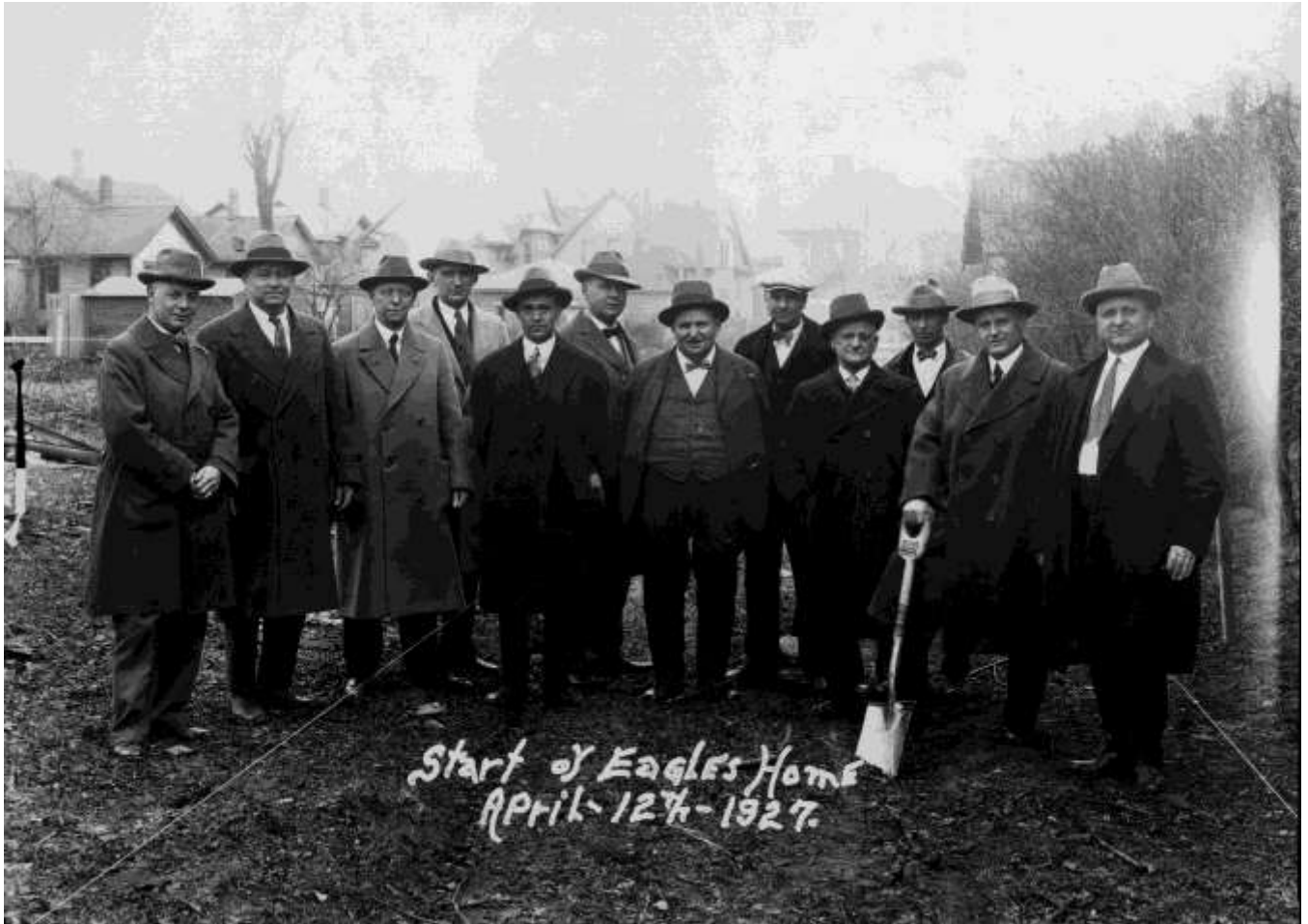
Figure 17: Eagles Club House ground breaking April 12, 1927, from Ben Ganther files
