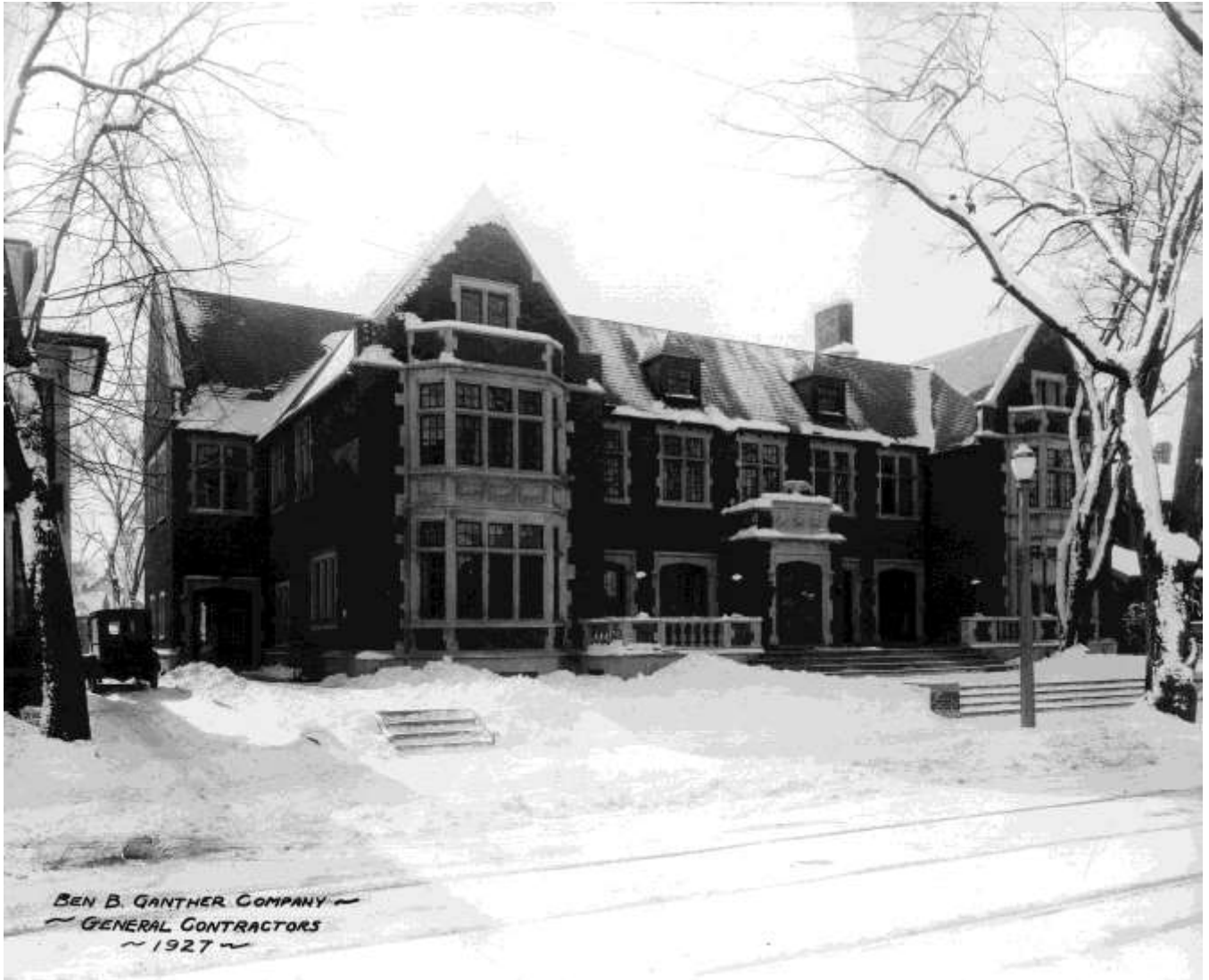
Figure 1: Fraternal Order of Eagles Building, North Facade, December 1927, from Ben Ganther
