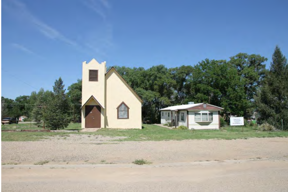
4 of 16. Main elevation with parsonage (mobile home), photographer facing west.
