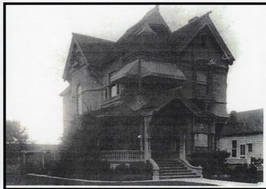
CA_Los Angeles County_James F Cosby House_0012
