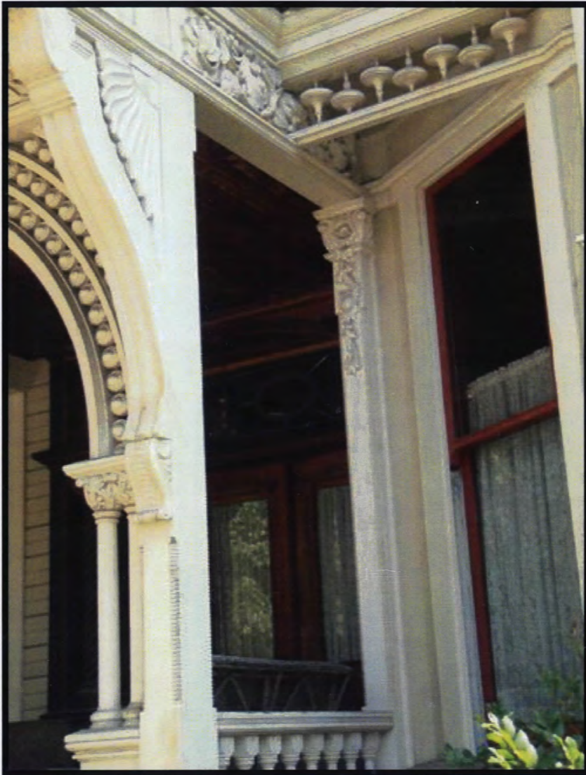
CA_Los Angeles County_James F Cosby House_0005
