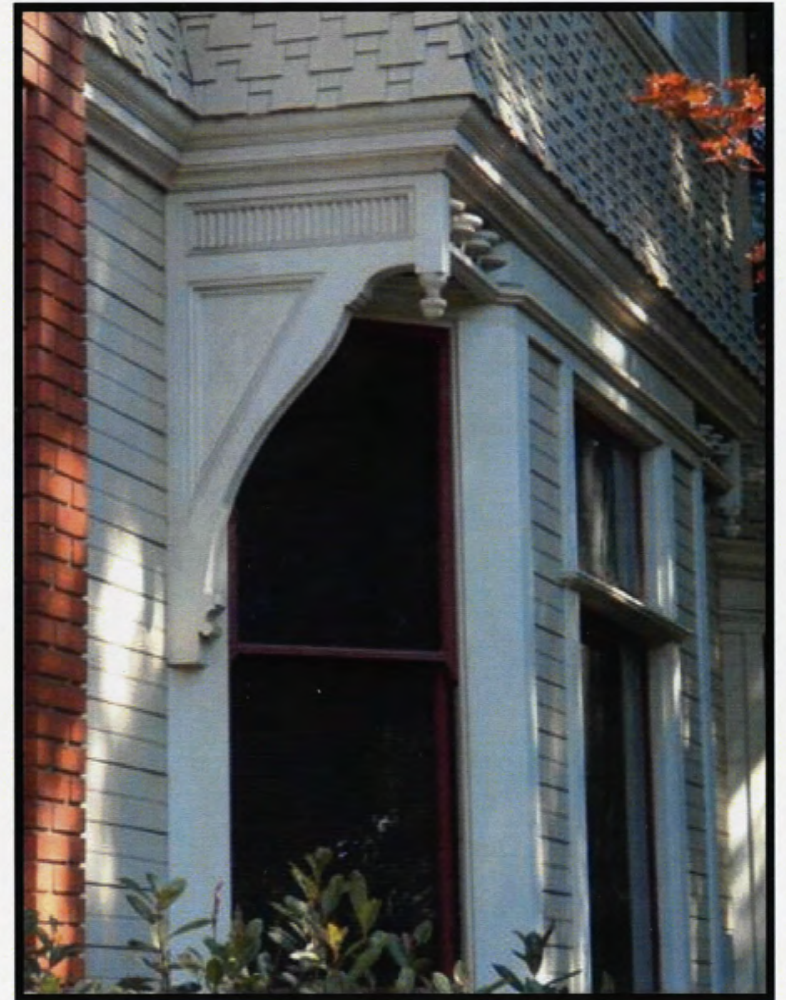
CA_Los Angeles County_James F Cosby House_0008
