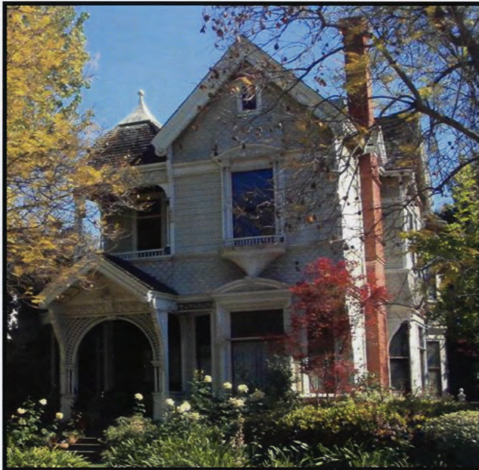
CA_Los Angeles County_James F Cosby House_0001
