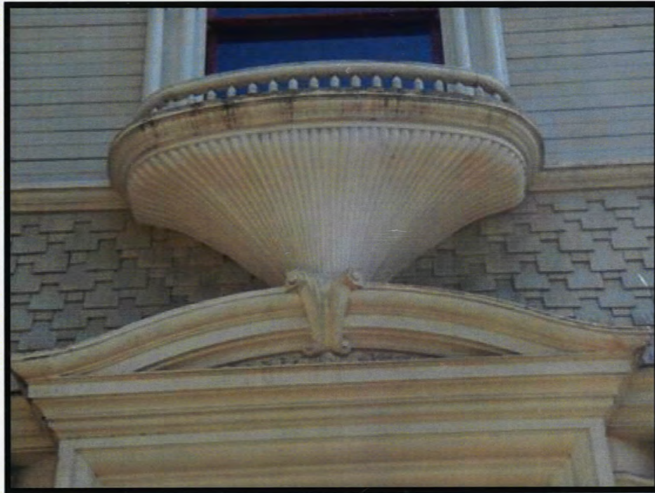
CA_Los Angeles County_James F Cosby House_0007
