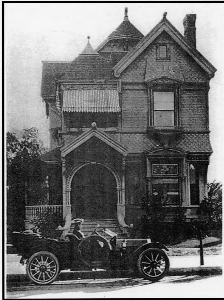
CA_Los Angeles County_James F Cosby House_0013
