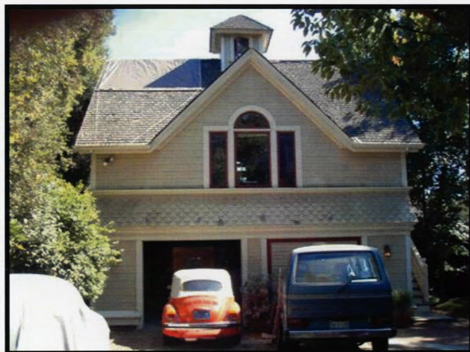
CA_Los Angeles County_James F Cosby House_0011
