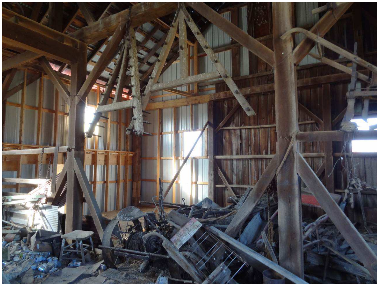
Figure 15. Interior of the bank barn, looking north. Source: MO SHPO Files, 2013.
