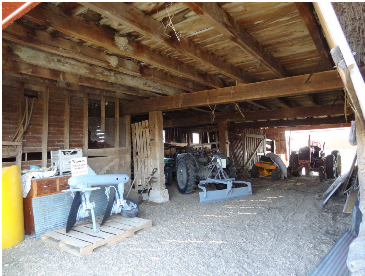
Figure 18. Interior of the Cattle Barn, looking southeast. Source: MO SHPO Files, 2013.
