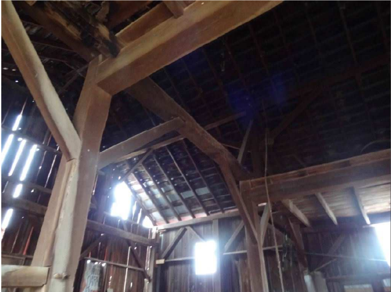
Figure 14. Interior of the bank barn, looking at the posts, collar, and rafter members. Source: MO SHPO Files, 2013.
