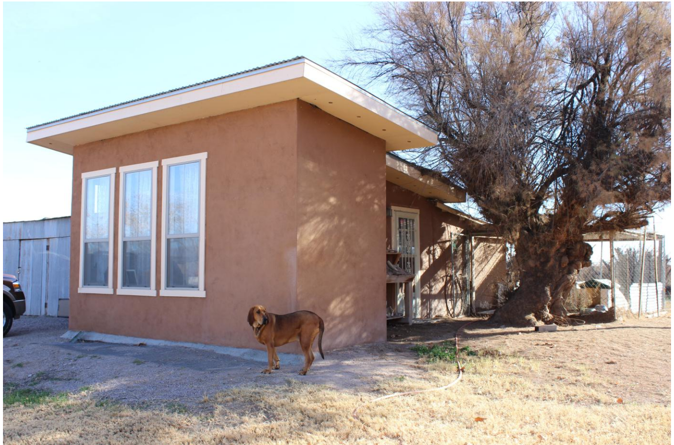
Photo 8 of 8. Well house with shed in background, looking southeast.
