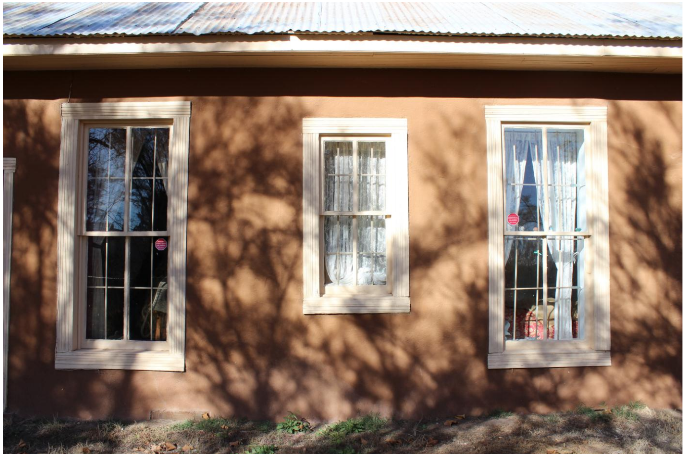
Photo 3 of 8. South elevation window grouping, looking north.
