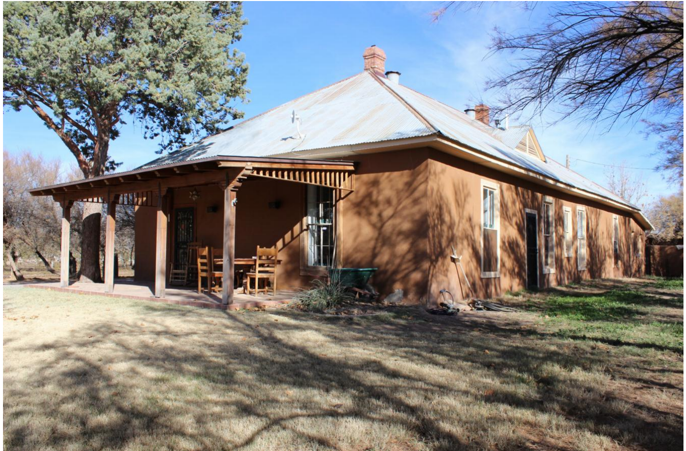
Photo 1 of 8. South and west (front) elevations, looking northeast.
