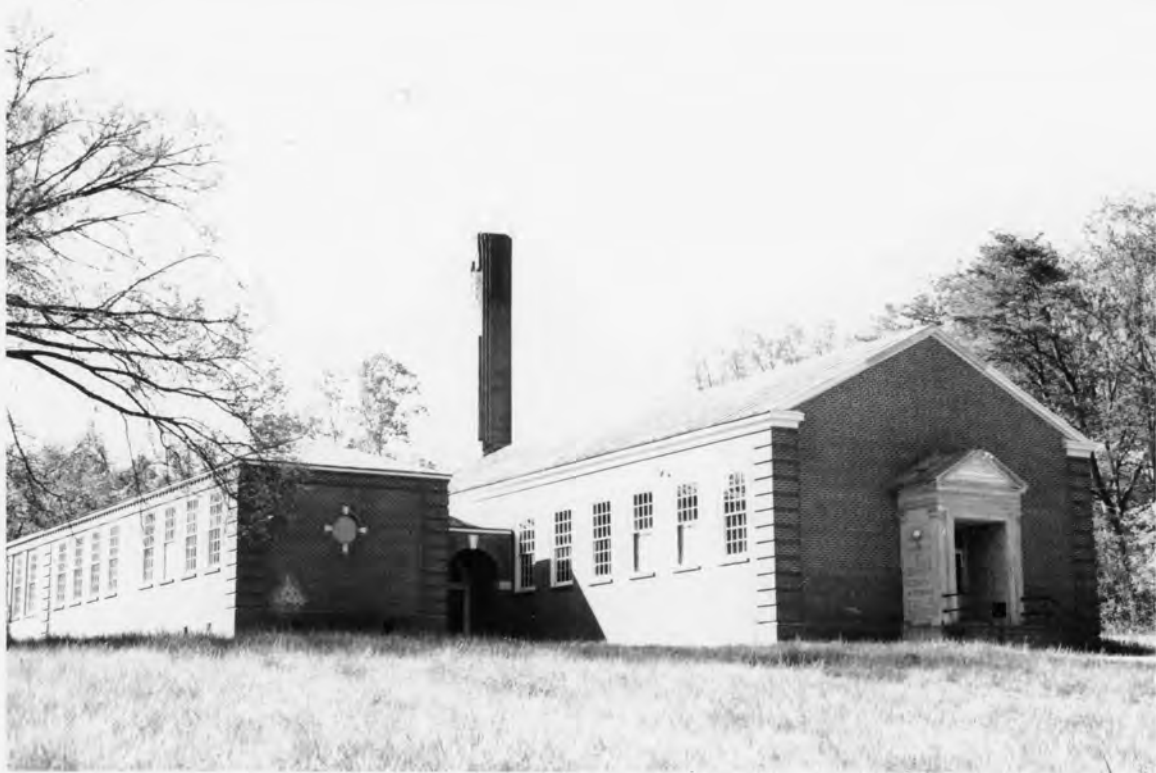
RIVERSIDE SCHOOL 30F21 KNOX COUNTY, TN
