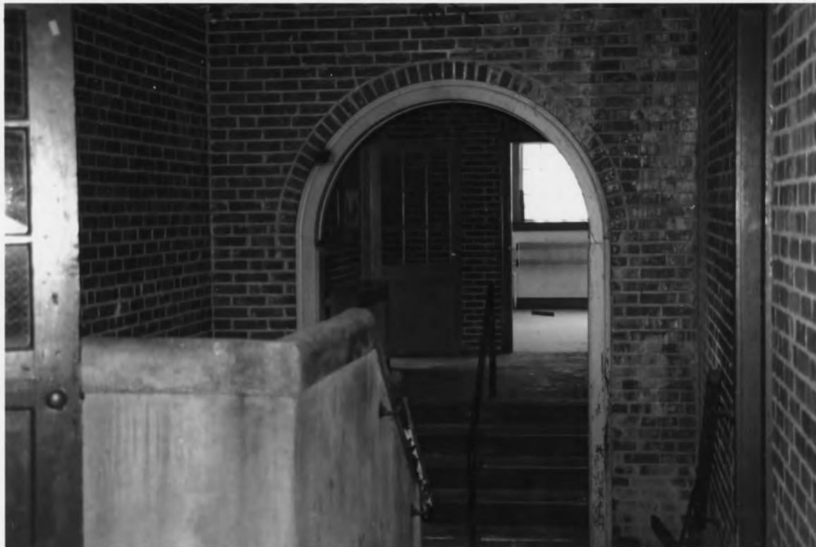
RIVERSIDE SCHOOL KNOX COUNTY TN 140f21
