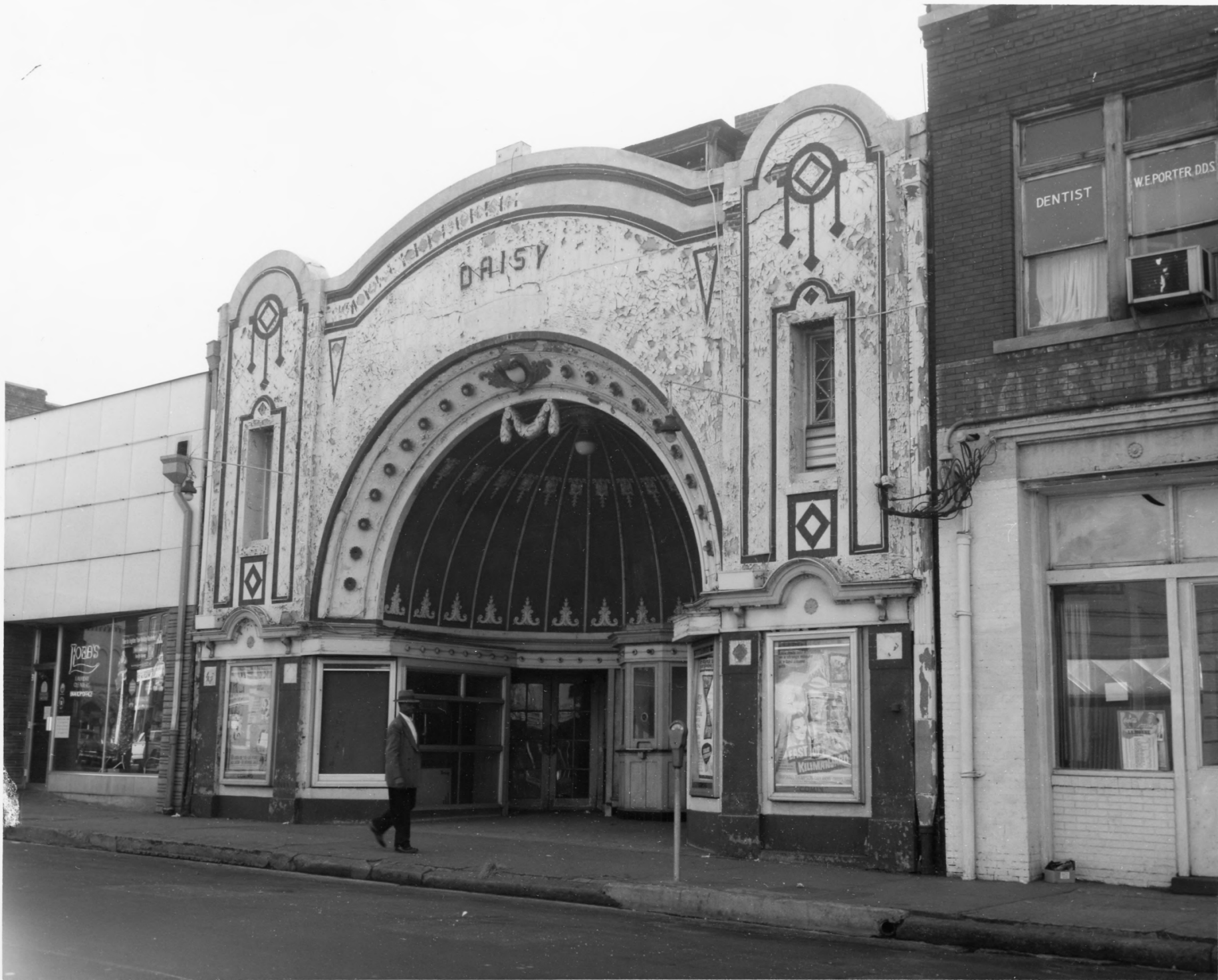
Beale Street Historic District-- Old Daisy Theater, December 23, 1965 (300 Block of Beale Street) National Park Service photograph
