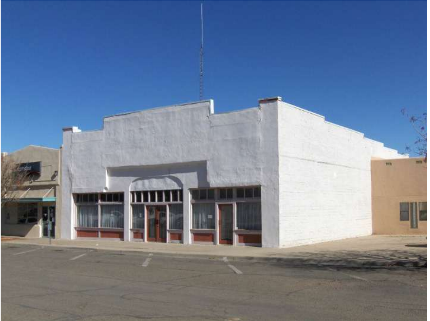
Photo 12 Deming Transfer Co. Building 105-107 N Silver Ave
