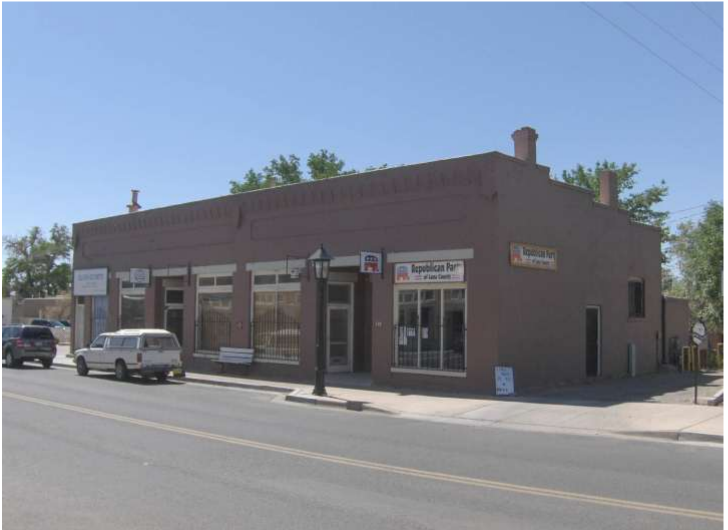
Photo 17 Commercial Building 112-120 E Spruce St
