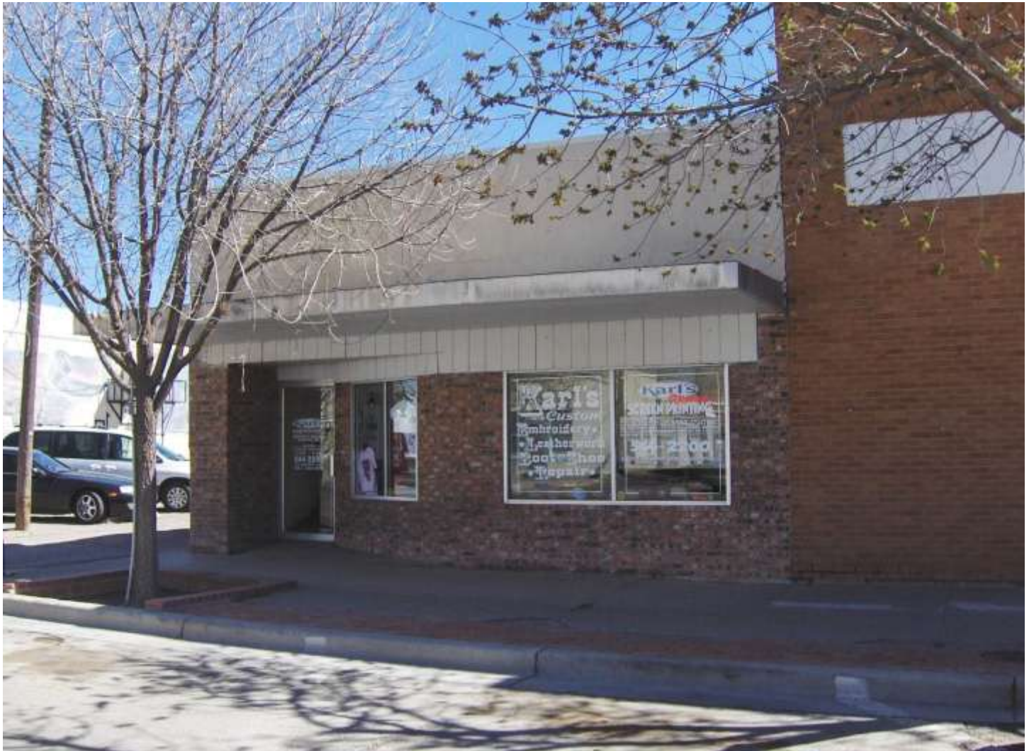
Photo 19 Commercial Building 113 S Silver Ave
