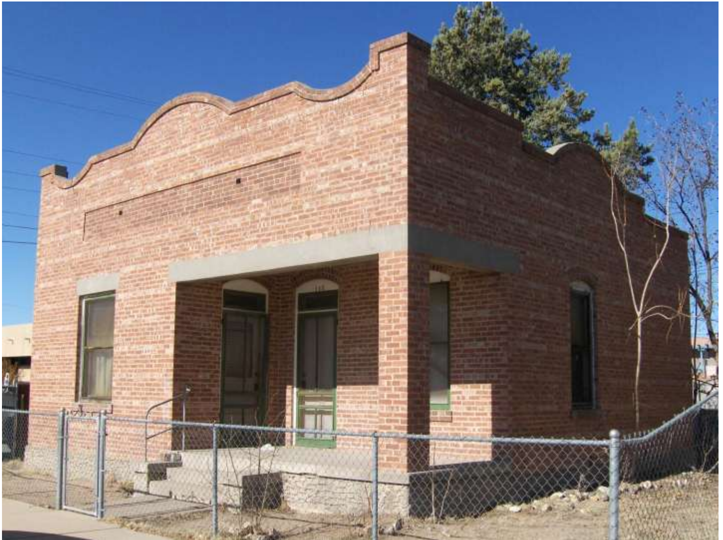
Photo 5 House 113 East Maple Street
