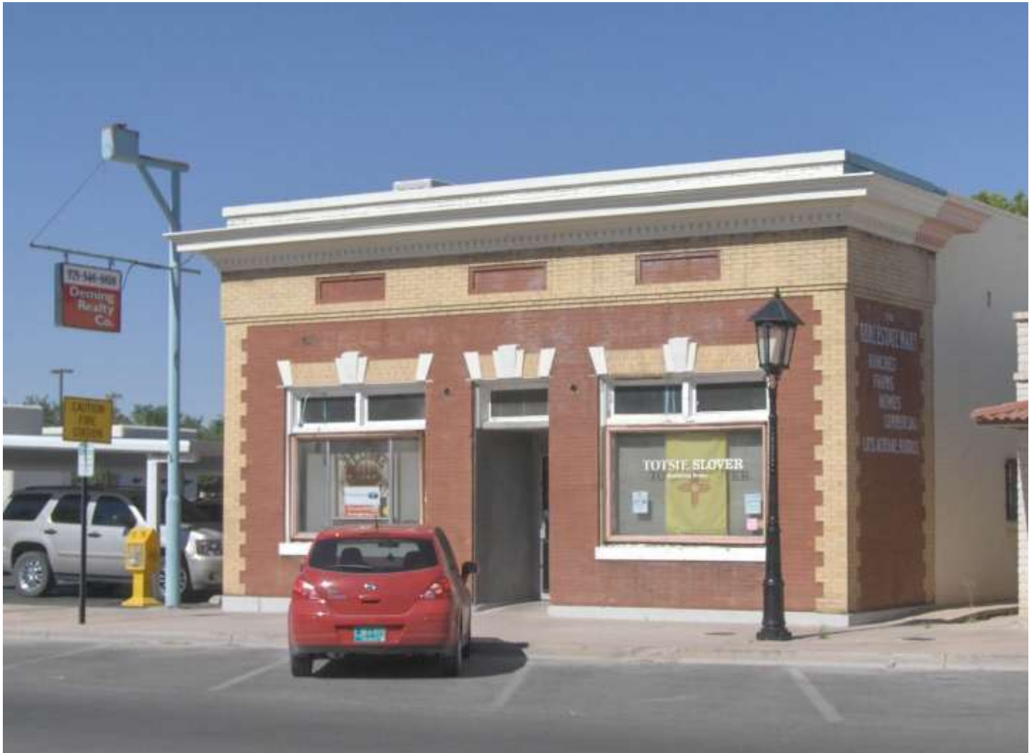
Photo 4 Mtn. States Telephone & Telegraph Co. Building 220 S Gold Ave
