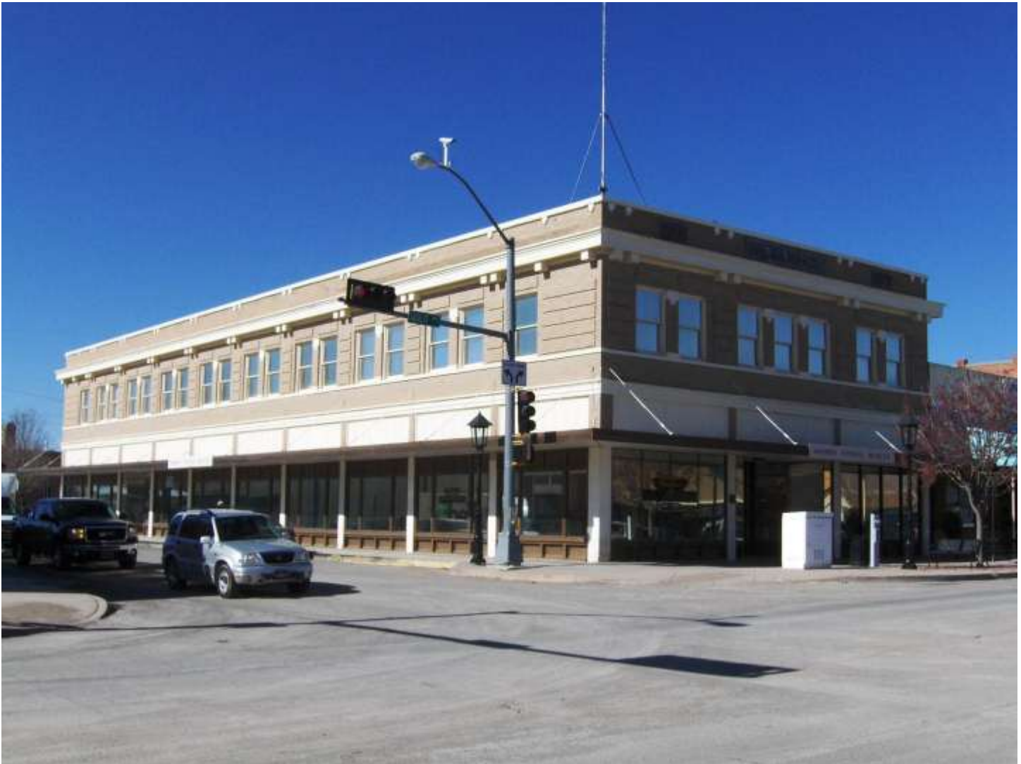
Photo 2 J.A. Mahoney Building 122 S Gold Ave
