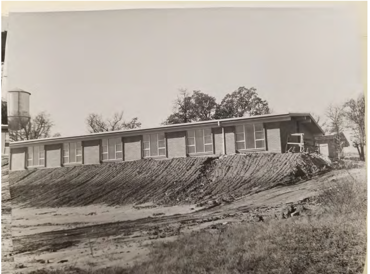
Fairhaven Retirement Home View of the east wing from the northeast 1964
