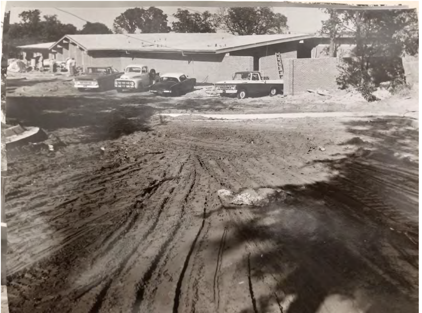
Fairhaven Retirement Home View of the west wing from the southwest 1964
