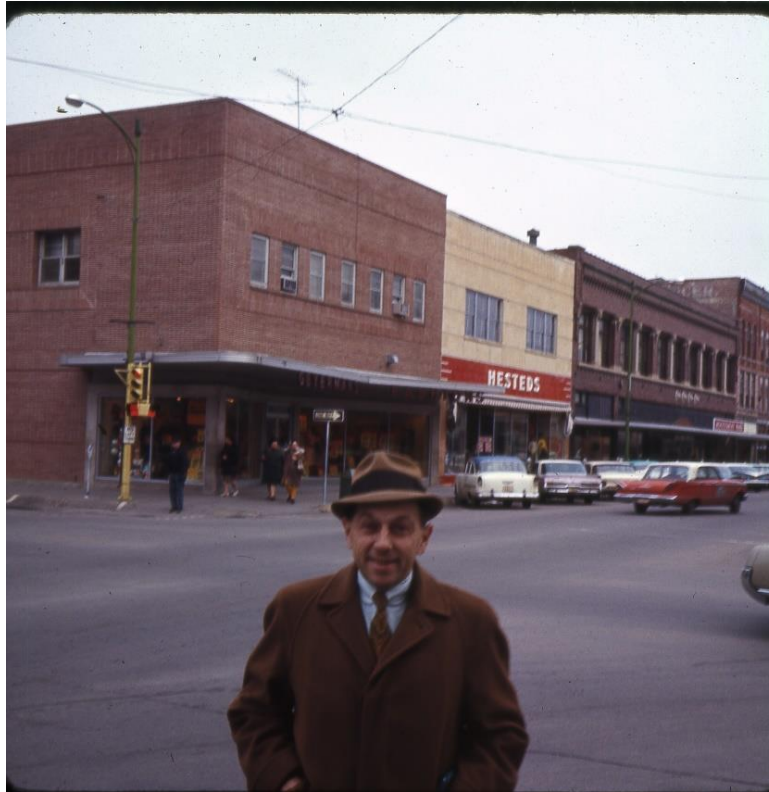
The former German National Bank at 642 West 2nd Street. The 1951 remodel removed the Victorian Era cornice and façade details replacing them with a streamlined thin textured brick façade, an effort at banded windows, and a unique awning. Photo c. 1960 courtesy of Adams County Historical Society
