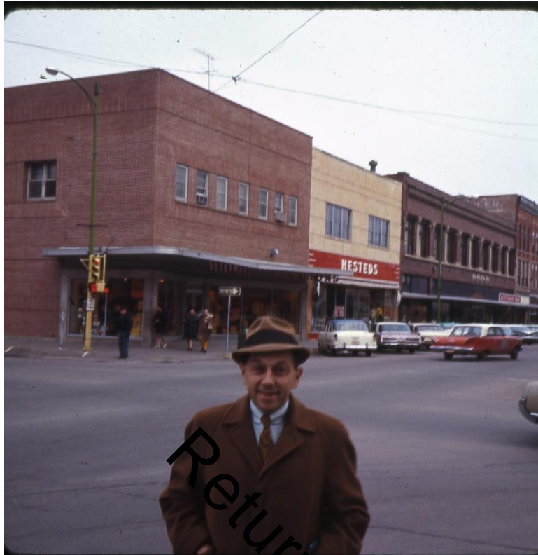
The former German National Bank at 642 West 2nd Street. The 1951 remodel removed the Victorian Era cornice and façade details replacing them with a streamlined thin textured brick façade, an effort at louvered windows, and a unique awning. Photo c. 1960 courtesy of Adams County Historical Society
