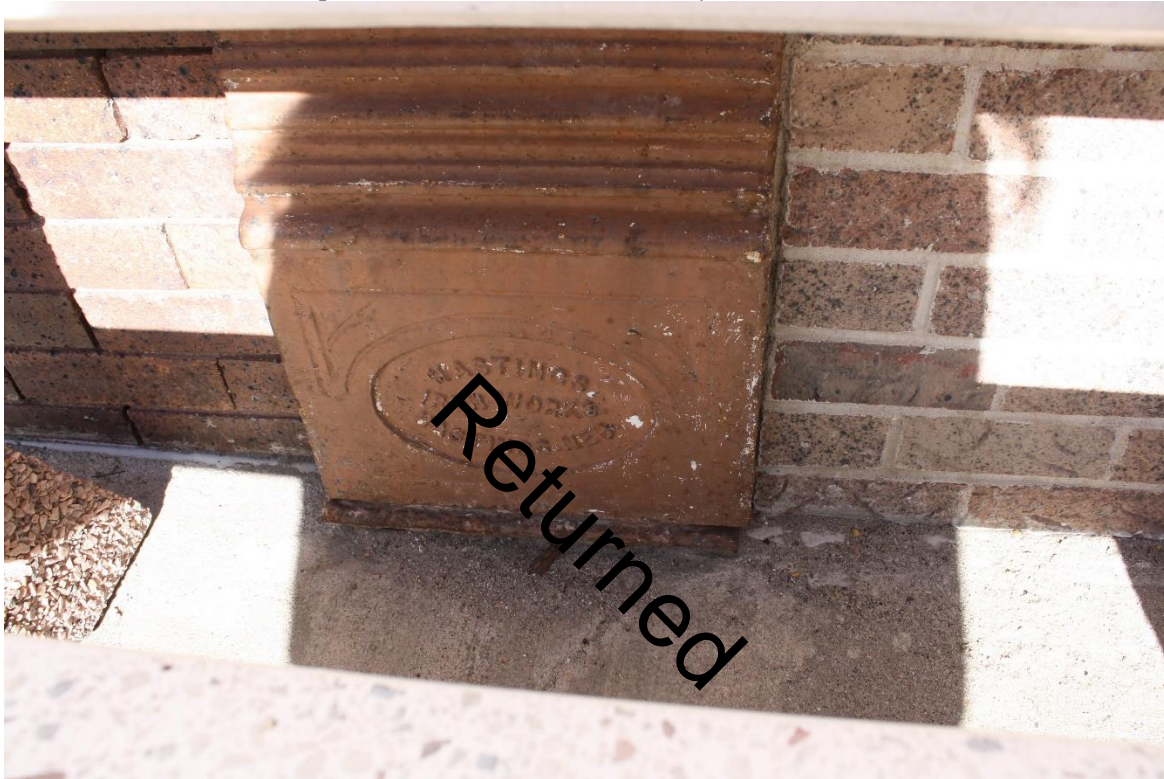
Hastings Iron Works column base at Stein Building on West 2nd Street.
