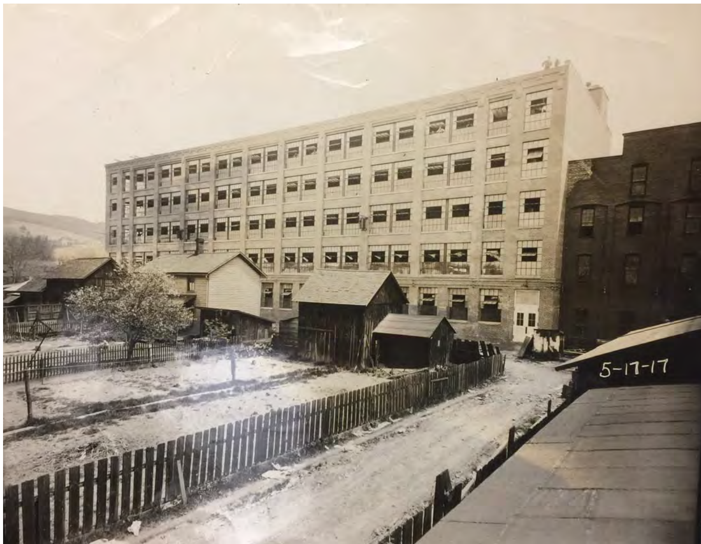
05-17-1917 Construction Photo of Building H (left), with Building B (right); looking northeast; Lycoming Rubber Company; Lockwood Greene Records, Archives Center, National Museum of American History, Smithsonian Institution
