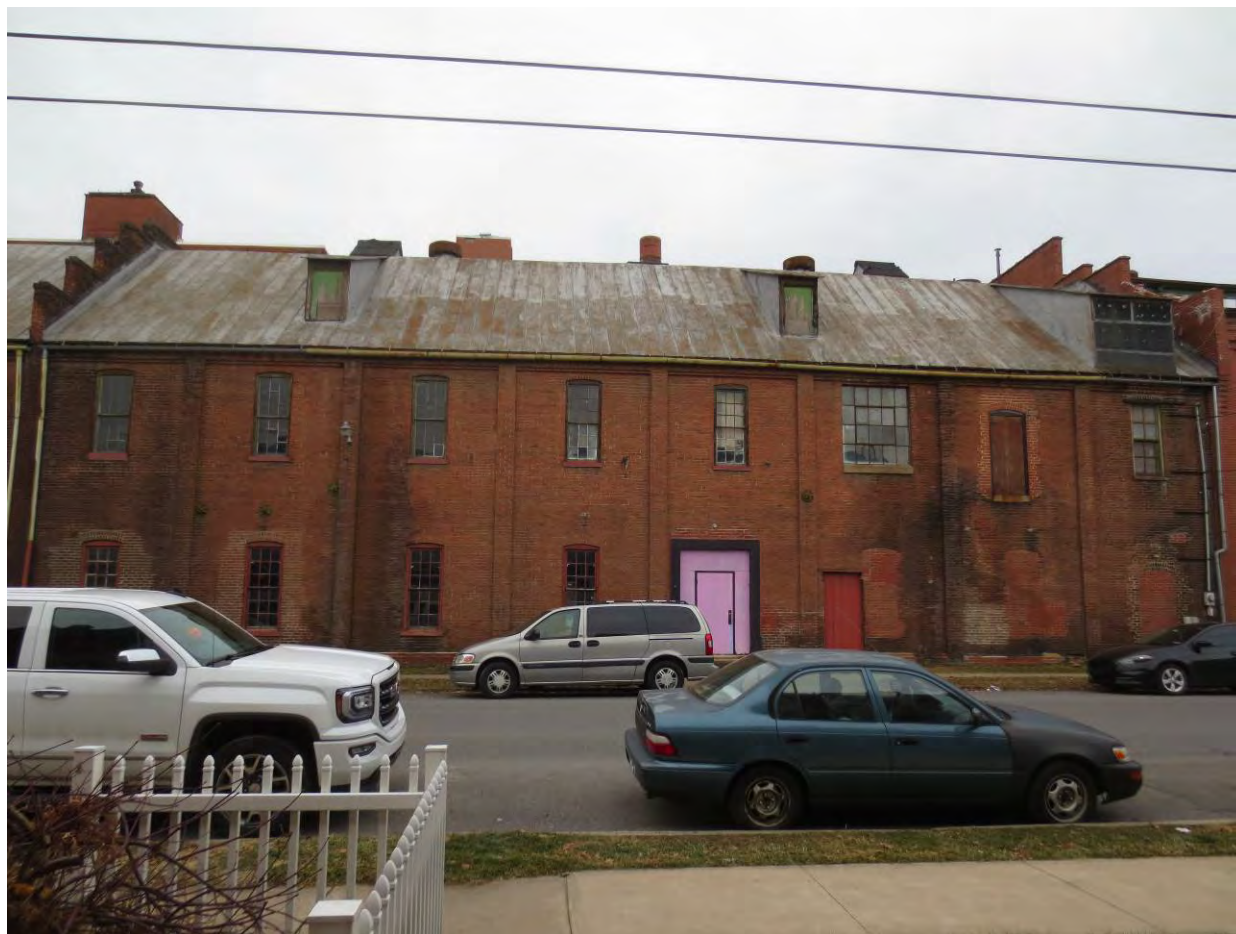
Photo 22. East Elevation of Building D extension
