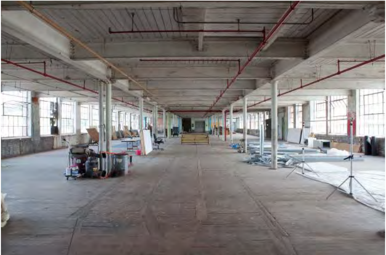
Photo 68. View of 4 th floor looking south toward firewall of Building H.
