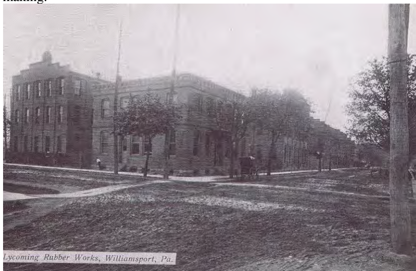
Figure 20. Postcard view of stepped gable annex at left, before the company office at right was demolished.
