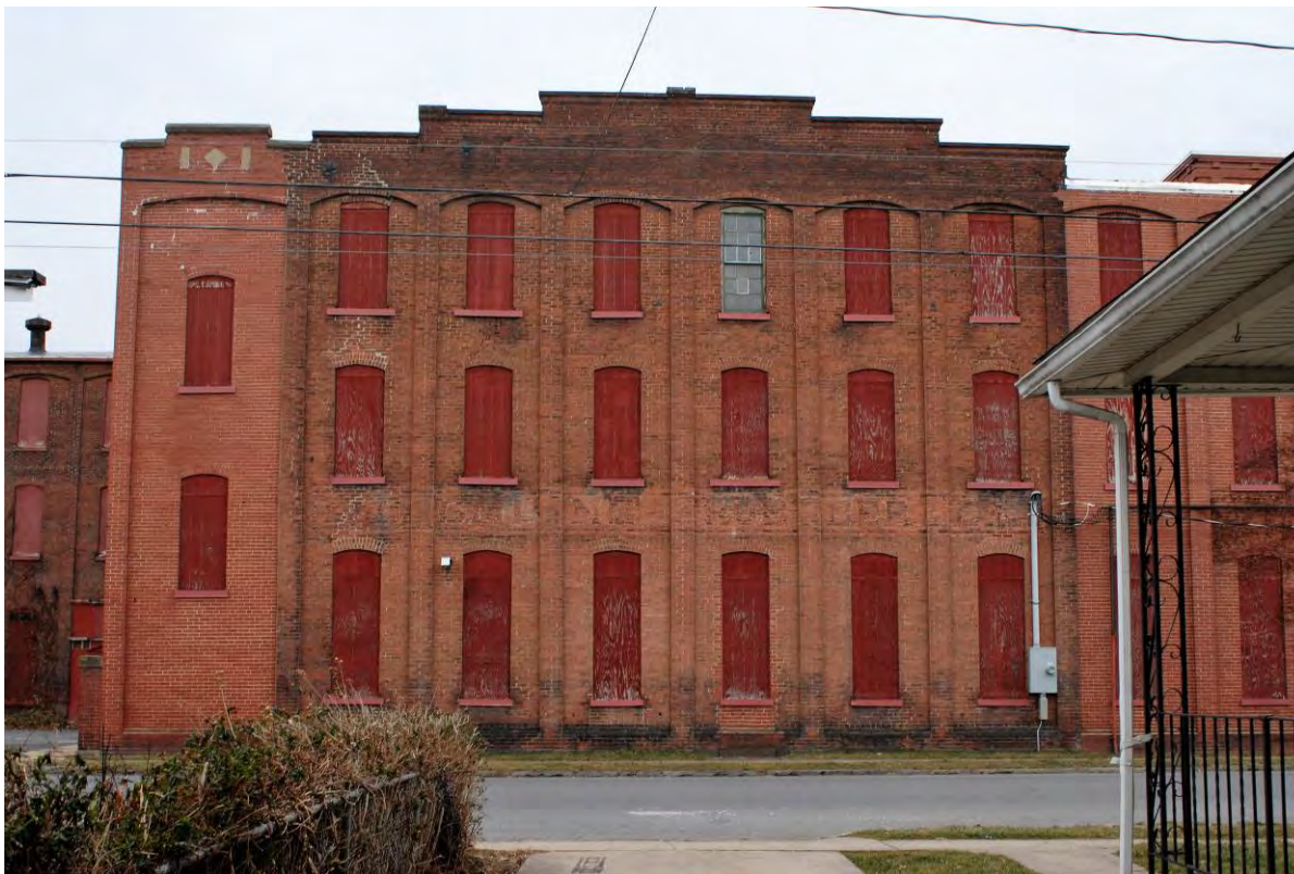
Photo 1. East Elevation of Building A, with 1918 stair tower addition (left) and mill room extension (right).
