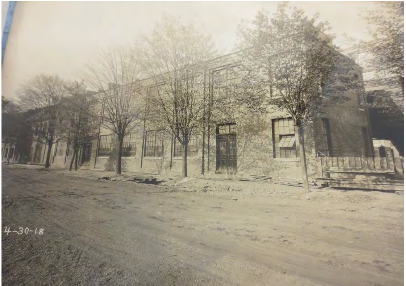
04-30-1918 Construction Photo of Building K (foreground), Building H (background); Lycoming Rubber Company; looking southwest from Rose Street; Lockwood Greene Records, Archives Center, National Museum of American History, Smithsonian Institution
