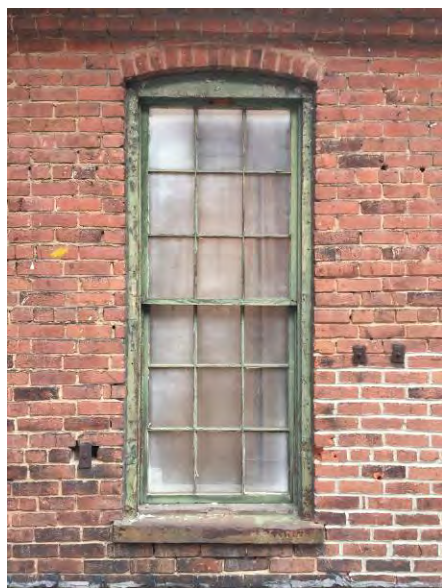
Photo 23. Detail of 2 nd floor window
