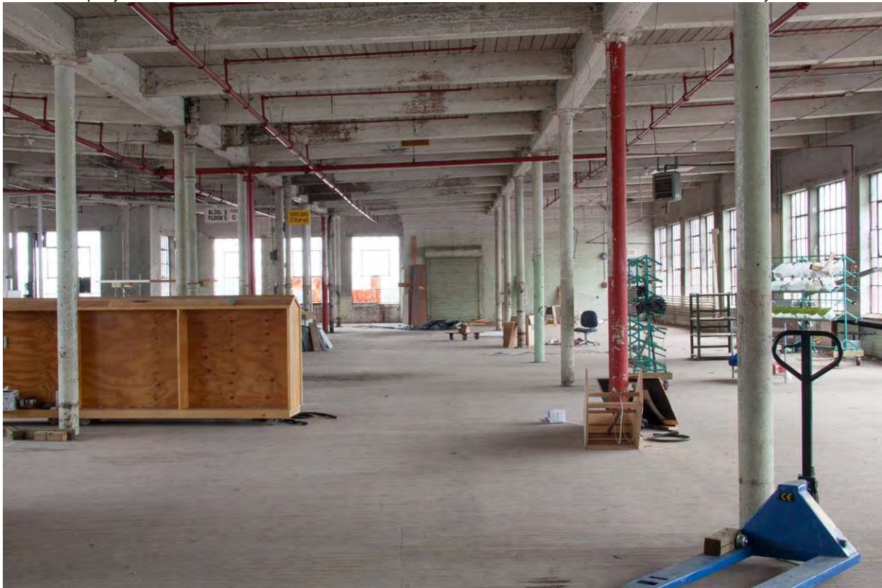
Photo 83. View of 5 th floor of New Building C looking east.
