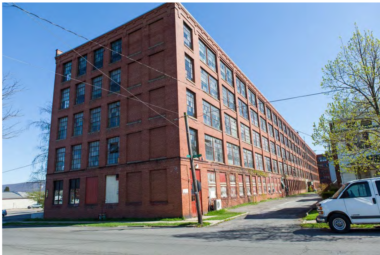
Photo 60. View of the northwest corner of Building L taken from Park Avenue north of Allen Street, showing the seamless 1918 extension of the west facade facing Allen Street north of the firewall of the 1917 manufacturing building on the right, and the north elevation of the 1918 extension facing Rose Street on the left.
