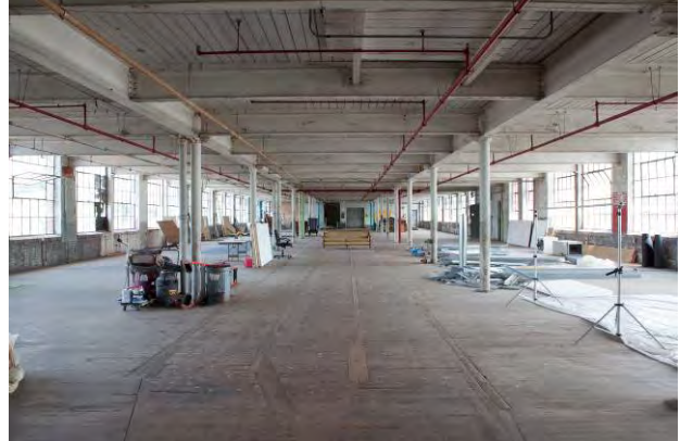
Photo 48. 4 th floor of Building H looking north
