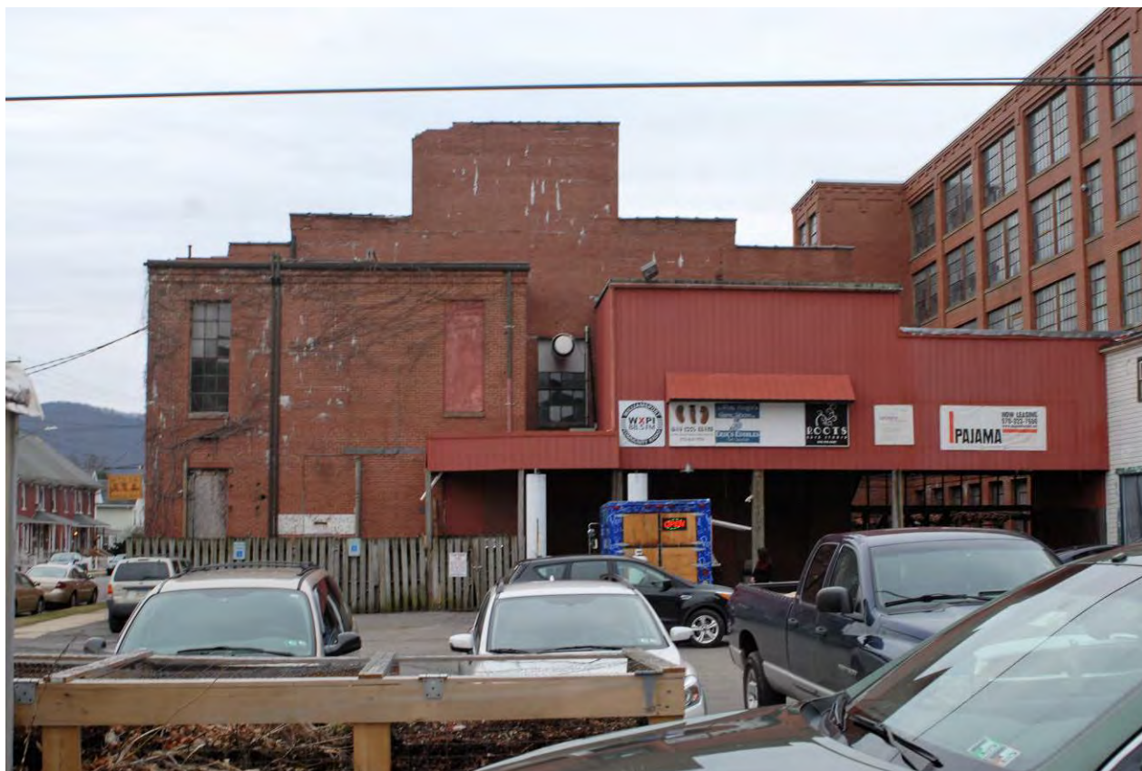
Photo 51. North elevation of Building K
