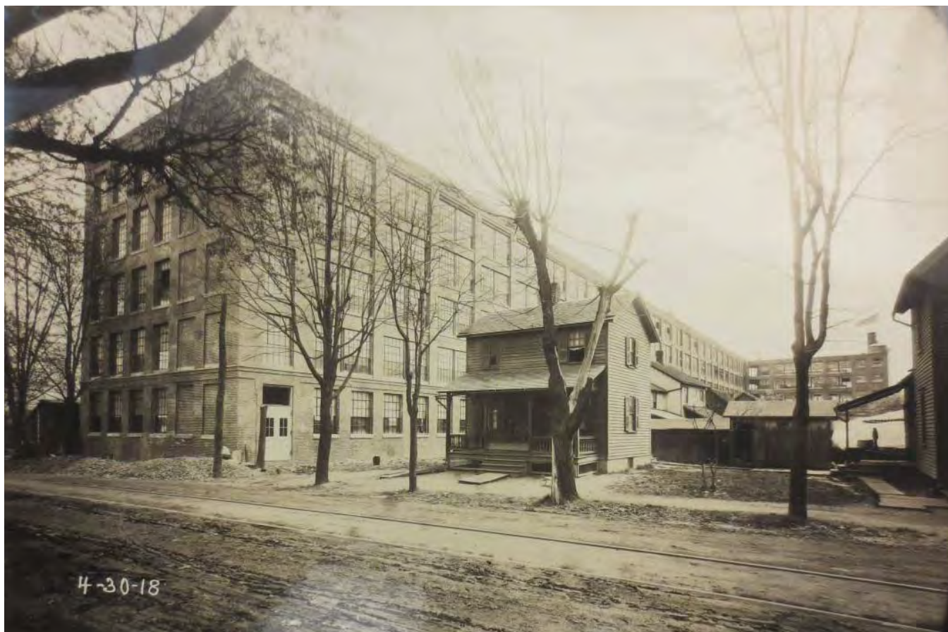
04-30-1918 Construction Photo of Building L (foreground), Building H (center) and Building C (background); Lycoming Rubber Company; looking southeast from Park Avenue west of Allen Street; Lockwood Greene Records, Archives Center, National Museum of American History, Smithsonian Institution
