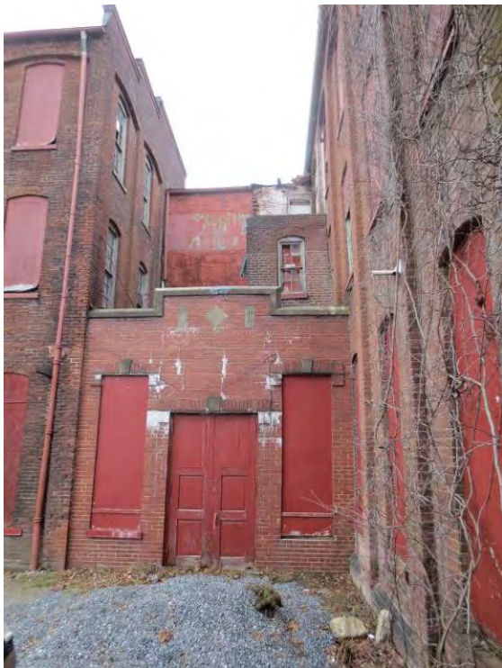
Photo 32. 1918 Infirmary and toilet tower beyond
