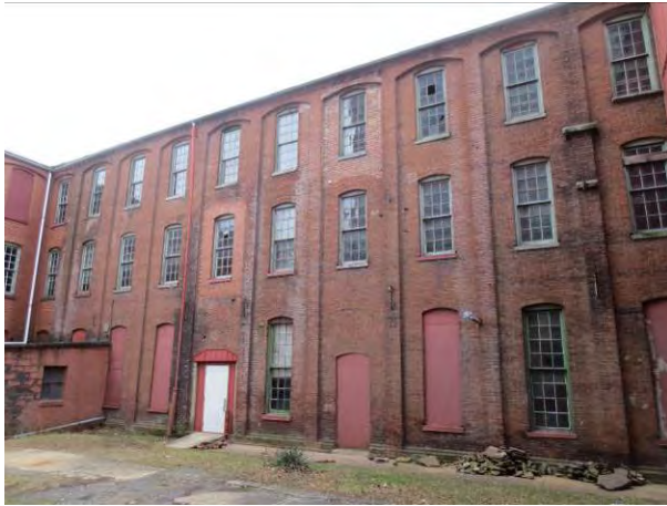
Photos 5. & 6. North elevation east and west of the 2-story bridge connecting Building A to Building C. The east end of the north elevation abuts the 1918 Building A extension, visible at the far right of Photo 5. An original doorway at the ground level of the engine room at the west end of the north elevation has been partially filled in with brick to accommodate a standard size metal door with a vision panel, and the ground floor window in the 4 th bay from the west end has been enlarged to provide an entrance door that is now covered with plywood.
