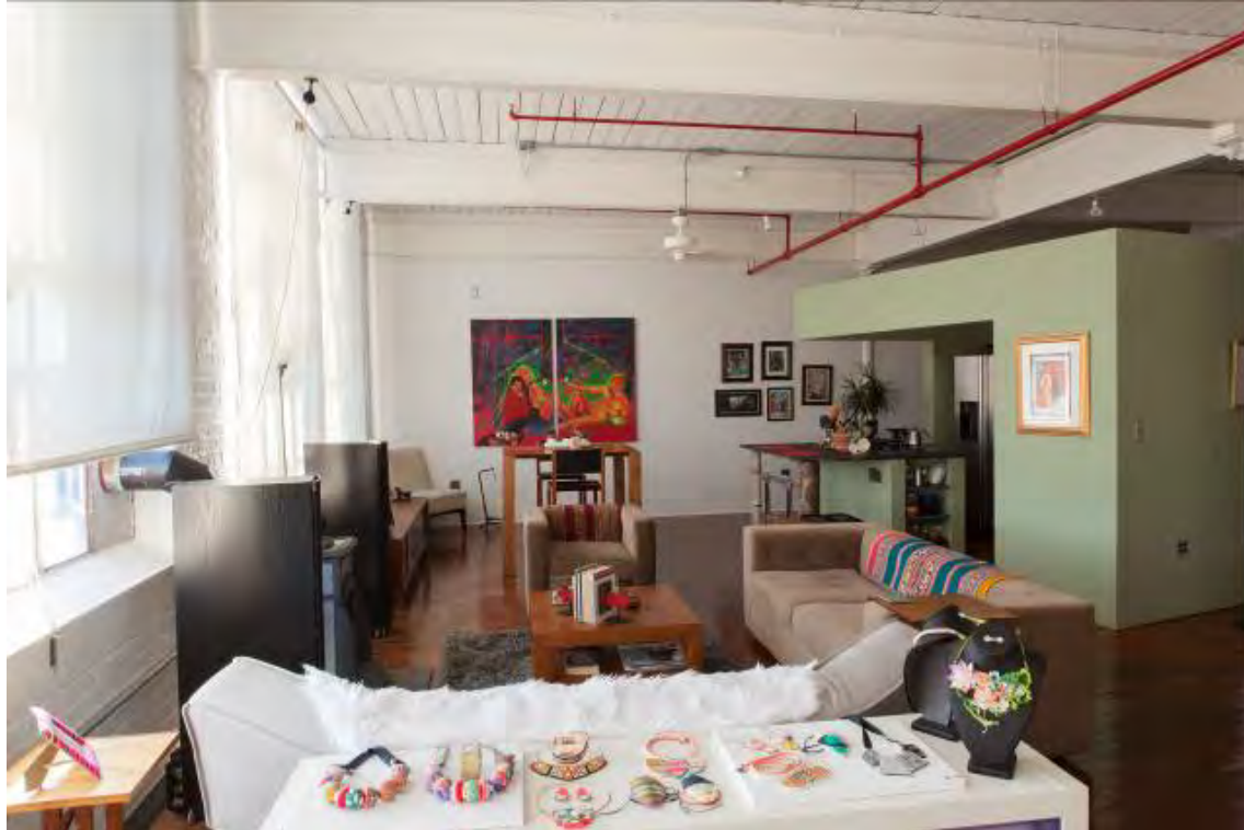
Photo 81. View of 4 th floor live-work space looking west. The green divider floating in the space beneath the structure encloses the kitchen. Original sprinkler pipes throughout the building are painted red in keeping with the color-coded system devised by Lockwood Greene & Co. Engineers for the Lycoming Rubber Company.
