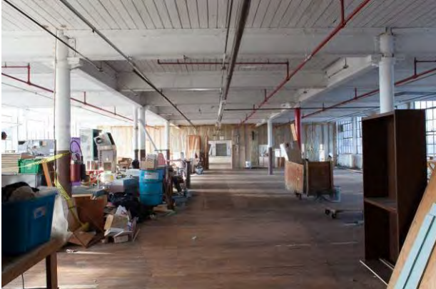
Photo 47. 3 rd floor of Building H looking north
