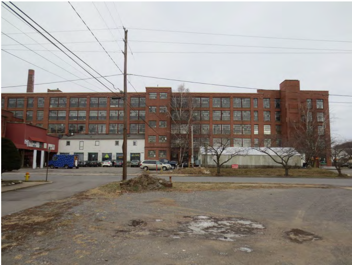
Photo 61. East (Rose Street) elevation of Building L
