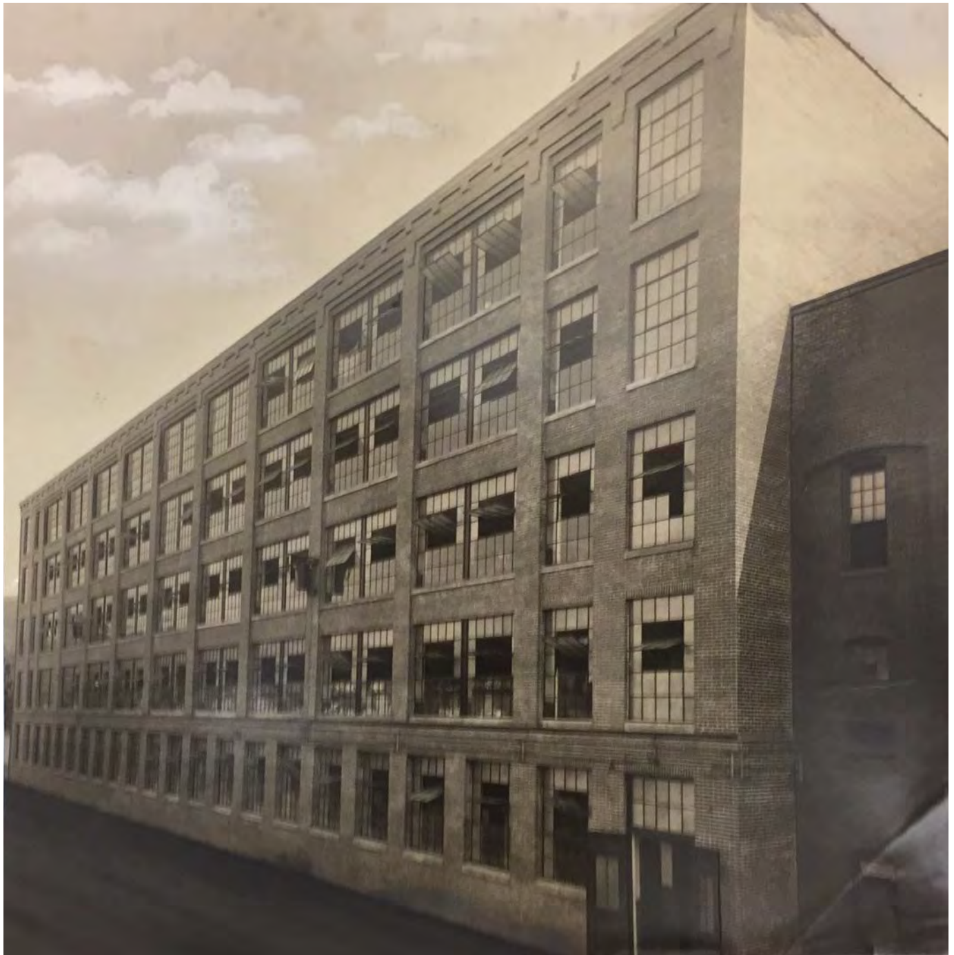
Circa 1917 Construction Photo of Building H (left), with Building B (right); looking northeast; Lycoming Rubber Company; Lockwood Greene Records, Archives Center, National Museum of American History, Smithsonian Institution
