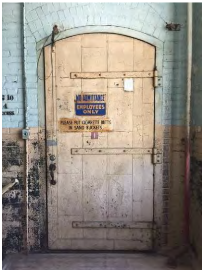
Photo 84. View of tin clad fire door with self-closing pulley and cable hardware and heavy duty face mounted metal strap hinges in stair tower, typical throughout the property.
