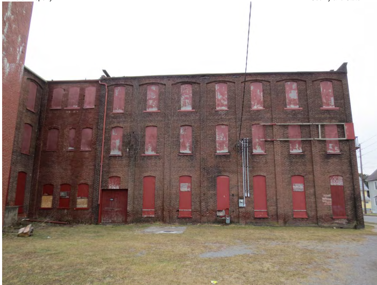
Photo 30. West (Cemetery Street) elevation of Building F.
