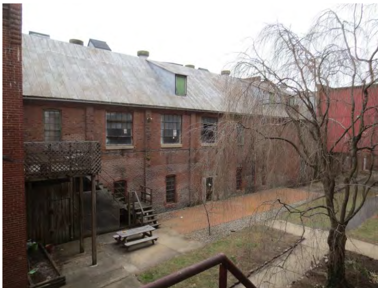
Photo 24. View of Courtyard Elevation of Building D extension
