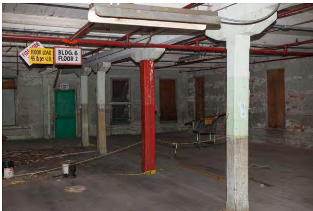
Photo 35. 2 nd floor of Building F looking south
