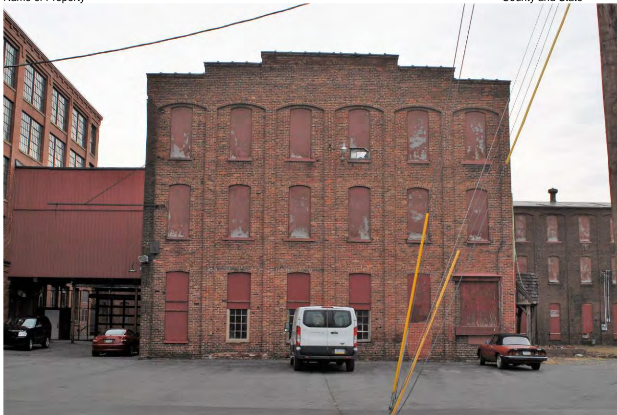
Photo 4. West Elevation of Building A, with the 2-story bridge connecting Building A to Building C beyond at left and the west elevation of Building F visible beyond at right.
