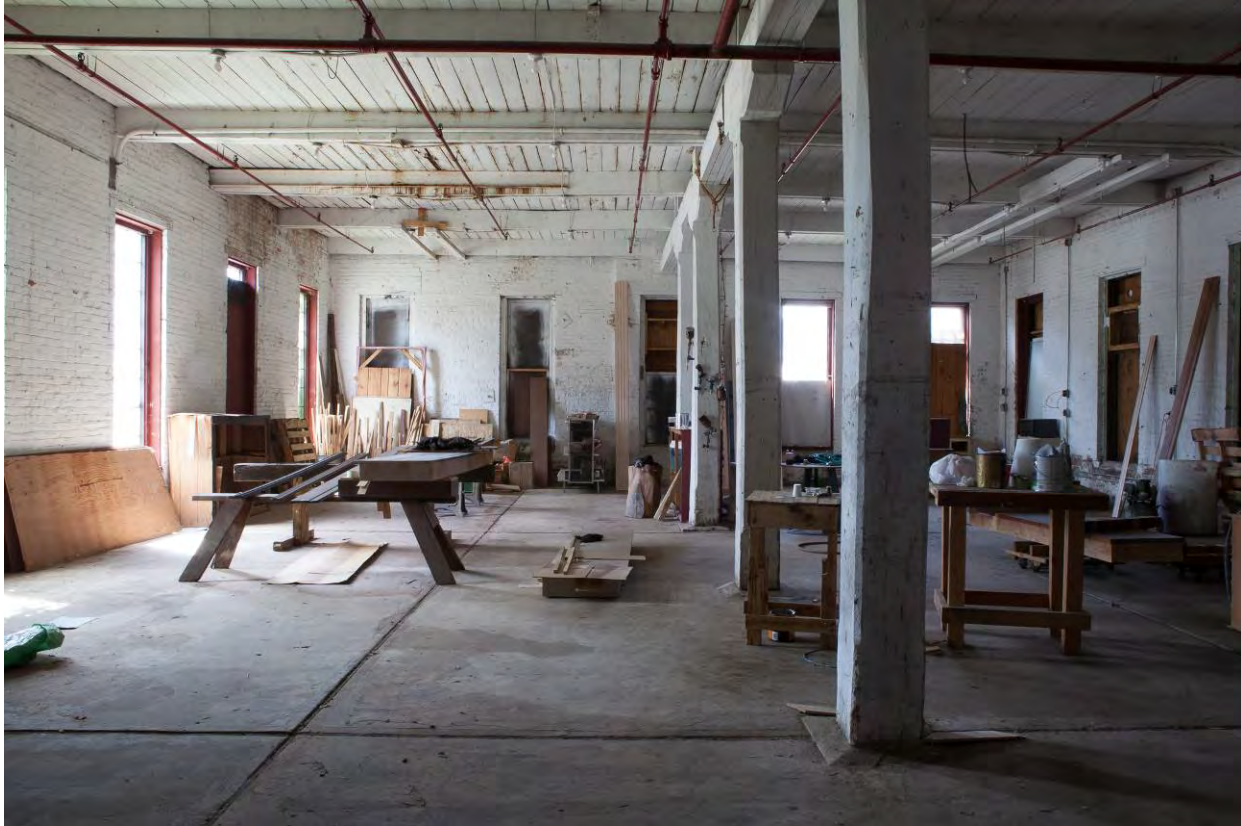
Photo 34. Ground floor of Building F looking south. Note corners of columns chamfered to improve fire resistance.
