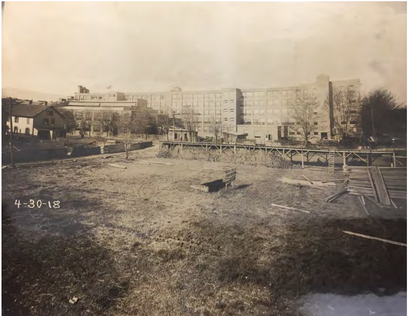
04-30-1918 Construction Photo of Lycoming Rubber Company; view from lot across Rose Street looking southwest; Lockwood Greene Records, Archives Center, National Museum of American History, Smithsonian Institution
