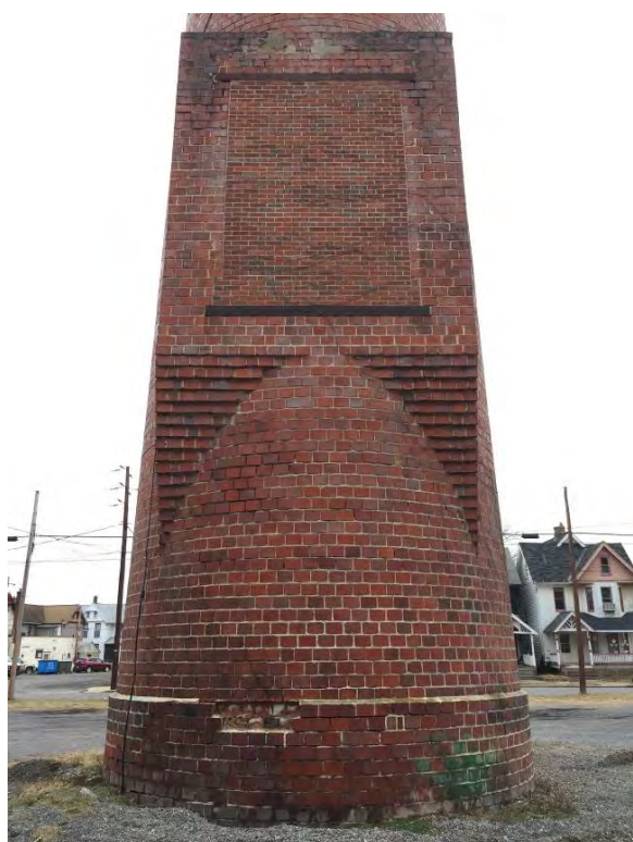
Photo 86. View of the throat of the boiler house chimney looking west toward Cemetery Street.
