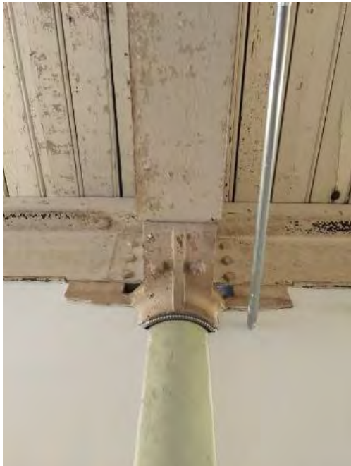
Photo 46. Column capital on second floor at corridor partition. Note exposed metallic wire just below capital.
