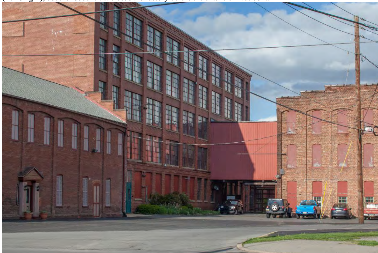
Photo 71. View of the South elevation of the 5-story Building C from the parking lot of the original 2-story Building C.
