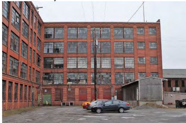
Photo 74. West end of north elevation of New Building C. The single-story concrete block loading dock covered in wood siding was constructed after the rail line and power plant were demolished.
