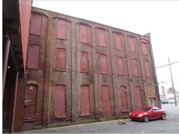
Photos 5. & 6. North elevation east and west of the 2-story bridge connecting Building A to Building C. The east end of the north elevation abuts the 1918 Building A extension, visible at the far right of Photo 5. An original doorway at the ground level of the engine room at the west end of the north elevation has been partially filled in with brick to accommodate a standard size metal door with a vision panel, and the ground floor window in the 4 th bay from the west end has been enlarged to provide an entrance door that is now covered with plywood.
