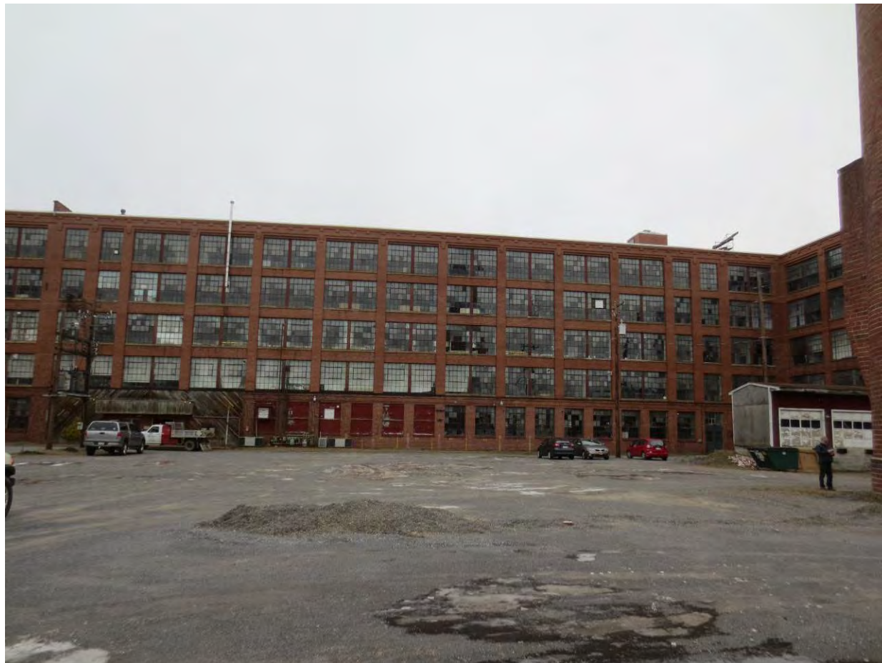
Photo 37. West elevation of Building H. The firewall visible above the roofline at the north end and the elevator tower and hoist visible above the roof line at the south end mark the limits of the building constructed in 1917.
