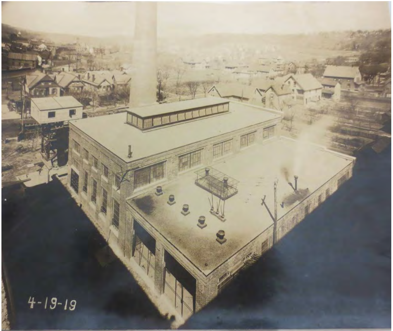
04-19-1919 Construction Photo of Building M, New Boiler House and Chimney; Lycoming Rubber Company; looking northwest; Lockwood Greene Records, Archives Center, National Museum of American History, Smithsonian Institution
