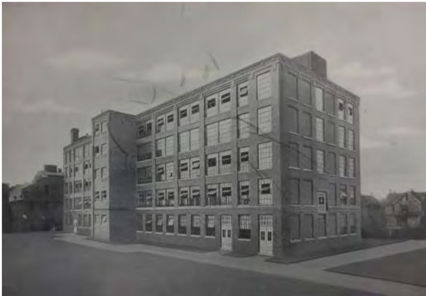
Undated construction photo of the east façade of Building H taken from the empty lot at the corner of Park Avenue and Rose Street before the bridge linking Building H to Building K was constructed. The original 4-story vulcanizer building constructed in 1882 is visible in the background at left. The clouds in the background and parking area in the foreground of the image were added by an artist. Construction images from Lockwood Greene Records, Archives Center, National Museum of American History, Smithsonian Institution
