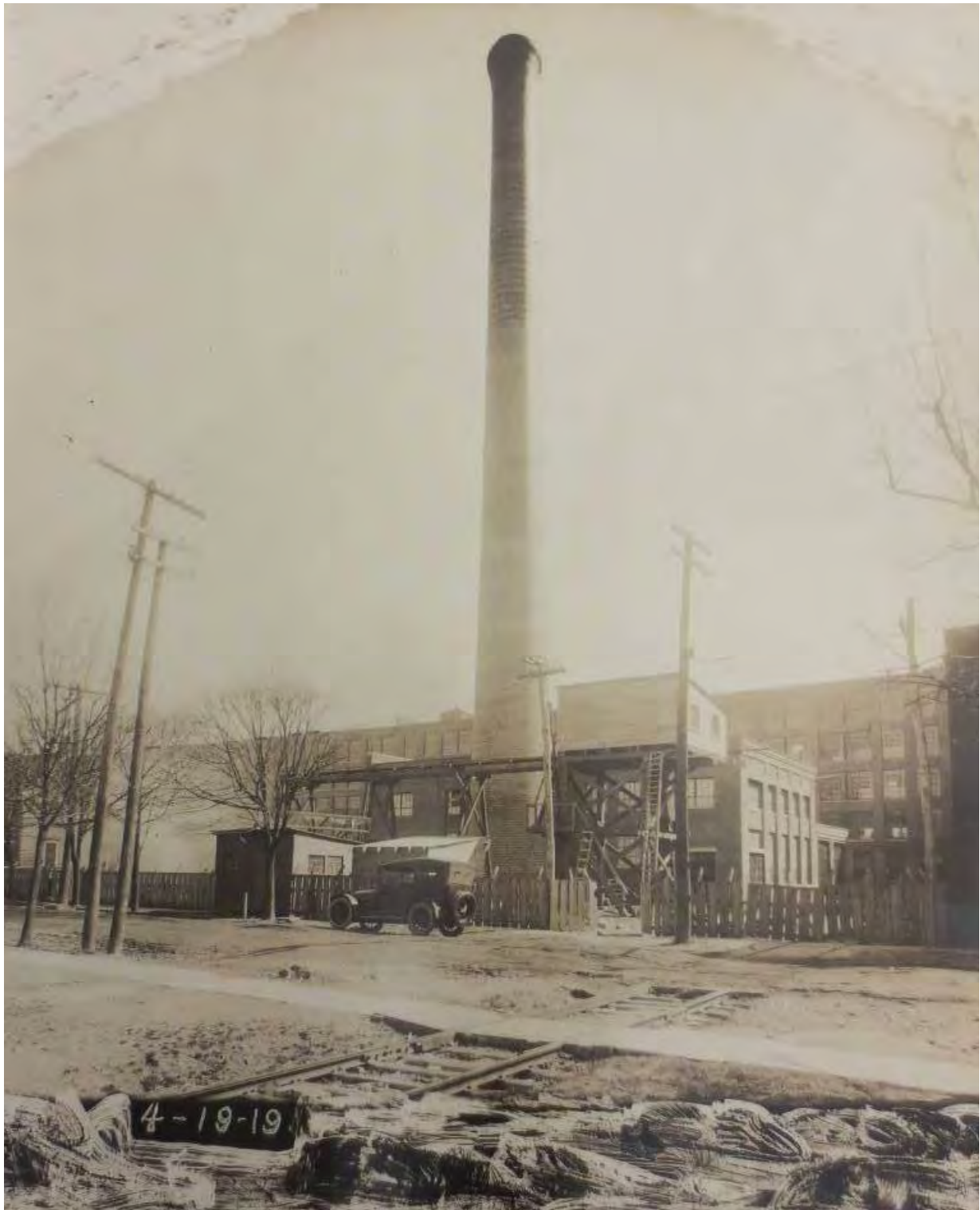
04-19-1919 Construction Photo of Building M, New Boiler House and Chimney; Lycoming Rubber Company; Lockwood Greene Records, Archives Center, National Museum of American History, Smithsonian Institution
