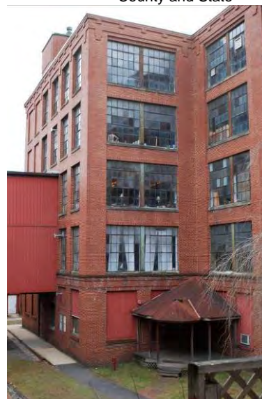
Photo 72. West elevation of Building E and Old Building C in the foreground, with 5-story New Building C behind. Note the brick infill in the masonry openings for the proposed extension to Cemetery Street.
