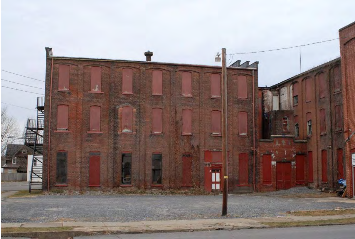
Photo 31. East (Rose Street) elevation of Building F, with ground floor infirmary at right.
