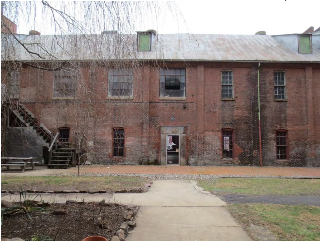
Photo 25. View of Courtyard Elevation of Building D extension
