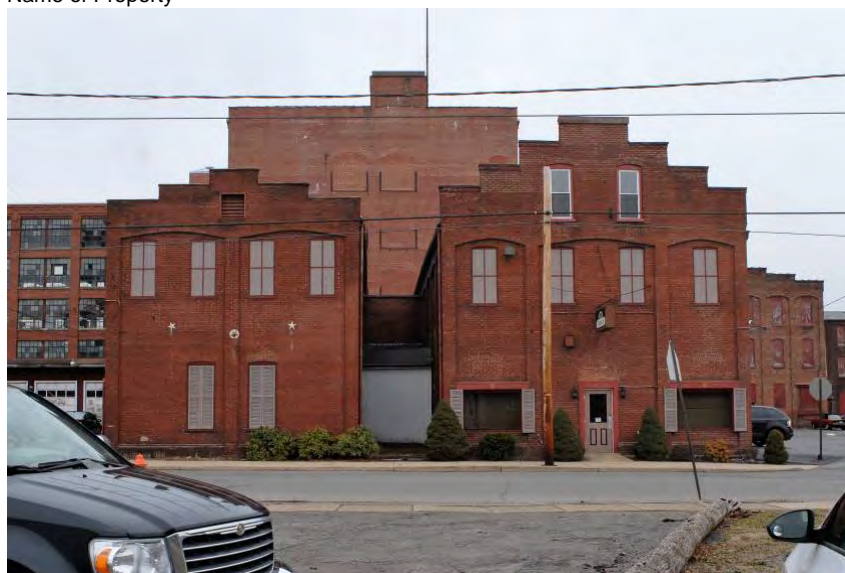
Photo 72. West elevation of Building E and Old Building C in the foreground, with 5-story New Building C behind. Note the brick infill in the masonry openings for the proposed extension to Cemetery Street.
