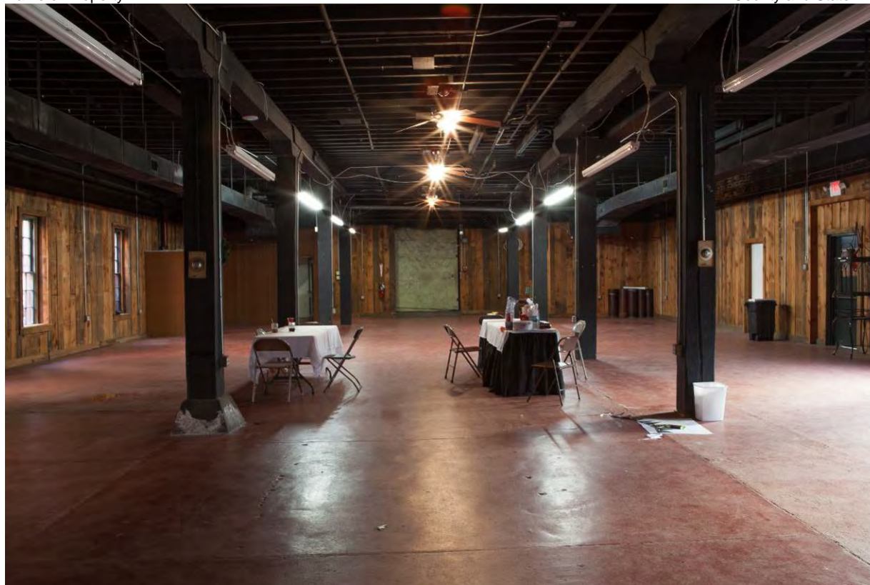
Photo 28. View of ground floor looking north. The volume, exposed structure and windows are all original.
