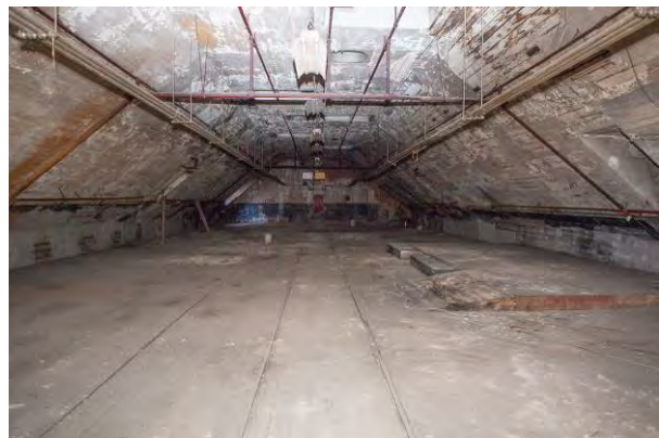
Photo 27. View of attic floor looking north.
