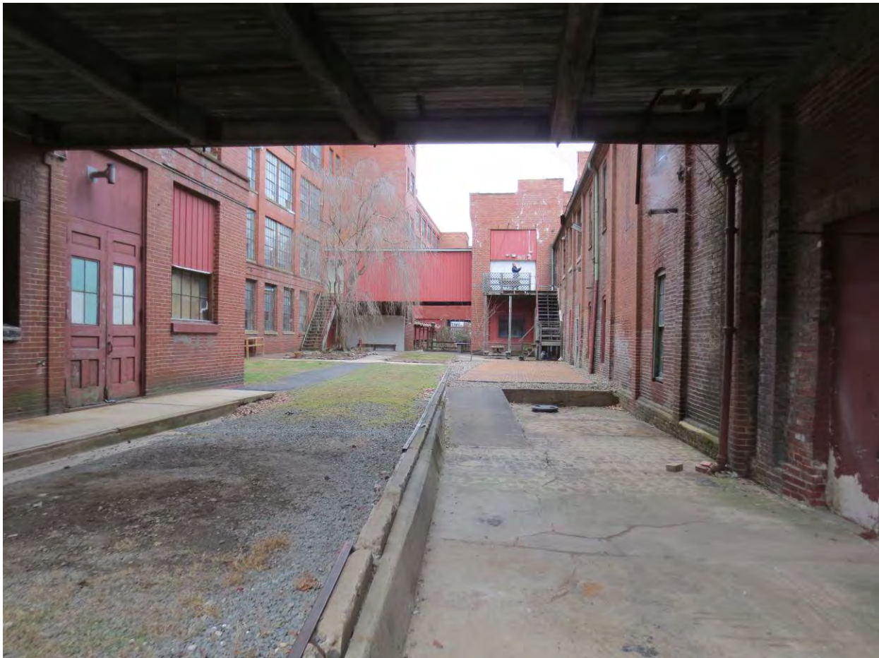
Photo 19. View of courtyard looking north from beneath the 2-story bridge between Building D and Building C.
