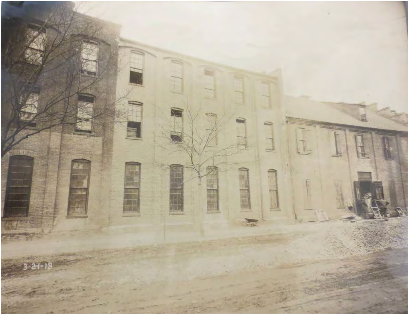
03-21-1918 Construction Photo of Building A extension (center), on Rose Street between Building A (left), and Building D (right); Lycoming Rubber Company; Lockwood Greene Records, Archives Center, National Museum of American History, Smithsonian Institution
