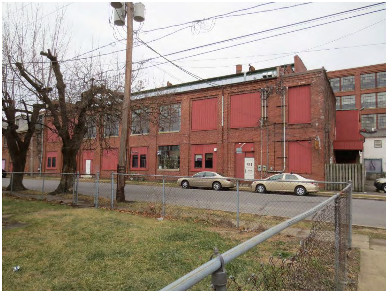
Photo 50. Rose Street elevation of Building K
