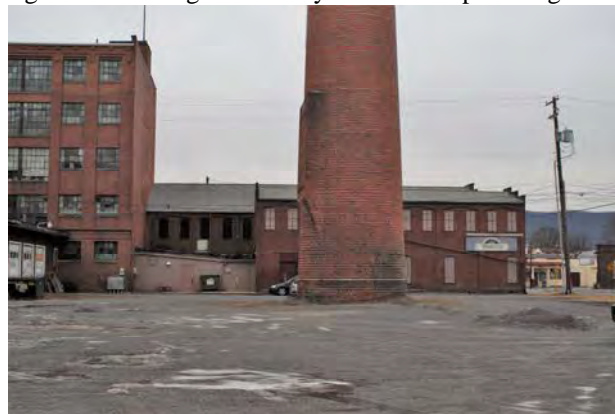
Photo 74. West end of north elevation of New Building C. The single-story concrete block loading dock covered in wood siding was constructed after the rail line and power plant were demolished.
