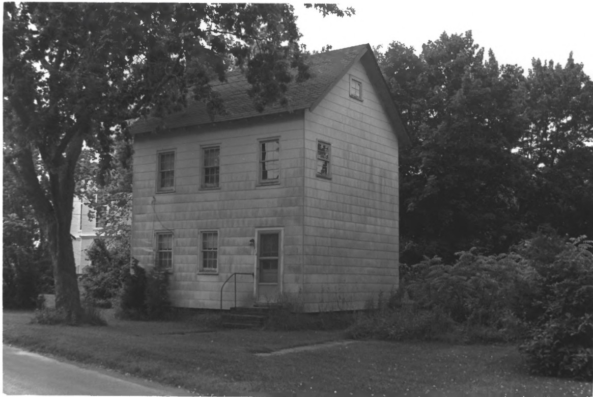
114 Main Street, Port Republic Historic District, Atlantic County, N.J. #10 of 40
