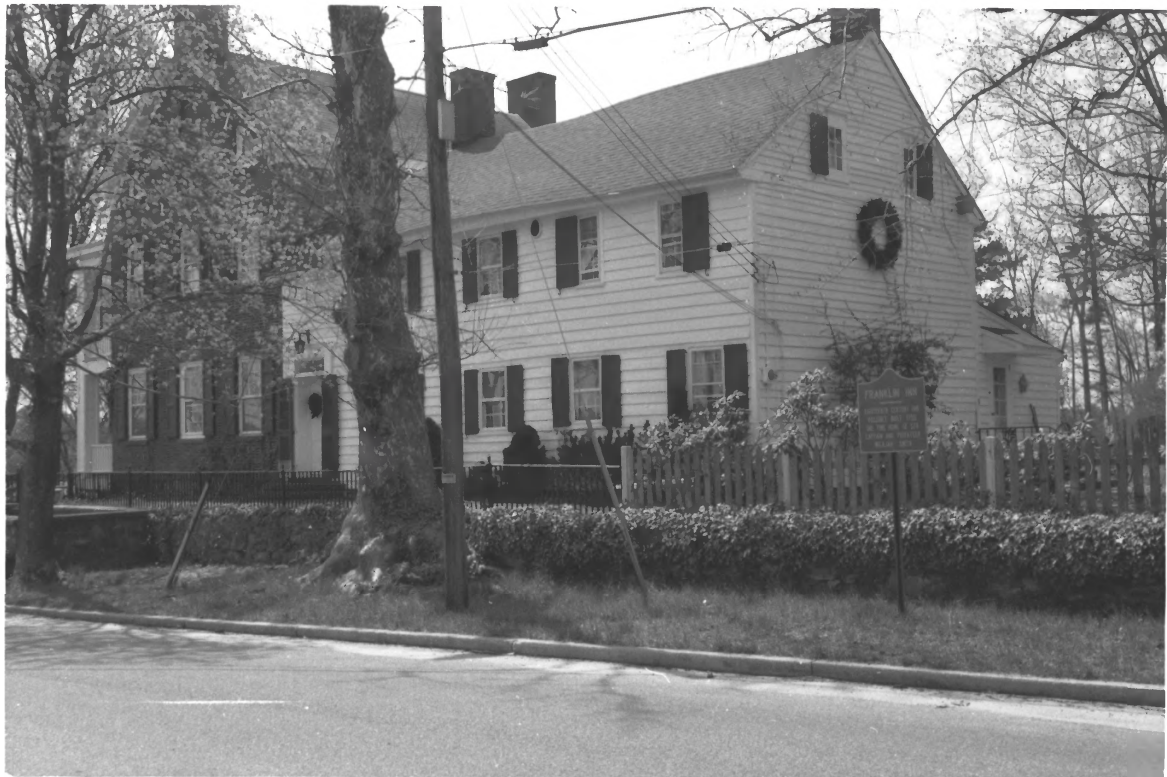
5 Mill Street, Franklin Inn, Port Republic Historic District, Atlantic County, N.J. # 2 of 40
