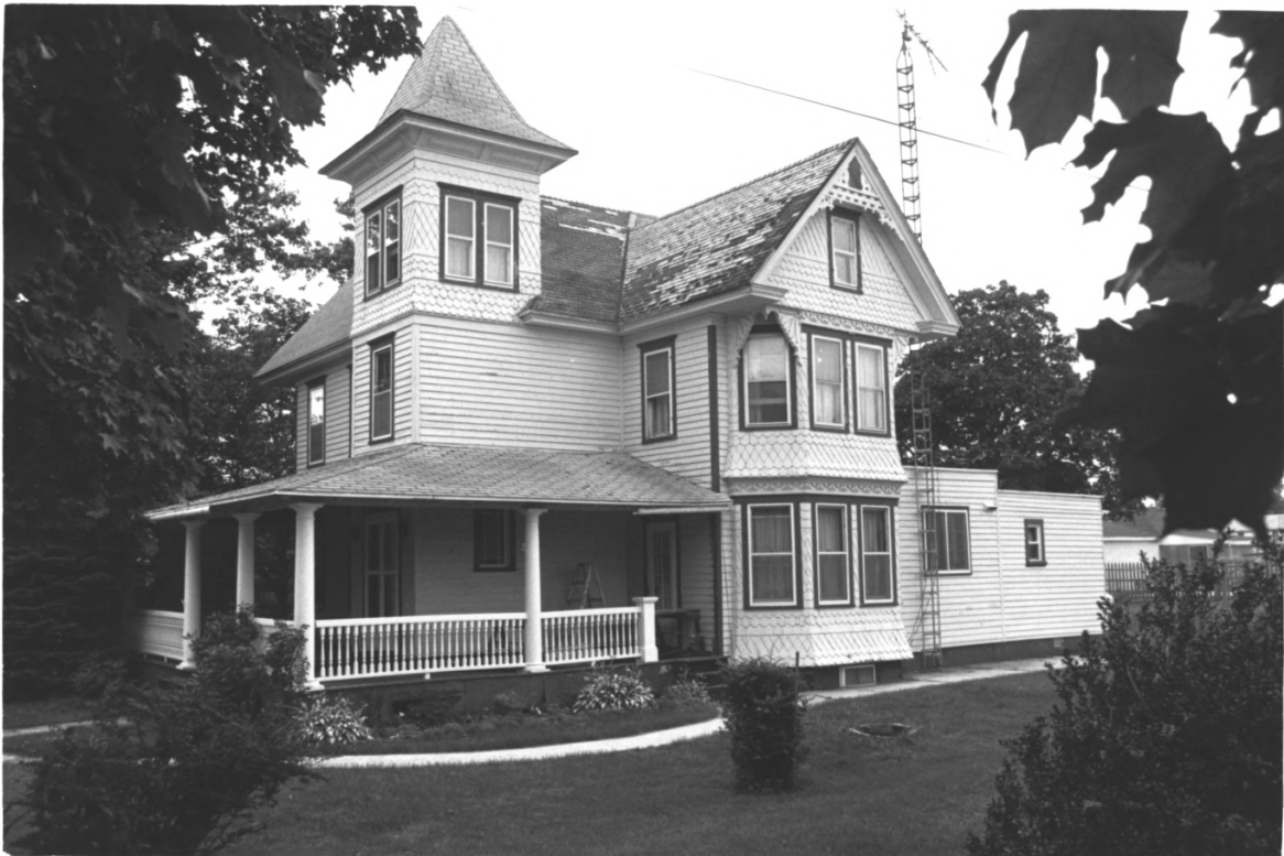
26 Main Street, Port Republic Historic District, Atlantic County, N.J. #29 of 40
