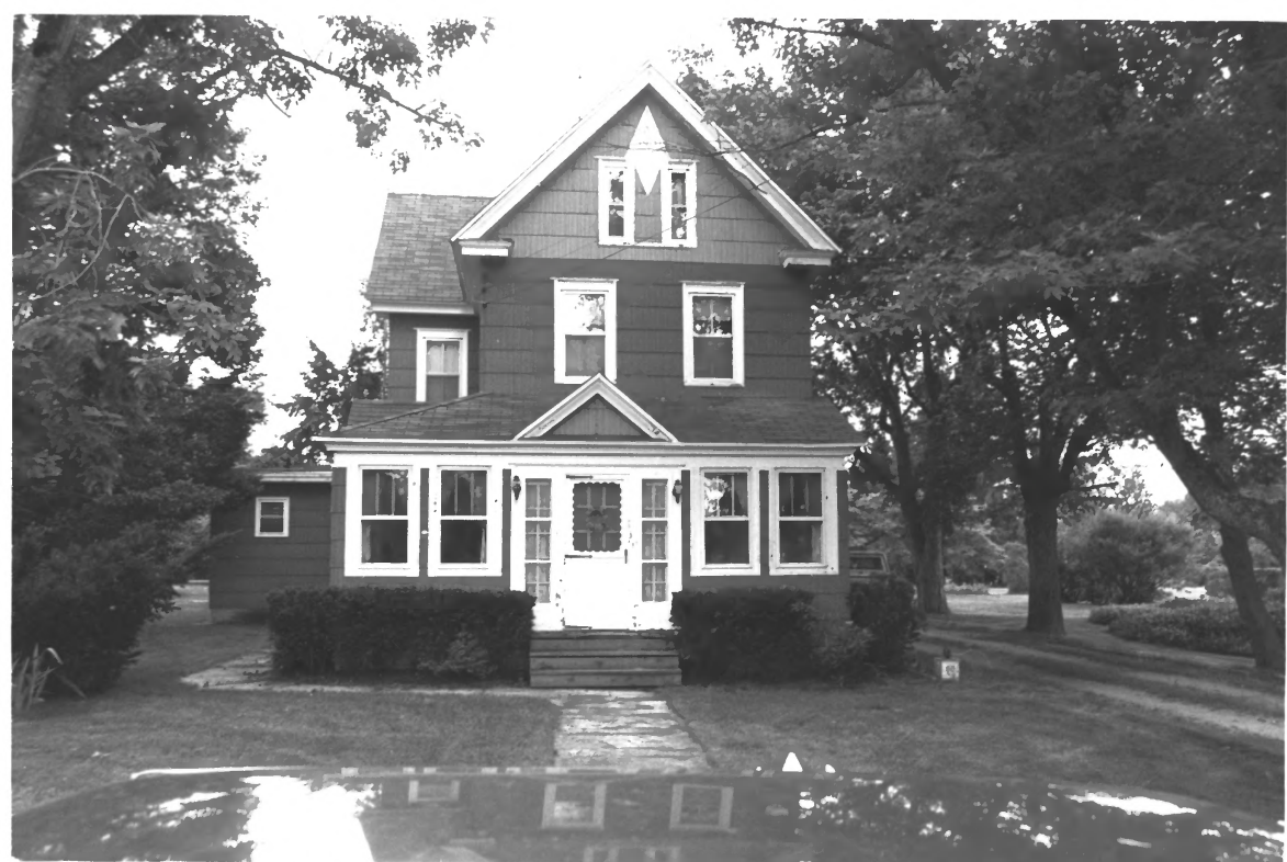
23 Main Street, Port Republic Historic District, Atlantic County, N.J. #34 of 40
