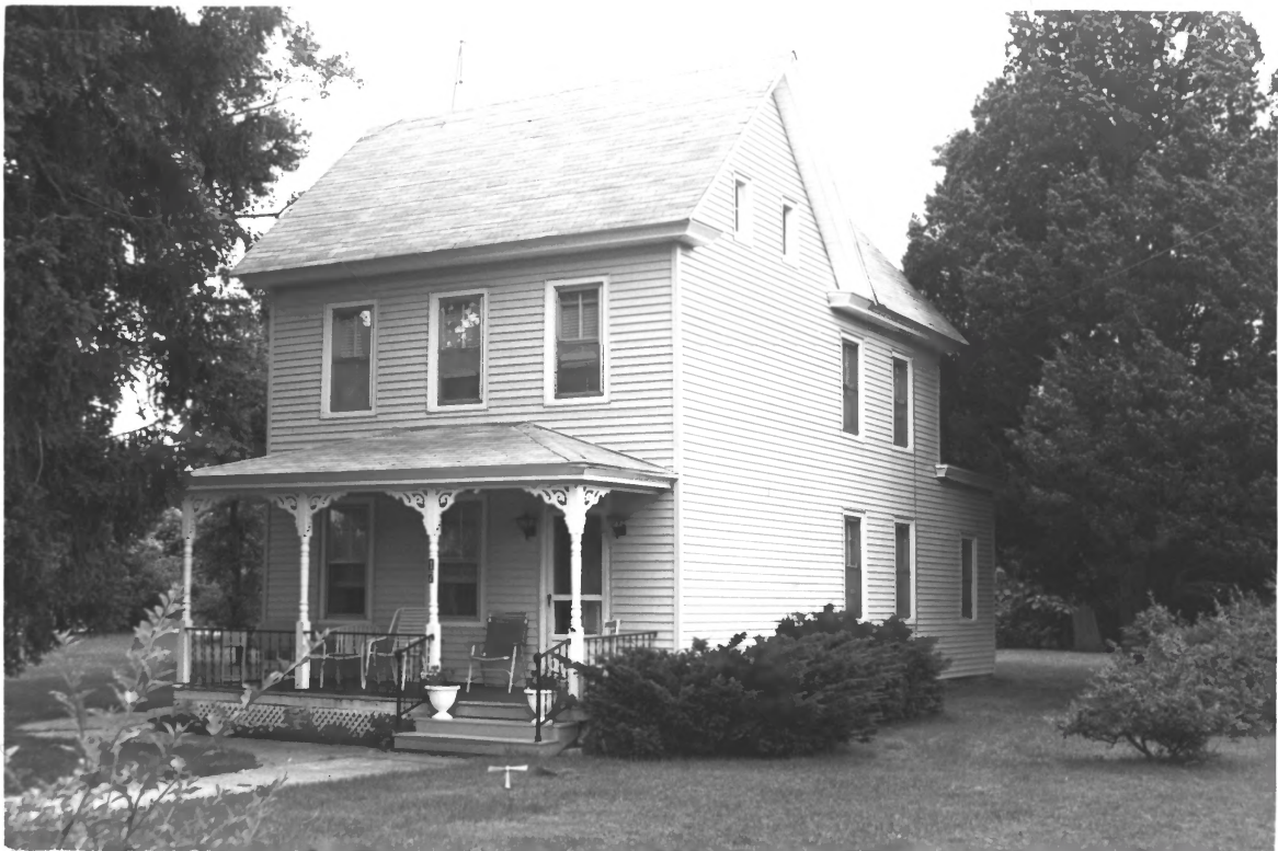
17 Main Street, Port Republic Historic District, Atlantic County, N. J. # 18 of 40
