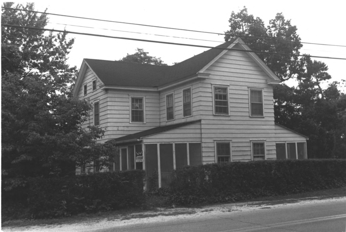
109 Main Street, Port Republic Historic District, Atlantic County, N.J. #12 of 40
