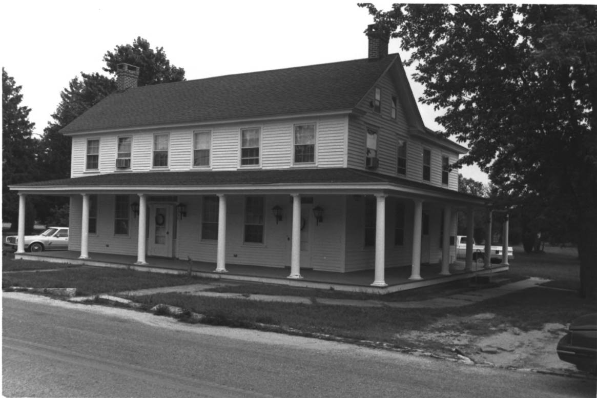
39 Main Street, Port Republic historic District, Atlantic County, N.J. #30 of 40
