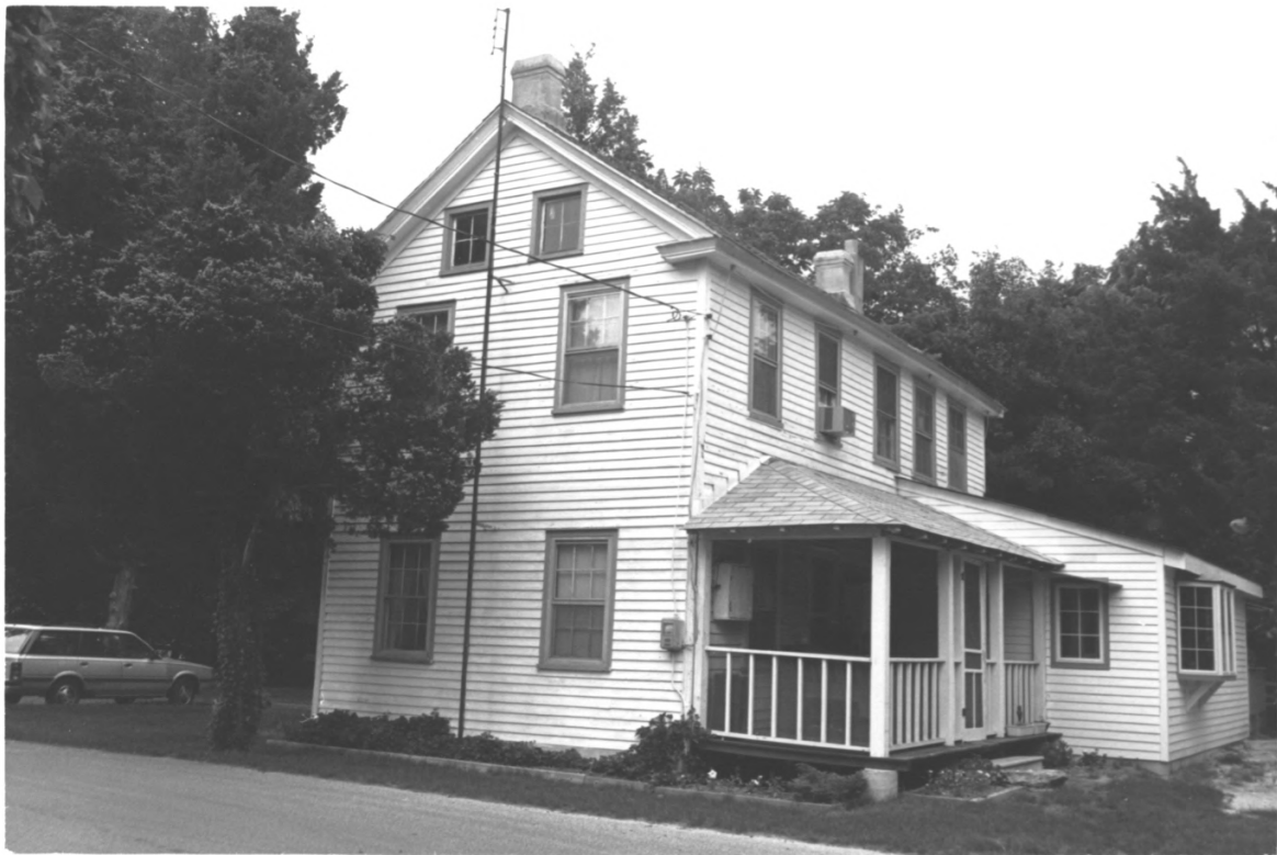
138 Central Ave., Port Republic Historic District, Atlantic County, N.J. #26 of 40
