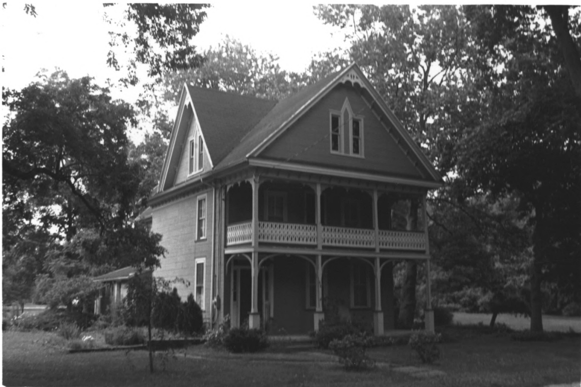
56 Main Street, Port Republic Historic District, Atlantic County, N.J. #15 of 40
