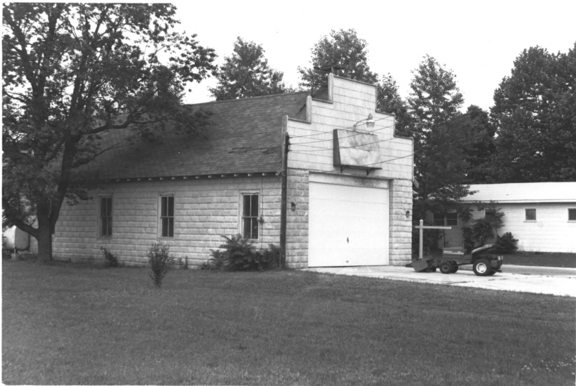
Old Firehouse on Pomona Ave, Port Republic Historic District, Atlantic Co., N.J. #40 of 40
