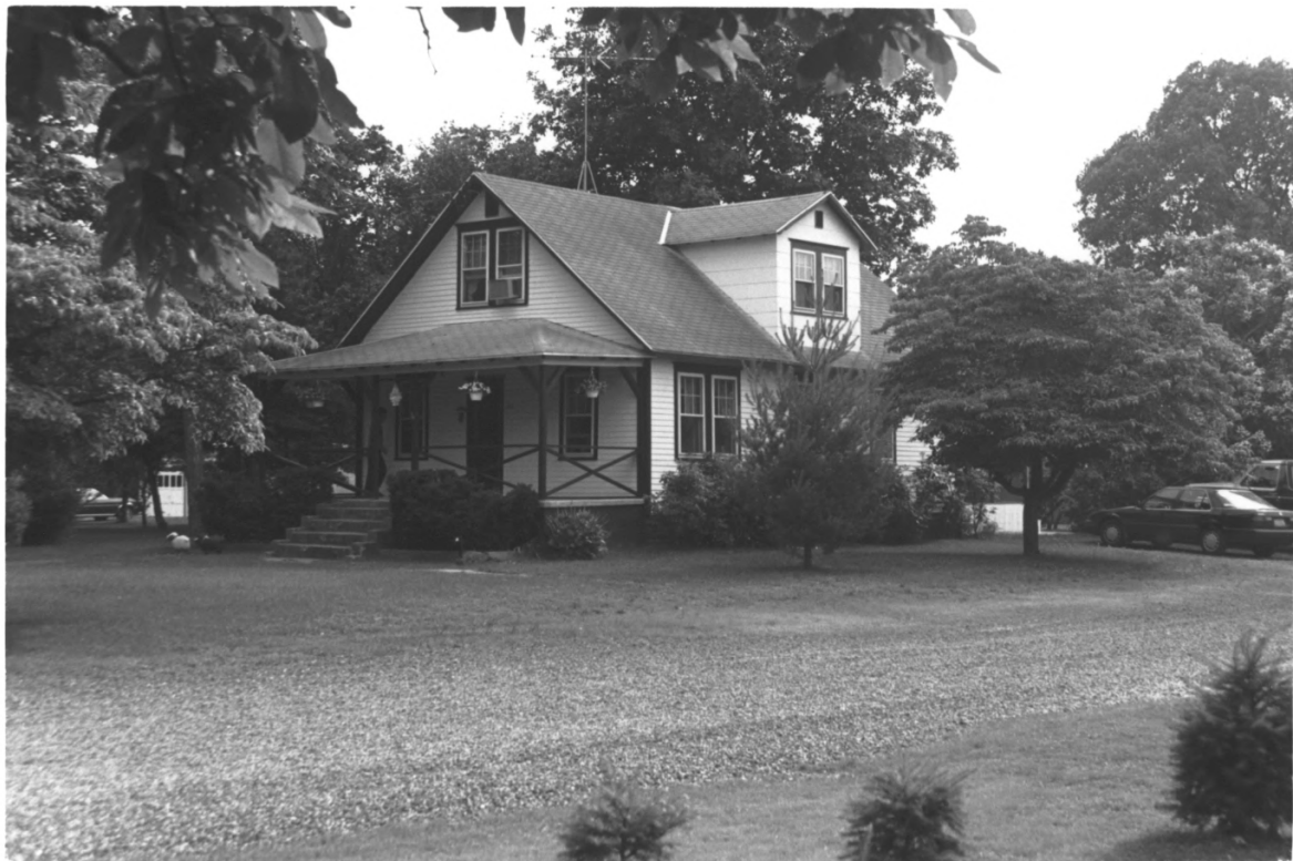
133 Central Ave., Port Republic Historic District, Atlantic County, N.J. #27 of 40
