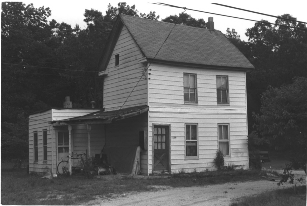
178 Mill Street, Port Republic Historic District, Atlantic County, N.J. # 24 of 40
