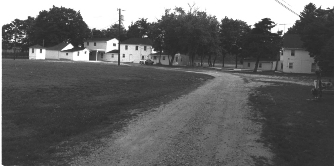
39-41 Main Street, Port Republic Historic District, Atlantic County, N. J. # 19 of 40
