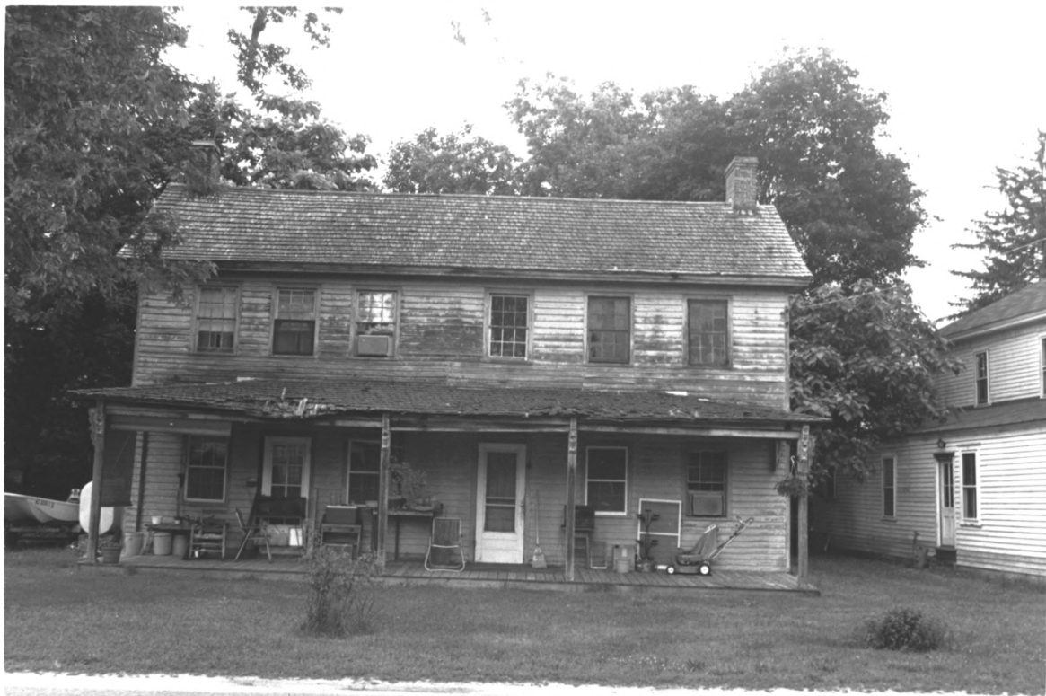
109 Main Street, Port Republic Historic District, Atlantic County, N.J. #13 of 40
