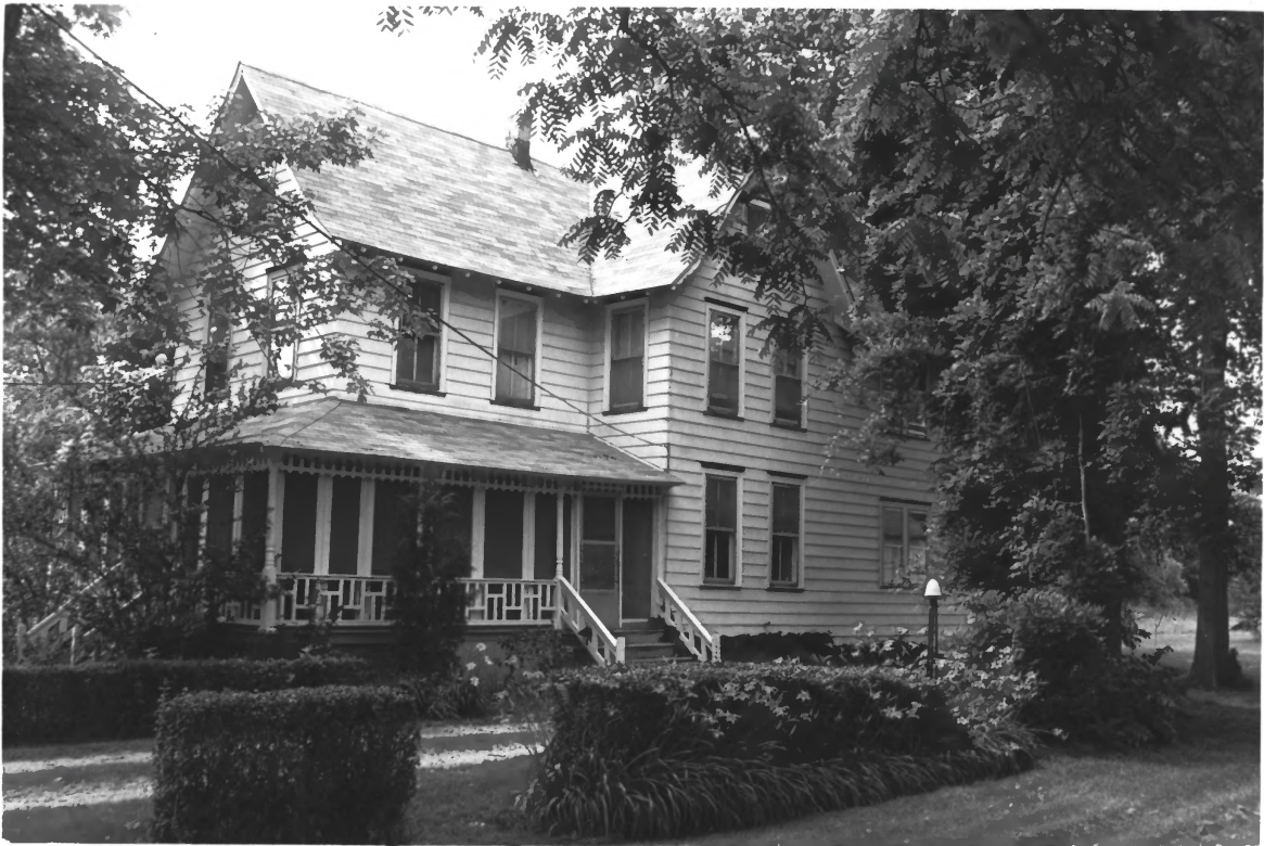
114 Main Street, Port Republic Historic District, Atlantic County, N. J # 11 of 40
