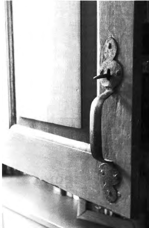
Photo 21. Enos Kellogg House, Norwalk, Fairfield County, Connecticut. Front door latch. July 29, 2011, Tod Bryant
