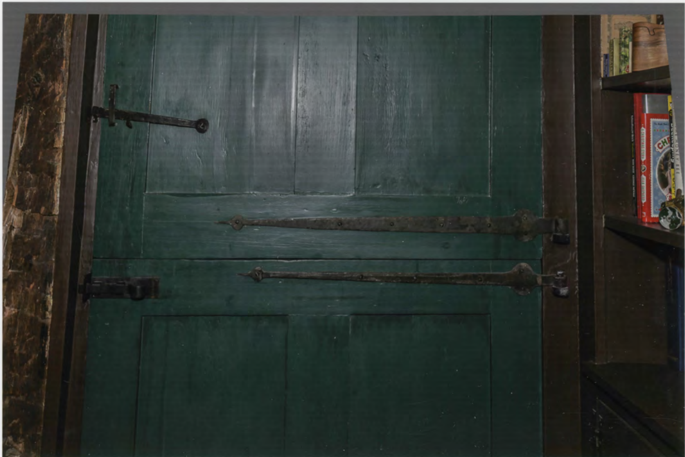
Photo 4. Enos Kellog House, Norwalk, Fairfield County, Connecticut. First floor interior, view west, showing original front door hardware. July 29, 2011, Tod Bryant.
