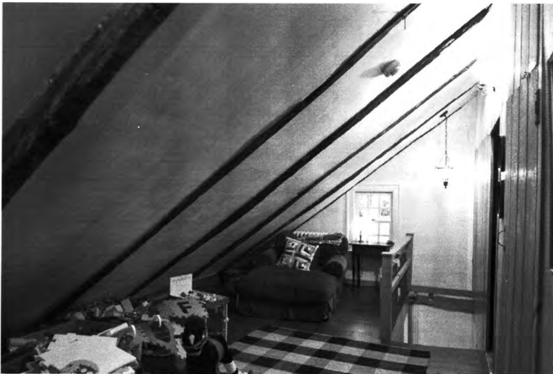
Photo 16. Enos Kellog House, Norwalk, Fairfield County, Connecticut. Second floor, view south showing saltbox ceiling slant. July 29, 2011, Tod Bryant
