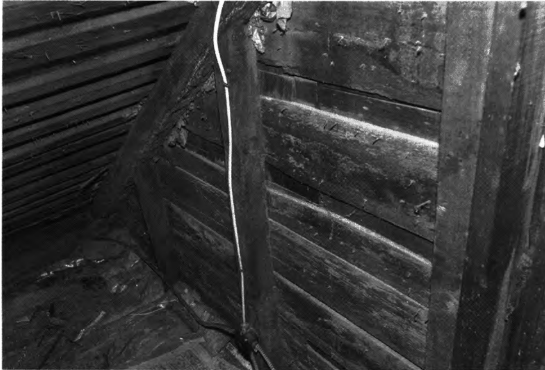
Photo 5. Enos Kellog House, Norwalk, Fairfield County, Connecticut. Attic showing original siding used as sheathing. July 29, 2011, Tod Bryant
