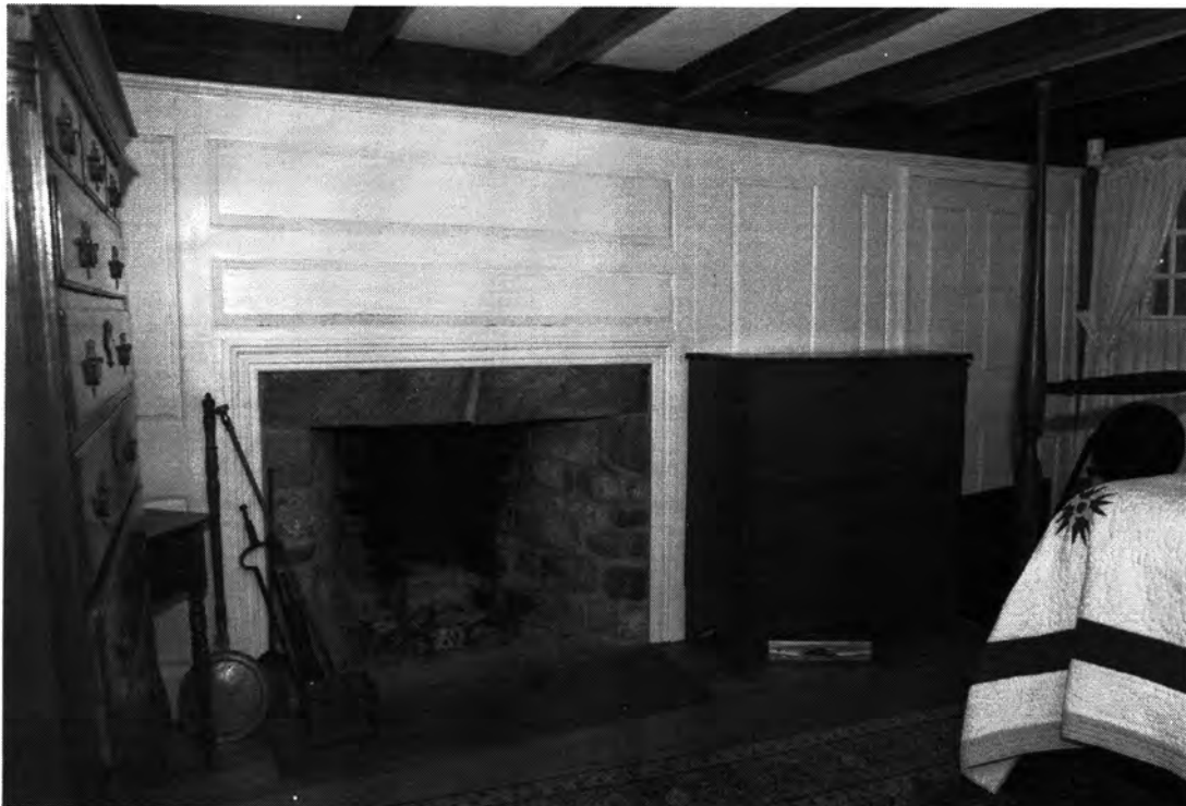
Photo 8. Enos Kellogg House, Norwalk, Fairfield County, Connecticut. First floor North Rom, view southeast showing paneling, framing and fireplace. July 29, 2011, Tod Bryant
