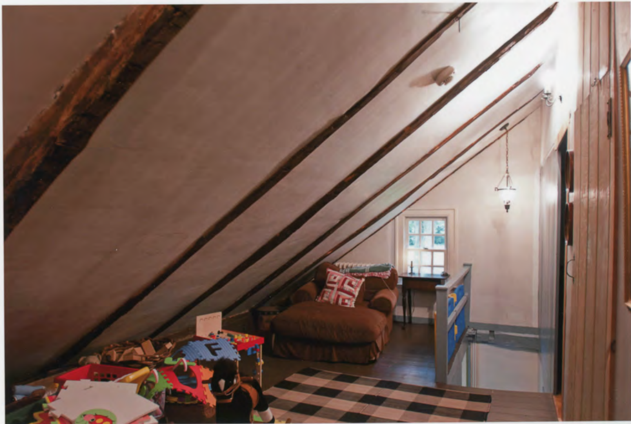
Photo 16. Enos Kellogg House, Norwalk, Fairfield County, Connecticut. Second floor, view south showing saltbox ceiling slant. July 29, 2011, Tod Bryant
