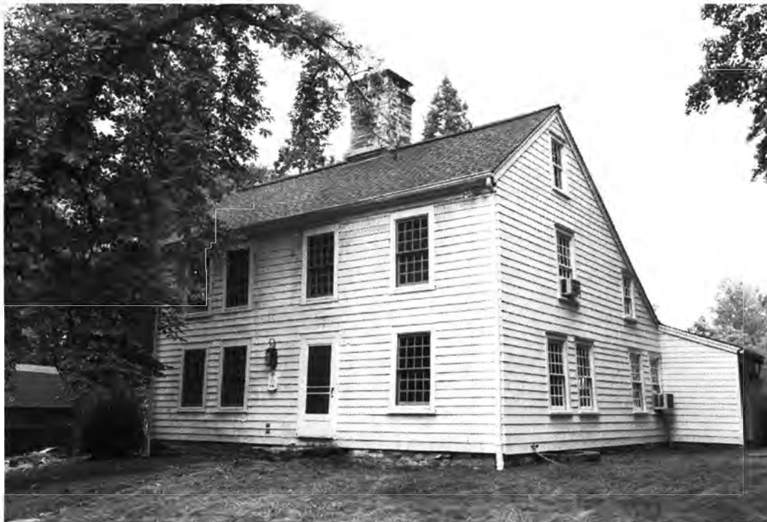
Photo 1. Enos Kellogg House, Norwalk, Fairfield County, Connecticut. View north, July 28, 2011, Tod Bryant
