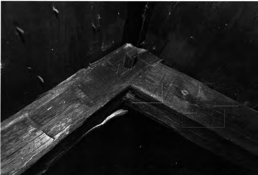
Photo 6. Enos Kellog House, Norwalk, Fairfield County, Connecticut. Attic showing rafter framing detail and raising marks. July 29, 2011, Tod Bryant
