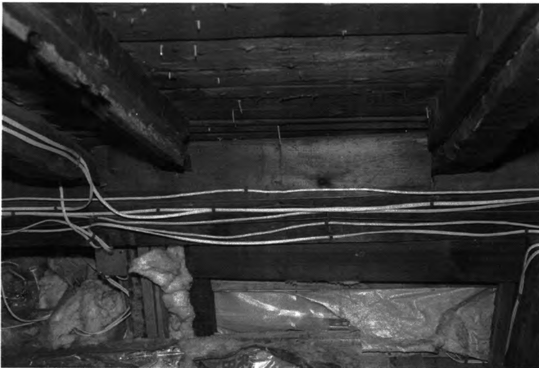
Photo 20. Enos Kellogg House, Norwalk, Fairfield County, Connecticut. Attic, view east showing raised plate framing detail. July 29, 2011, Tod Bryant
