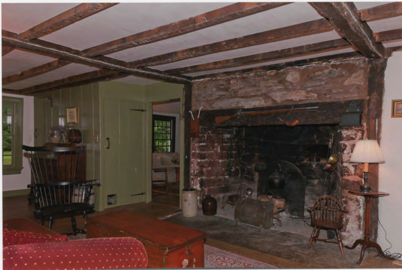
Photo 11. Enos Kellogg House, Norwalk, Fairfield County, Connecticut. First floor interior view southwest showing fireplace and framing. July 29, 2011, Tod Bryant
