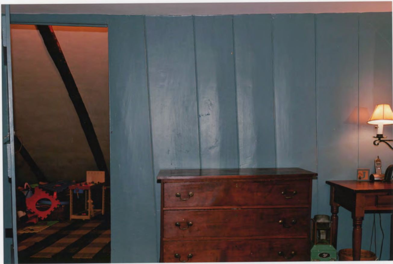
Photo 17. Enos Kellog House, Norwalk, Fiarfield County, Connecticut. Second floor South Chamber, view east, showing slanted paneling. July 29, 2011, Tod Bryant.
