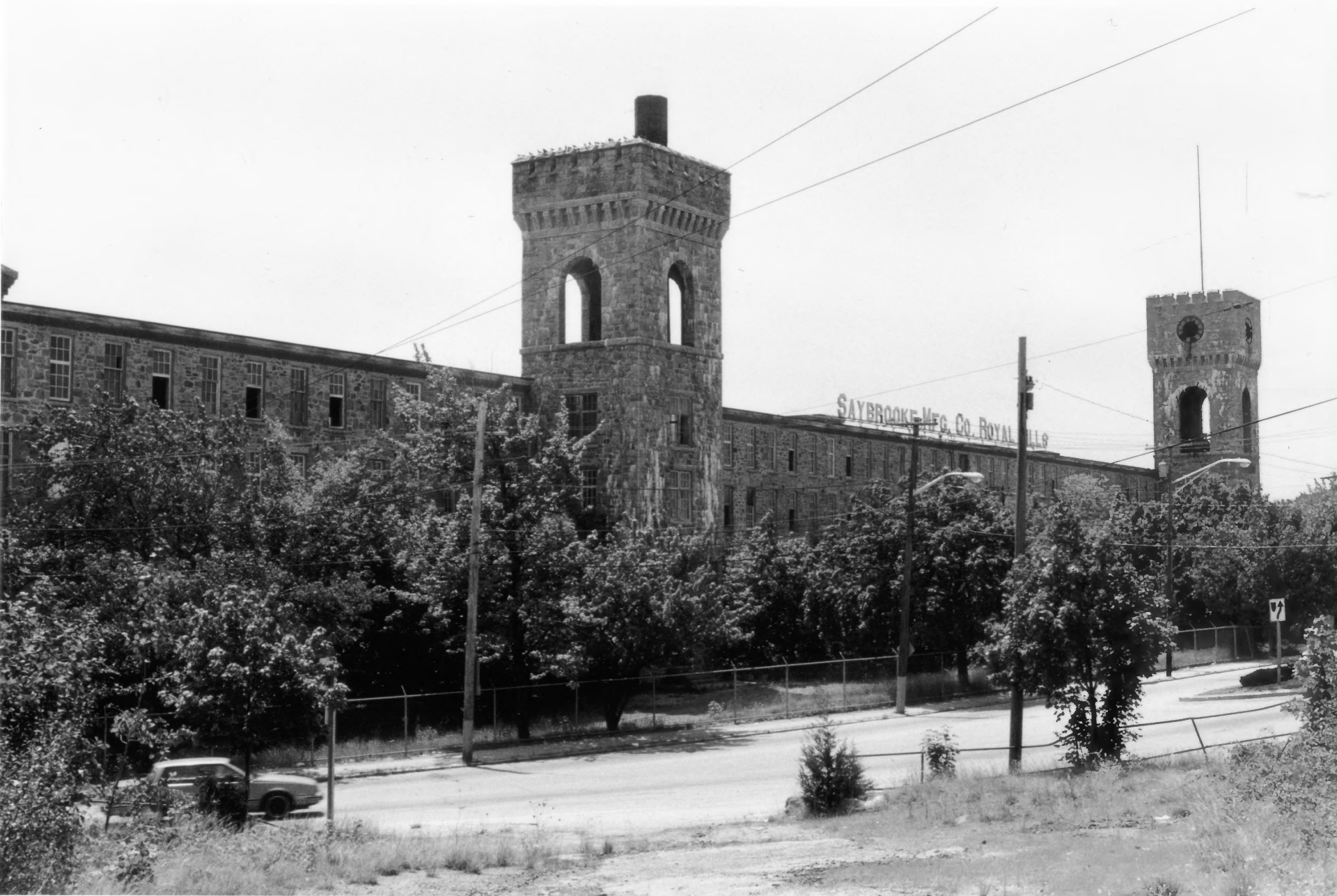
ROYAL MILL COMPLEX KENT COUNTY, RI No. 1
