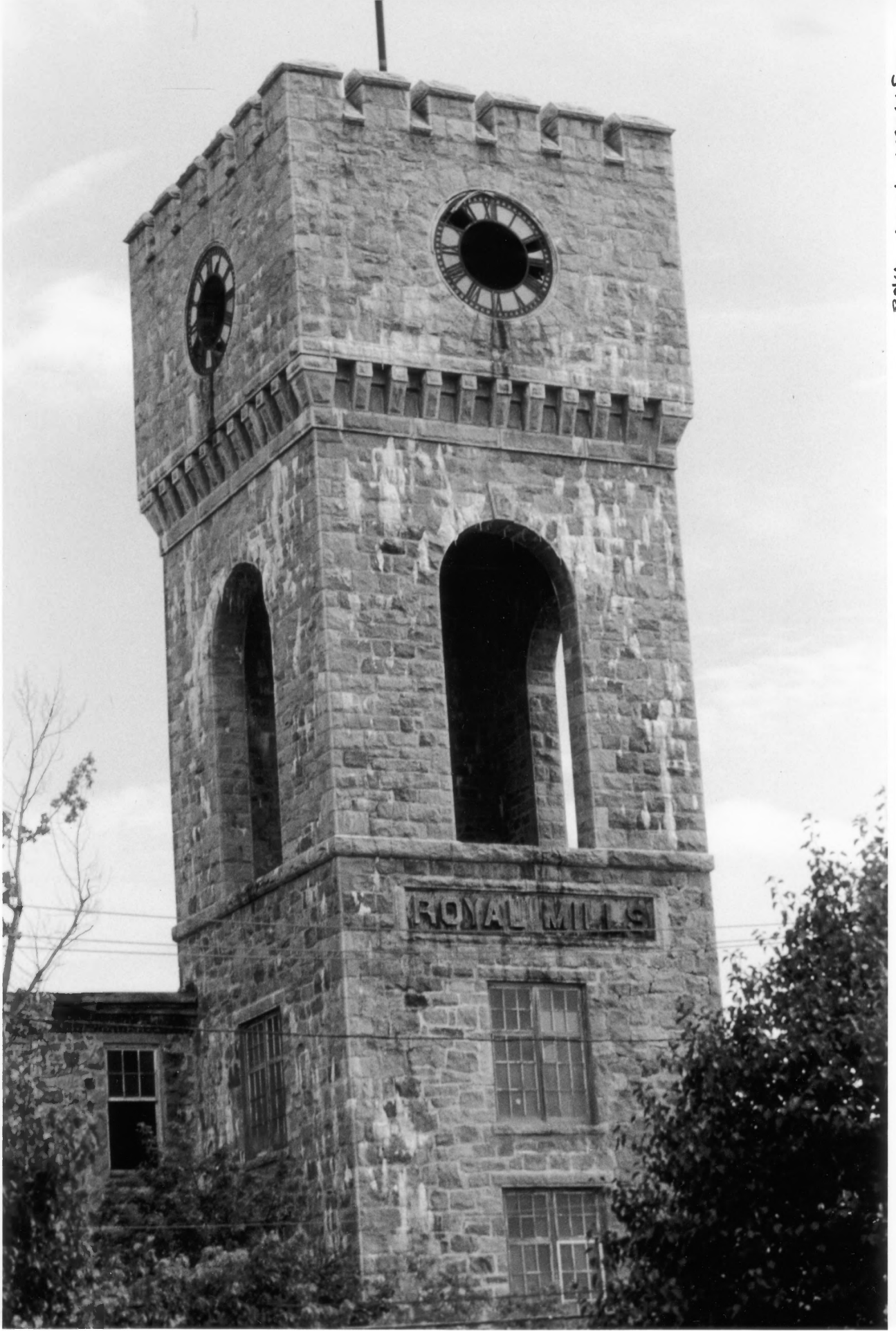
ROYAL MILL COMPLEX KENT COUNTY, RI No. 2
