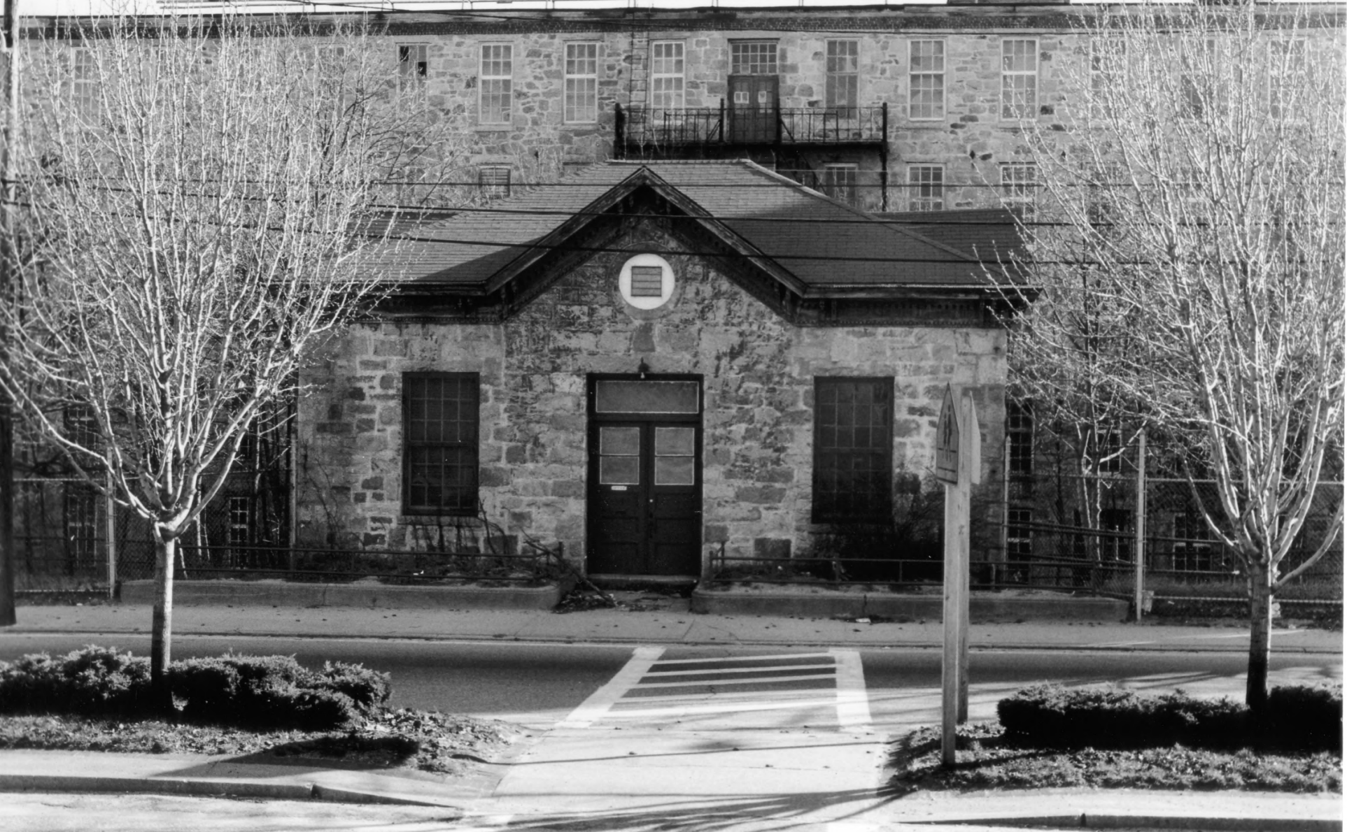
ROYAL MILL COMPLEX KENT COUNTY, RI No. 6
