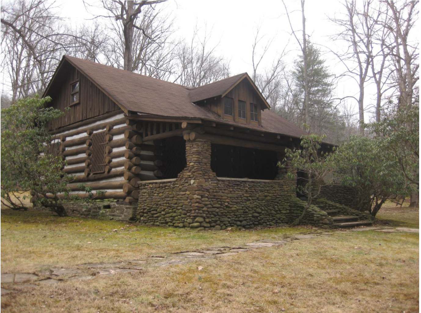
Photo 8 of 11: Cabin No. 7, camera facing southeast
