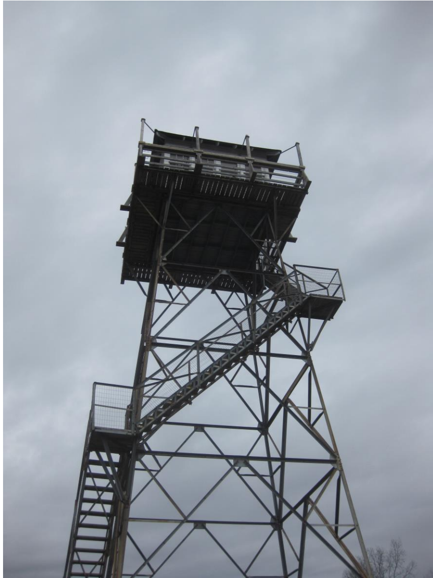
Photo 3 of 11: Brushy Mountain Fire Tower, camera facing up
