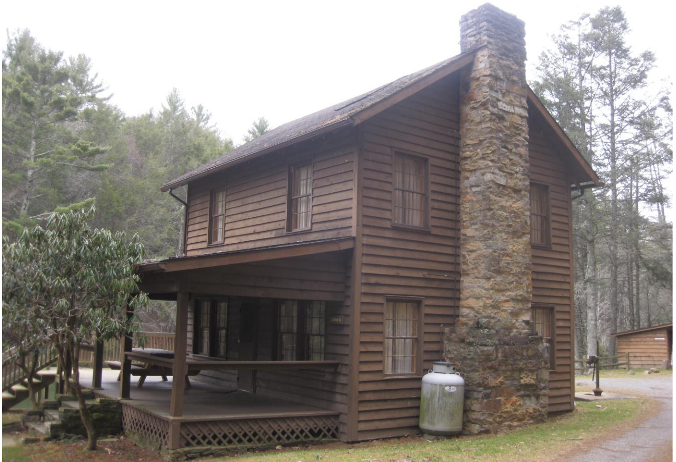
Photo 10 of 11: Cabin No. 4, camera facing northeast
