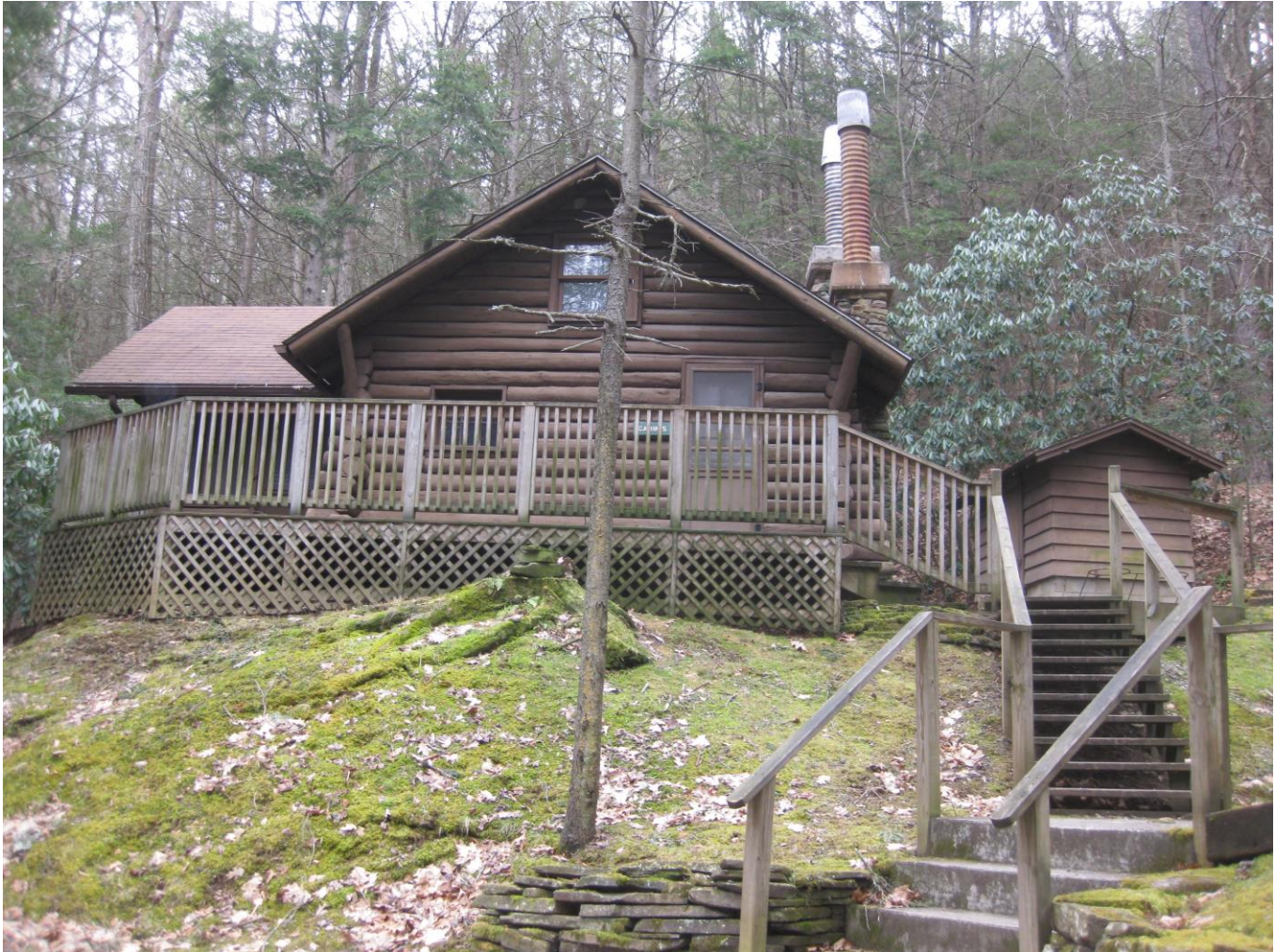
Photo 9 of 11: Cabin No. 5, camera facing south
