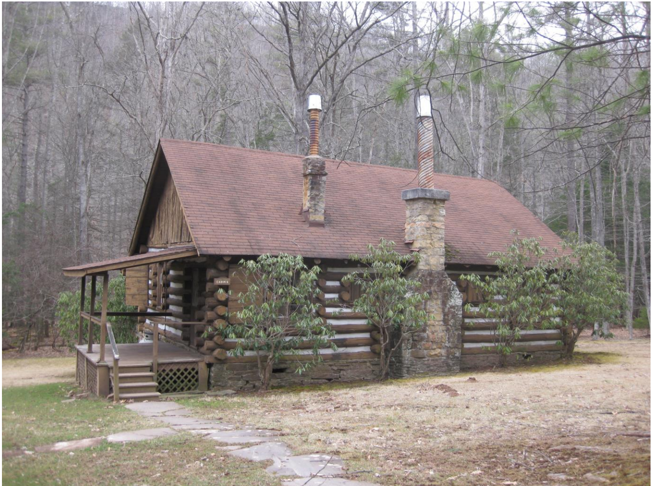
Photo 7 of 11: Cabin No. 6, camera facing west
