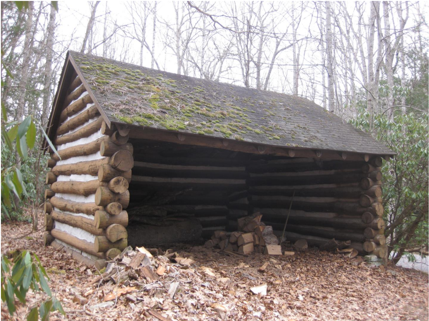
Photo 6 of 11: Wood Depot/CCC Garage, camera facing east
