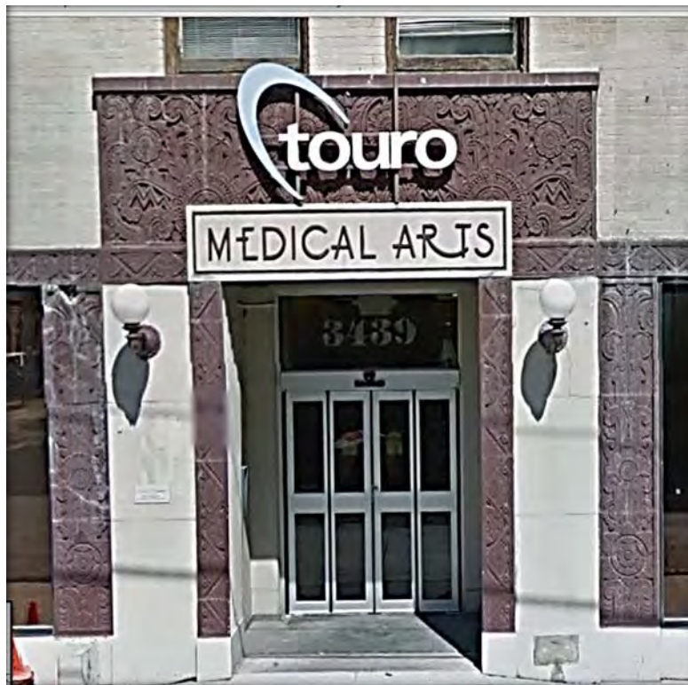
Figure 16. 3435 Prytania St., Nola. Medical Arts Building. Richard Koch, architect (1949). Image courtesy of www.google.com/maps .
