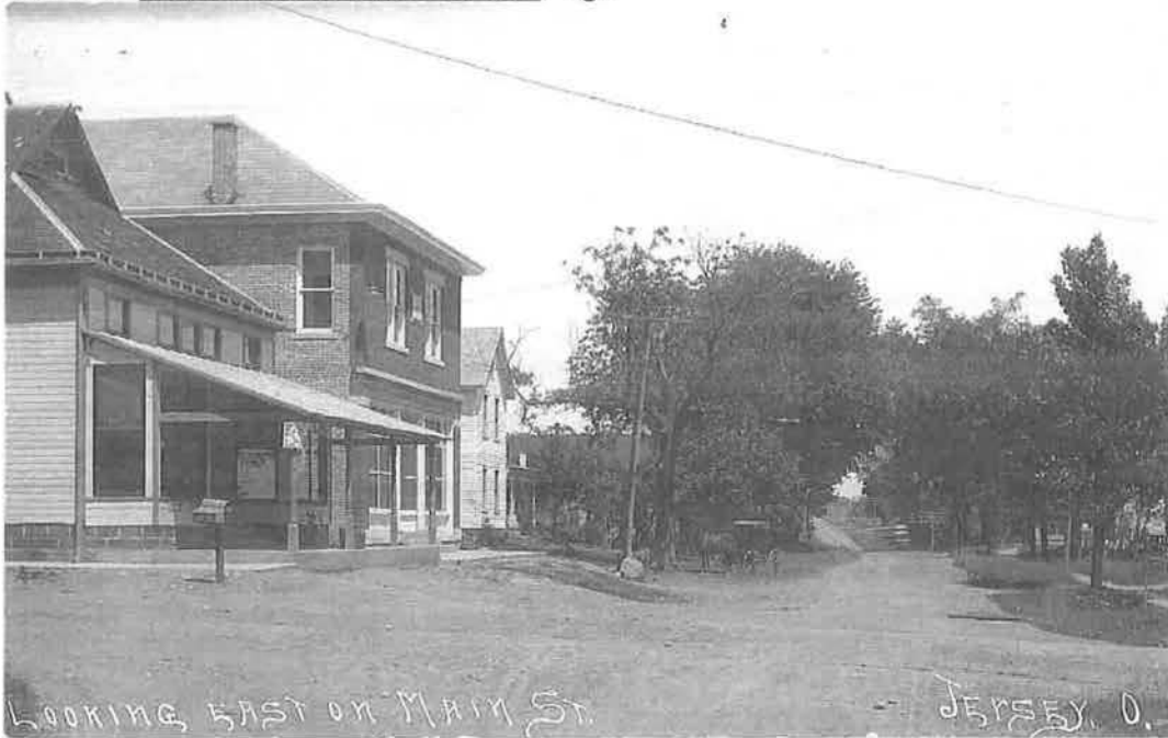
Figure 9. Another view, looking east, of the rebuilt IOOF building, second from left.
