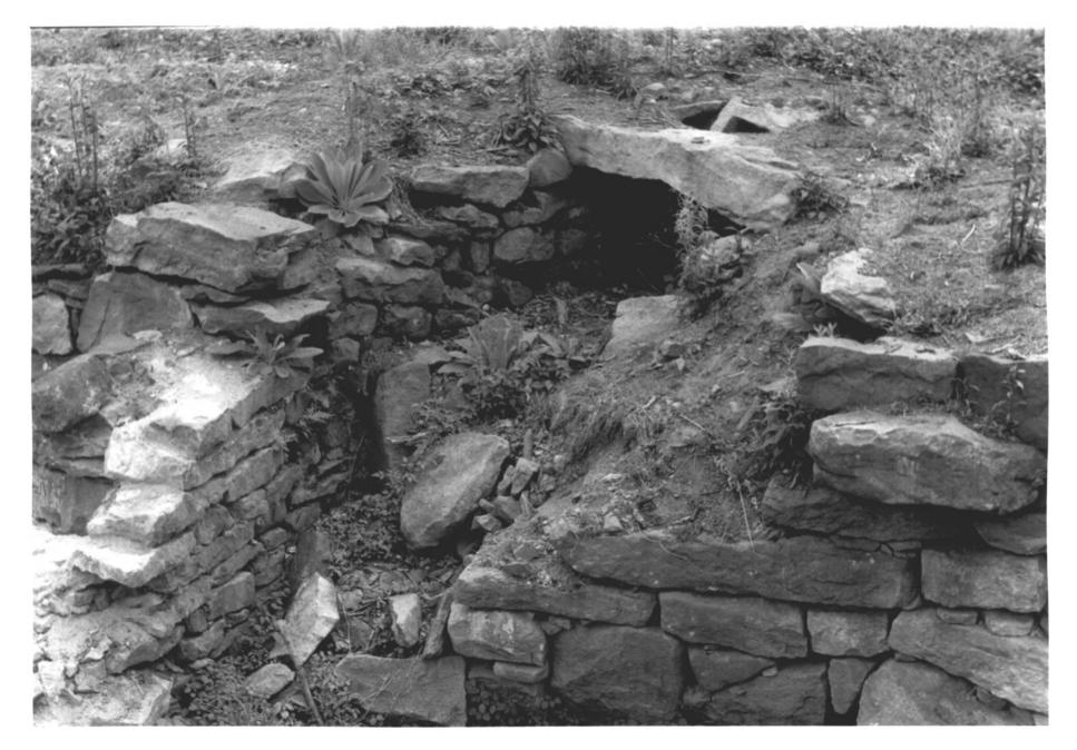
Photograph No. 3 Intersection of underground channel and FARMINGTON CANAL LOCK NO. 13 Hamden, Connecticut Michael S. Raber June 23, 1981 Negative: Connecticut Historical Commission stone headers which separated the masonry lock walls from the original wooden lock chamber is at right center.
