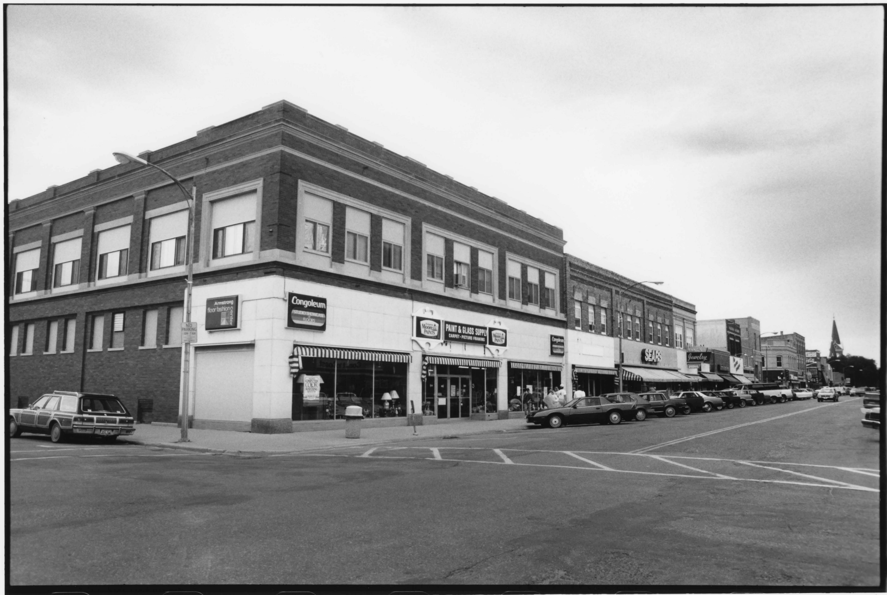
F.W. MANN CO. BUILDING RAMSEY CO. NORTH DAKOTA PHOTO 11
