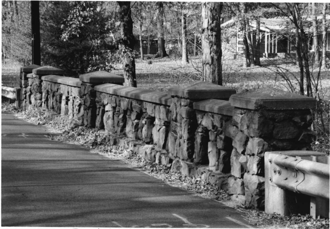
034 023 Randolphville Bridge (3 of 7)
