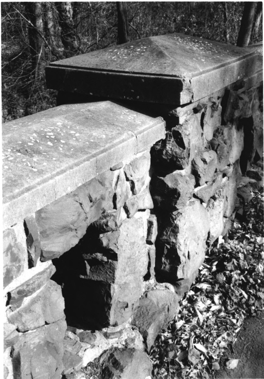
034 023 Randolphville Bridge (7 of 7)
