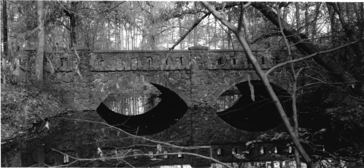
034 023 Randolphville Bridge (5 of 7)
