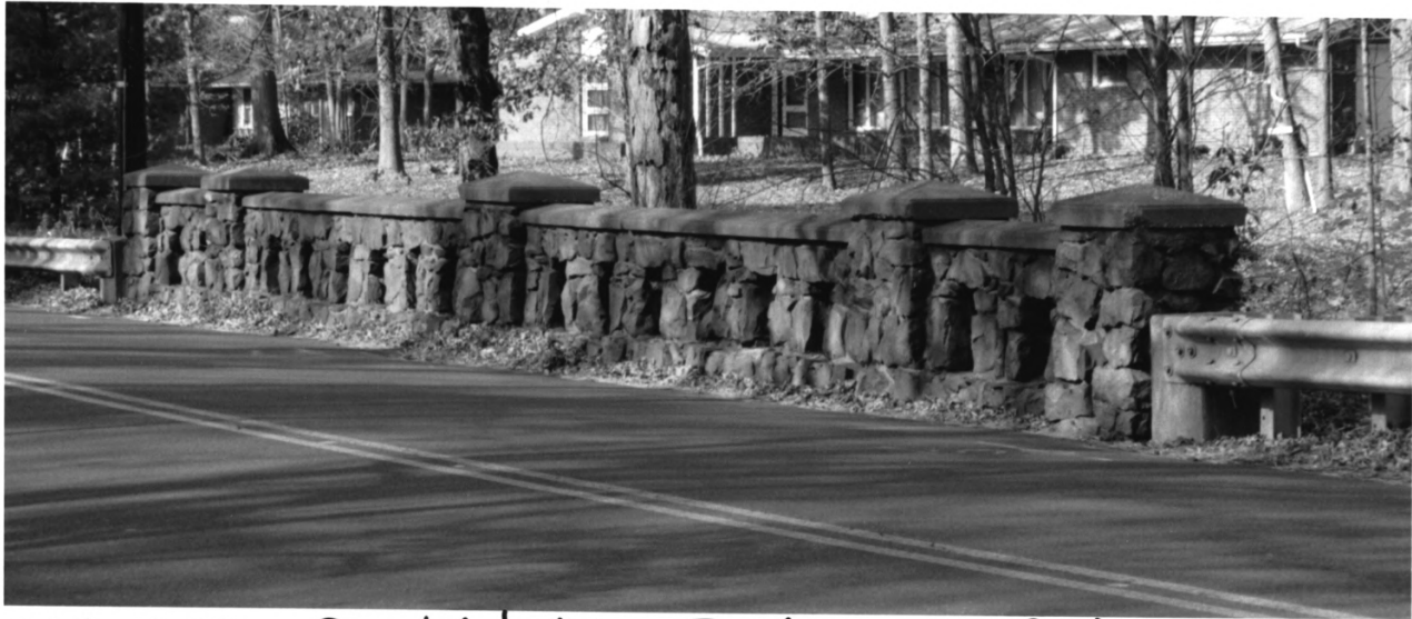
034 023 Randolphville Bridge (2 of 7)
