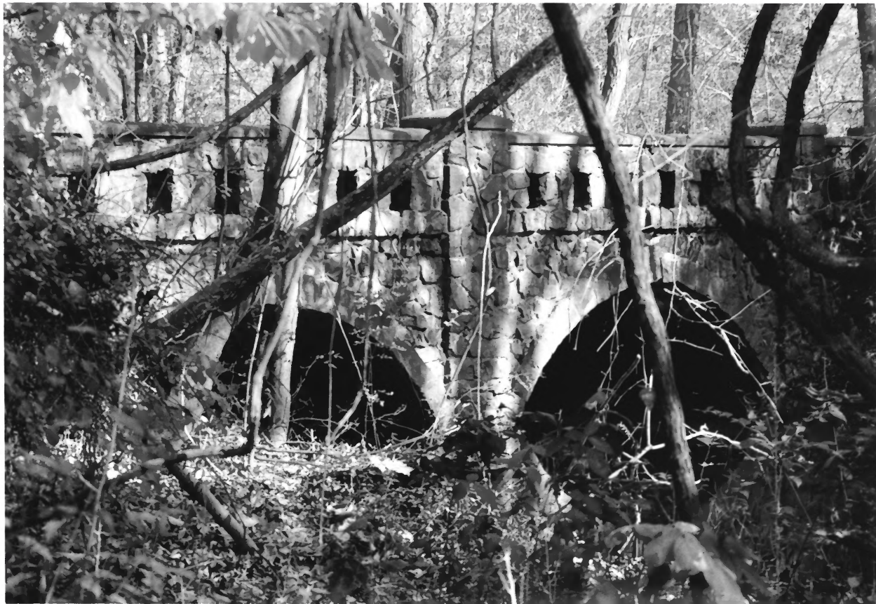
034 023 Randolphville Bridge (1 of 7)
