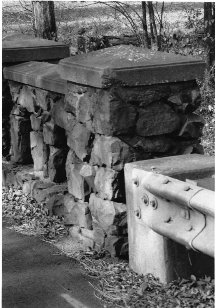
034 023 Randolphville Bridge (4 of 7)
