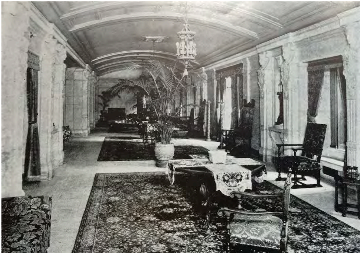
3. View of the gallery looking south, 1930. ( Architecture and Building , vol. 62, February 1930)
