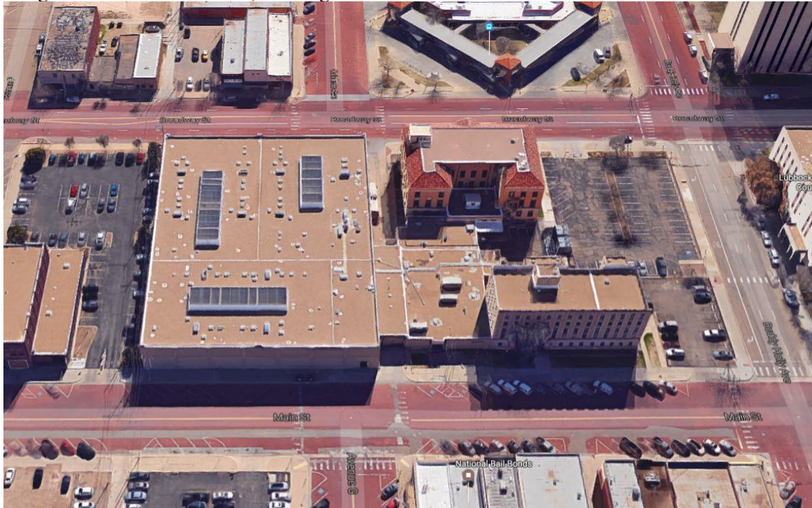
Google Earth: North Elevation, Looking South
