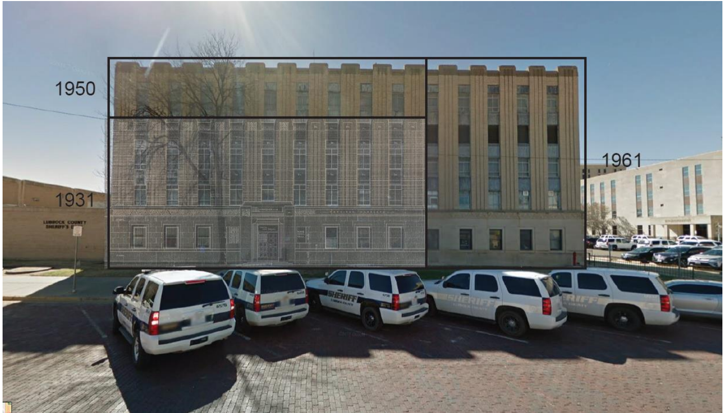
North Elevation Showing Additions by Year (with 1931 Drawing Overlay)
