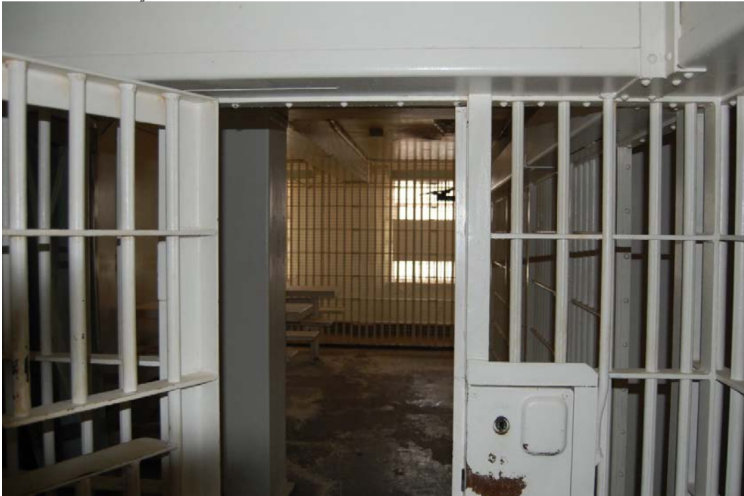
Photo 19: Security Entrance into Fifth Floor Cell Block
