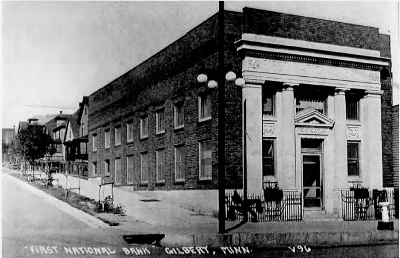
Figure 3: First National Bank building, ca. 1920. This building's bold expression of Classical Revival architecture contrasted with the muted classicism of the previous bank building. Postcard available at Iron Range Historical Society, Gilbert.
