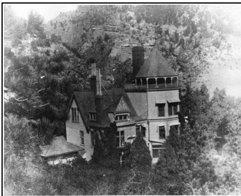
Figure 18. Historic photograph of the remodeled wood-frame house, ca. 1885. Courtesy of the Pikes Peak Library District.
