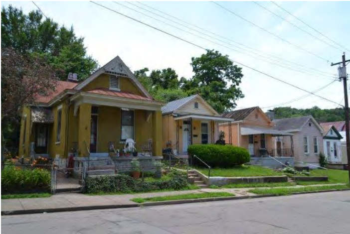
Photo 13: row of Shotgun houses
