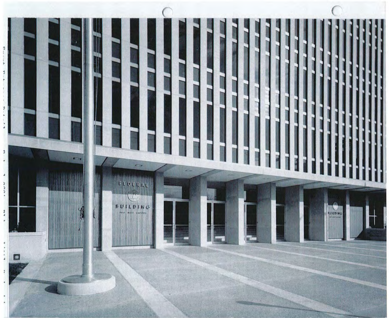
Front entry detail, Federal Building, Little Rock, AR (GSA EDOCs Photo 14055; Photo dated December 14, 1961).
