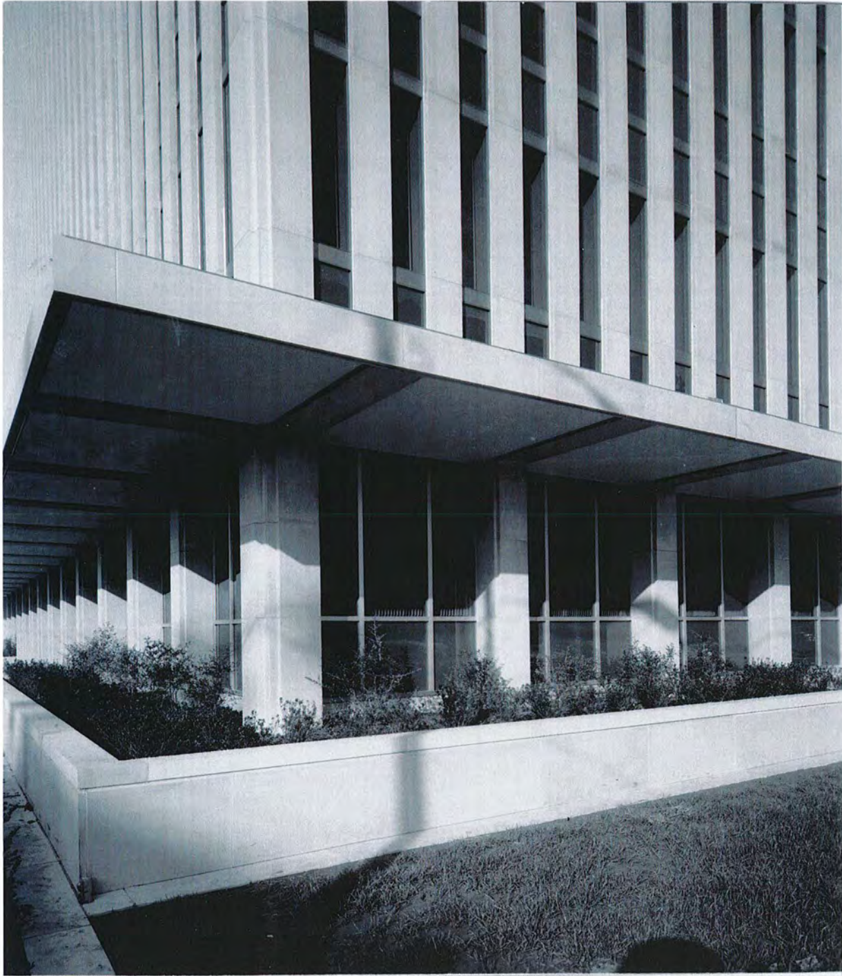
Corner detail, Federal Building, Little Rock, AR (GSA EDOCs Photo 14056; Photo dated December 14, 1961).
