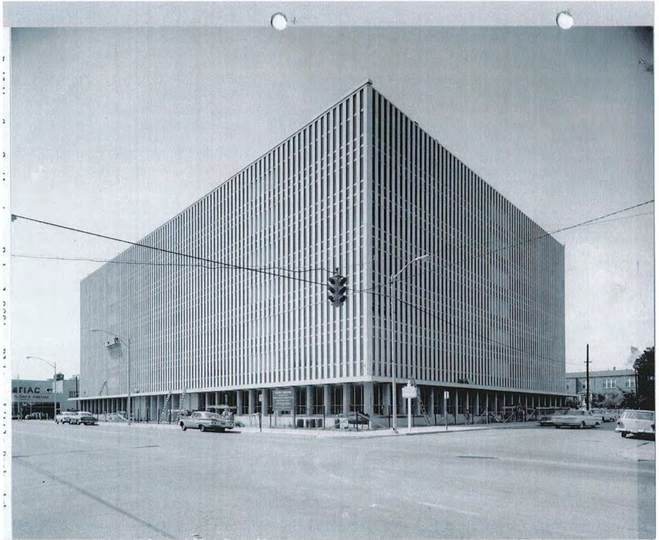
Federal Building (under construction), Little Rock, AR (GSA EDOCs Photo 14026; Photo dated July 31, 1961).
