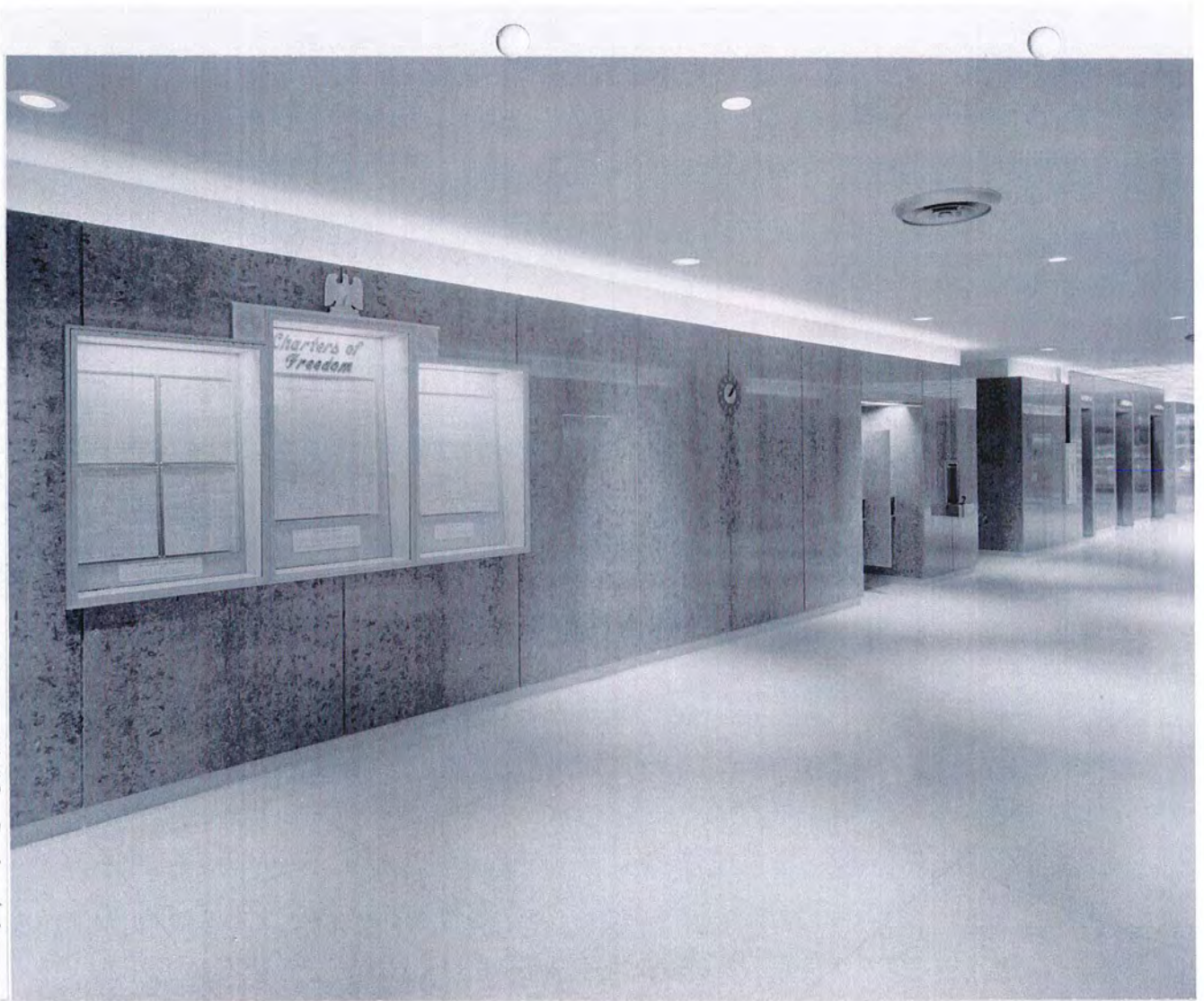
First floor, wall of main lobby, Federal Building, Little Rock, AR (GSA EDOCs Photo 14020; Photo dated December 14, 1961).
