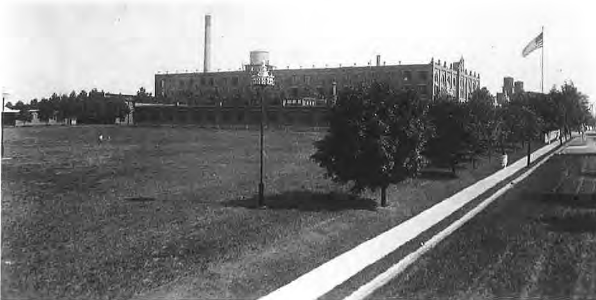
ca. 1915, North Elevation, Martin Birdhouses in foreground Courtesy of United States Playing Card Company Archives – copyright protected
