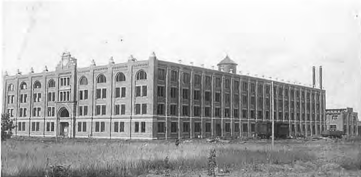
ca. 1899, Under construction
