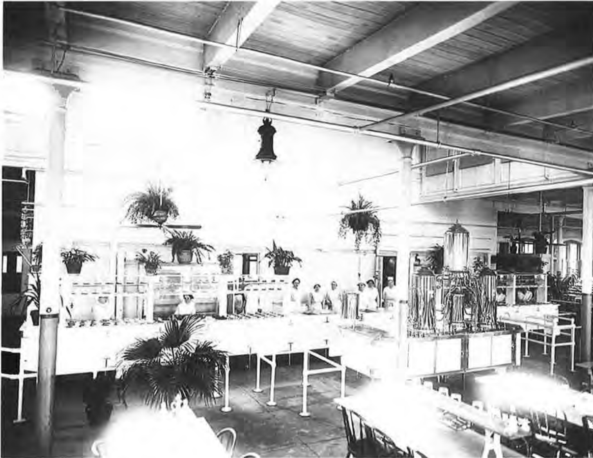
1903 Cafeteria Building, Interior
