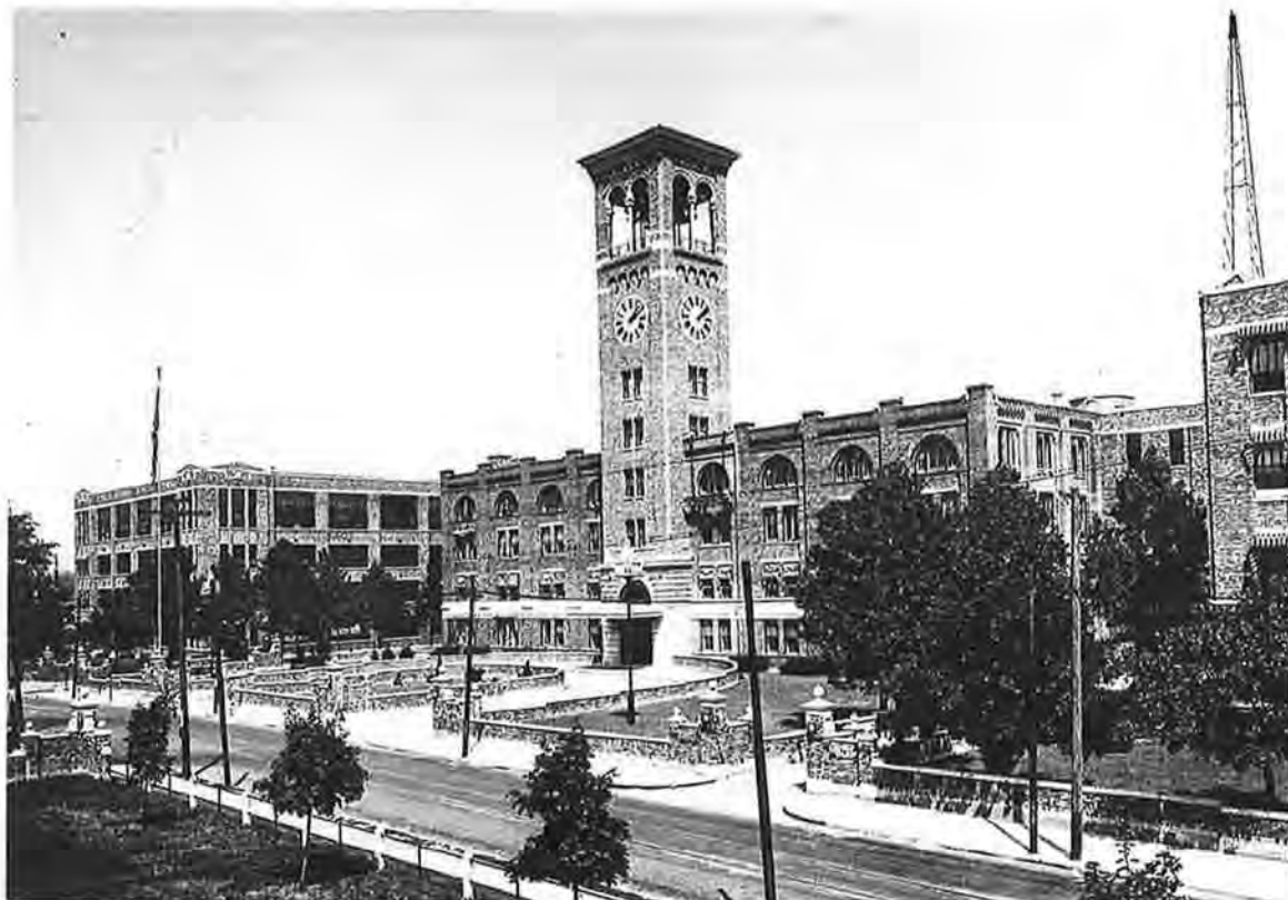
ca. 1922-1930, Radio towers on North and South Additions Courtesy of United States Playing Card Company Archives – copyright protected
