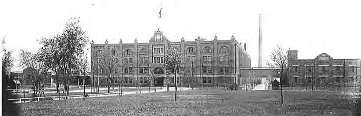
ca. 1905, Façade, Boiler House Smoke Stack added, Park Boulevard under construction Courtesy of United States Playing Card Company Archives – copyright protected
