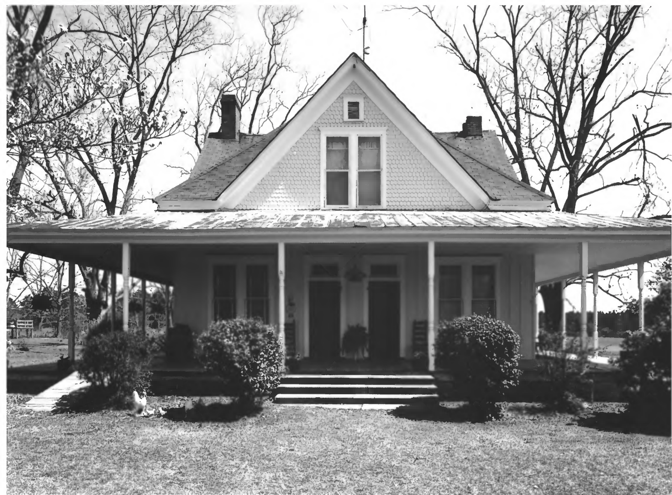
WILSEY, MILES V., HOUSE (KIMBALL, CHARLES W., HOUSE) BEN HILL COUNTY, GEORGIA PHOTOGRAPH 2 OF 12
