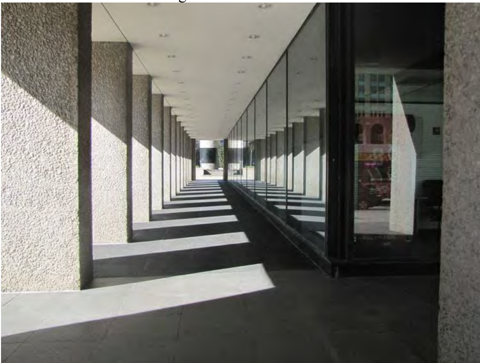
TX_Dallas County_One Main Place_0008 West arcade – camera facing north
