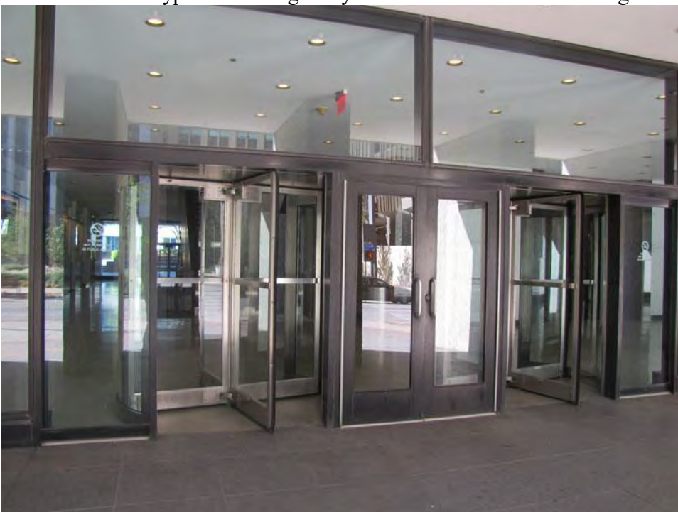
TX_Dallas County_One Main Place_0010 Exterior view of typical building entry at street level – camera facing north
