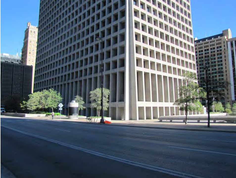
TX_Dallas County_One Main Place_0005 Northwest oblique – detail of lower elevation
