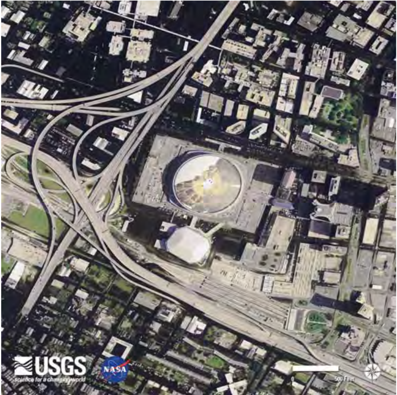
Figure 8. USGS Aerial satellite view of Hurricane Katrina damage to Superdome's roof, including flooding; Source: USGS
