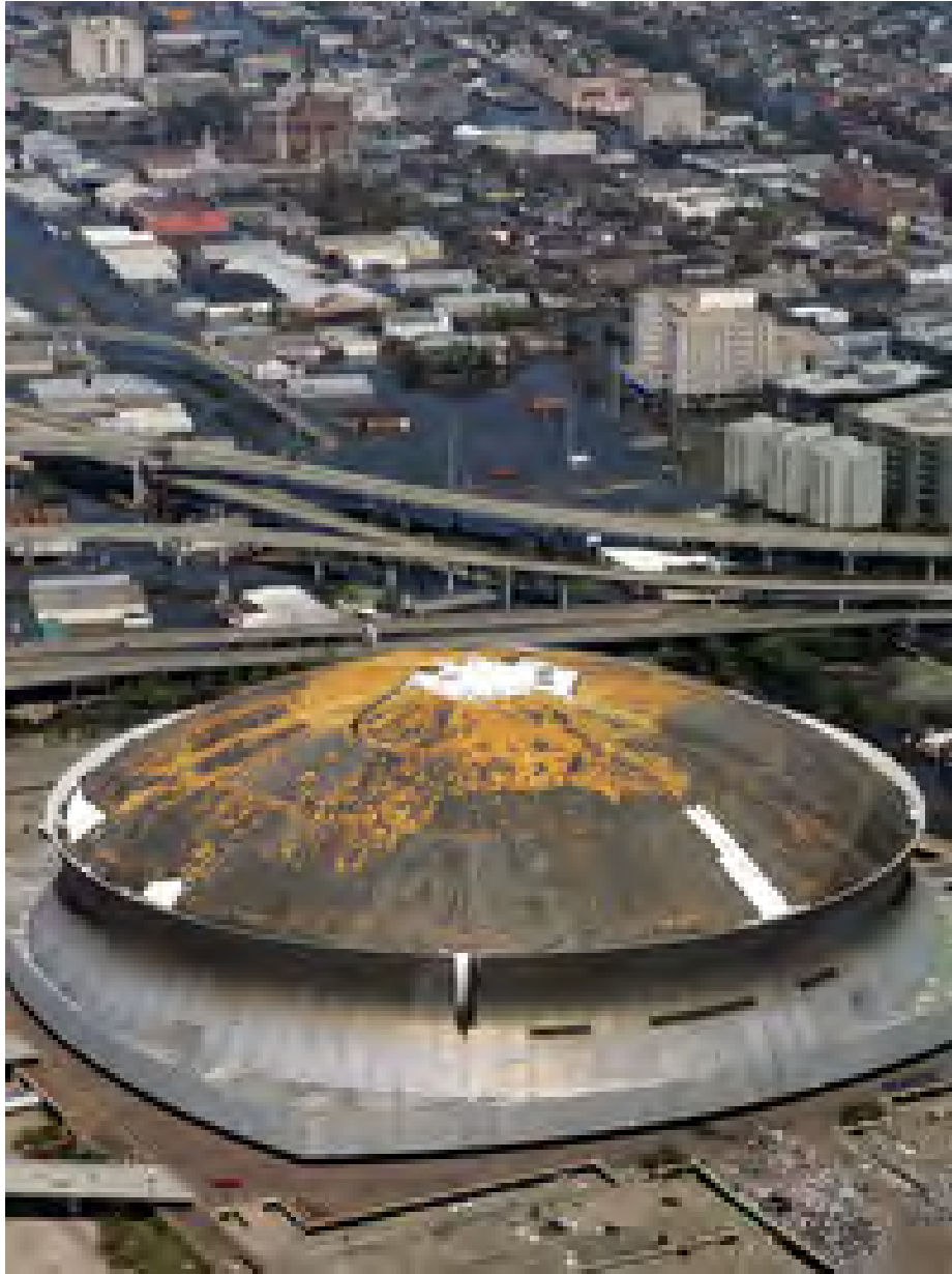
Figure 7. Roof damage caused by Hurricane Katrina; Source: www.media.npr.org
