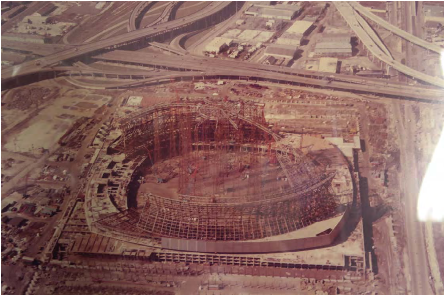
Figure 22. Construction photo with tension ring for lamella dome; Source: Curtis and Davis Office Records, Southeastern Architectural Archives, Tulane University
