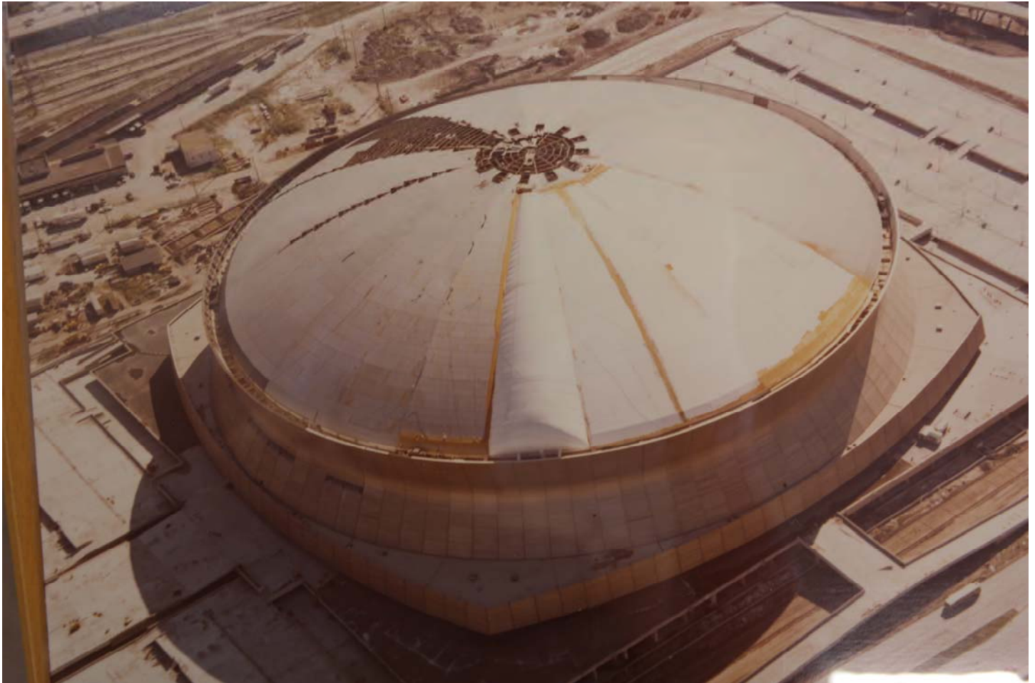
Figure 19. Construction photos of roof; Source: Curtis and Davis Office Records, Southeastern Architectural Archives, Tulane University
