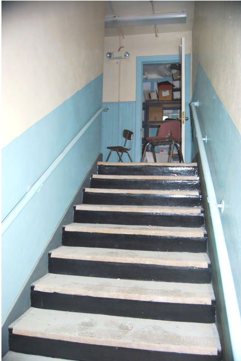
H-17. Typical stair tower, 1915 section of school.
