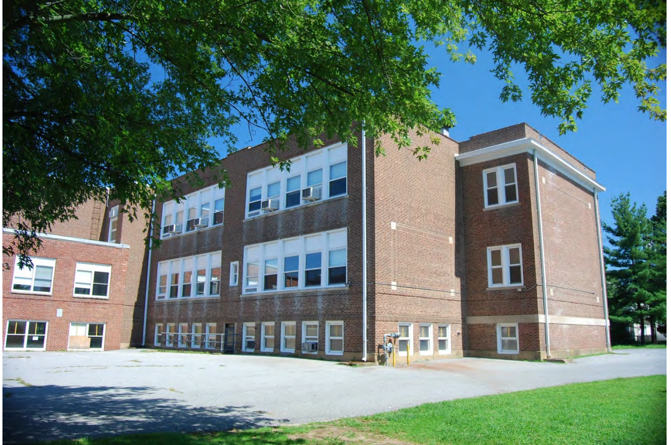
H-7. Looking NW at rear wall of 1915 school; 1925 classrooms identified by lack of detailing on left side wall
