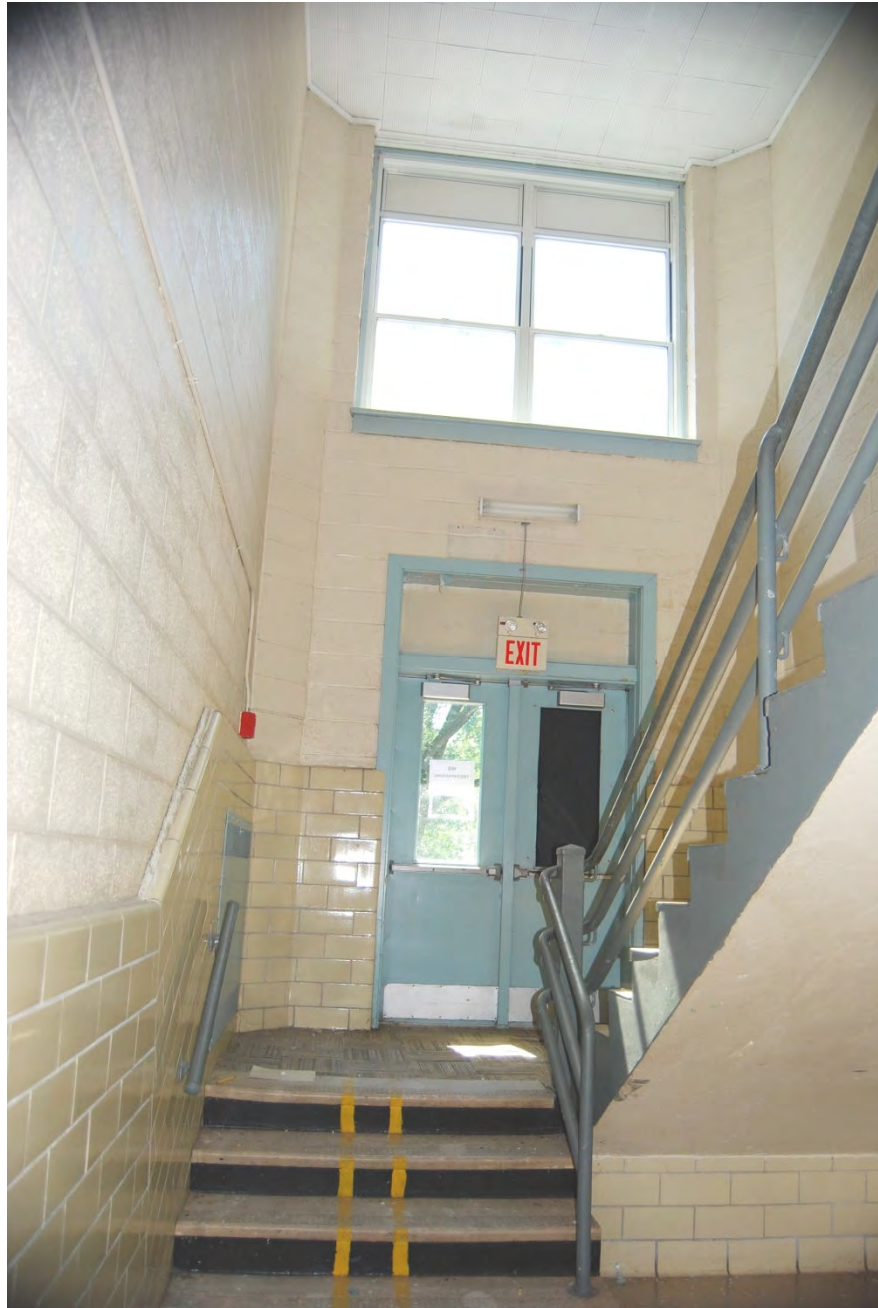
H-19. Looking S in stair tower in 1952 addition.
