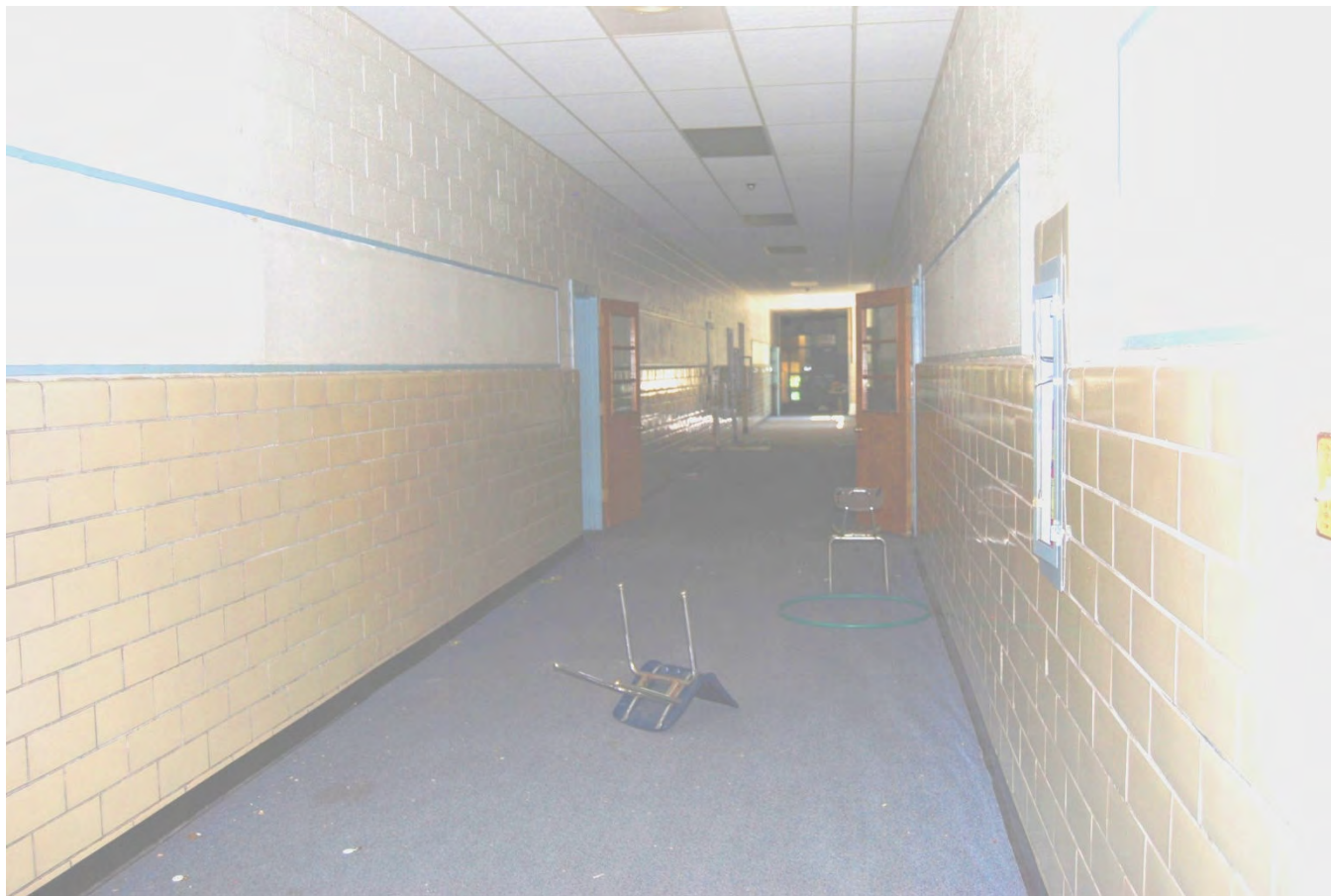
H-20. Looking W in 2 nd floor corridor in 1952 addition.
