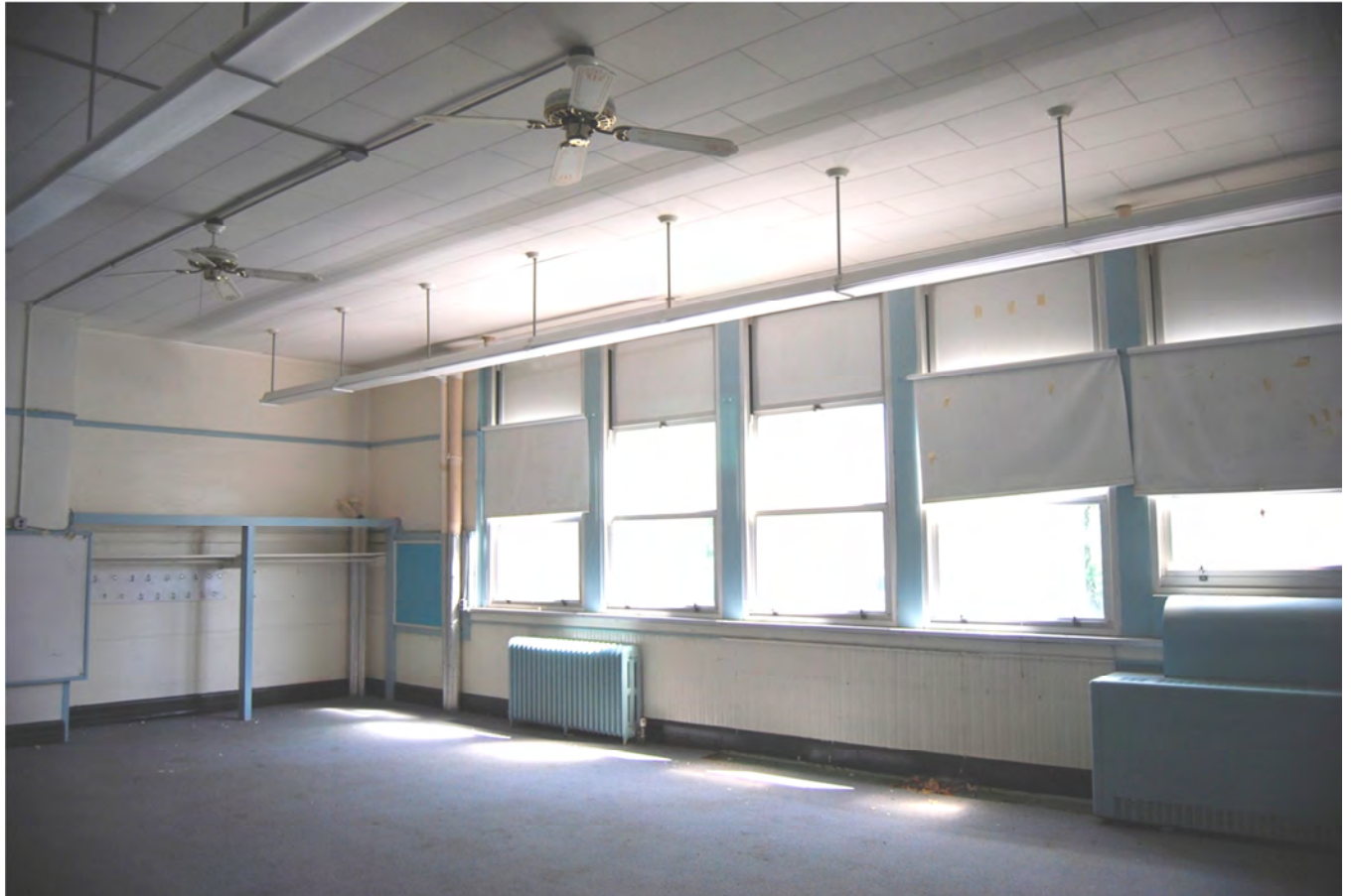
H-16. Typical classroom, 1915 and 1927 sections of school
