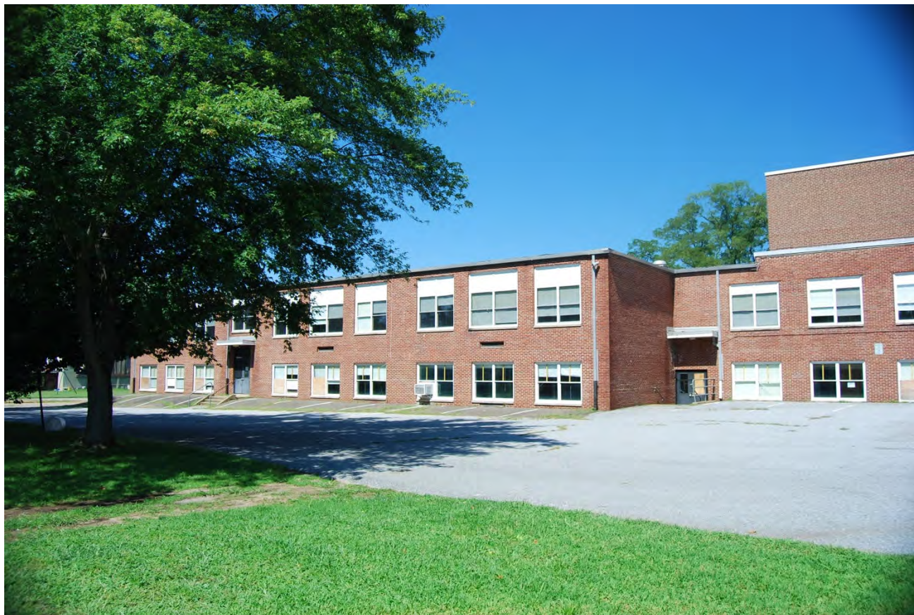
H-8. Looking NW at S (side) façade of 1952 addition.
