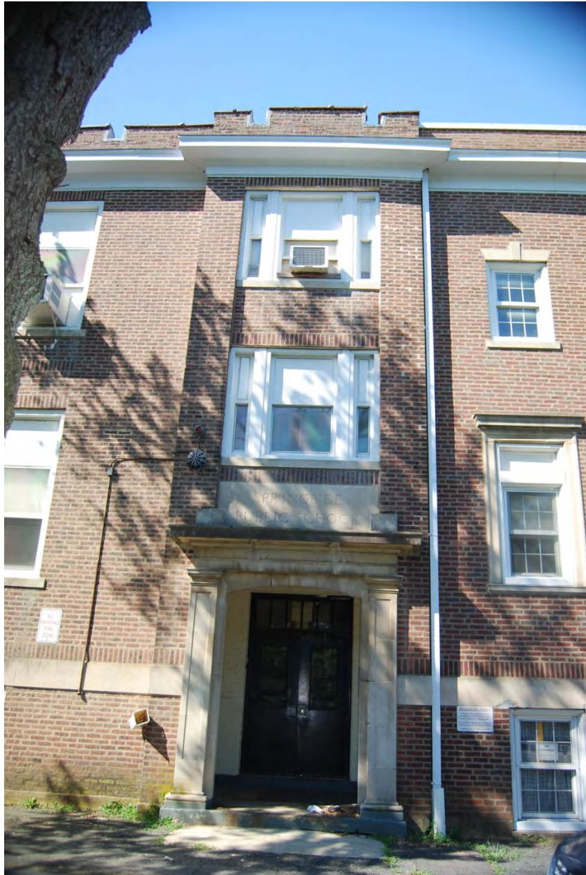
H-5. Looking W at center entrance on E (main) façade. This entrance was originally the north entrance to the school and became the center entrance with the 1927 addition.
