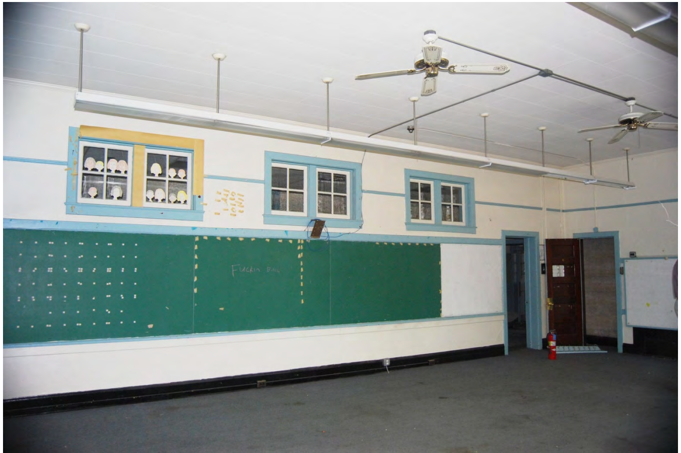
H-15. Typical classroom, 1915 and 1927 sections of school
