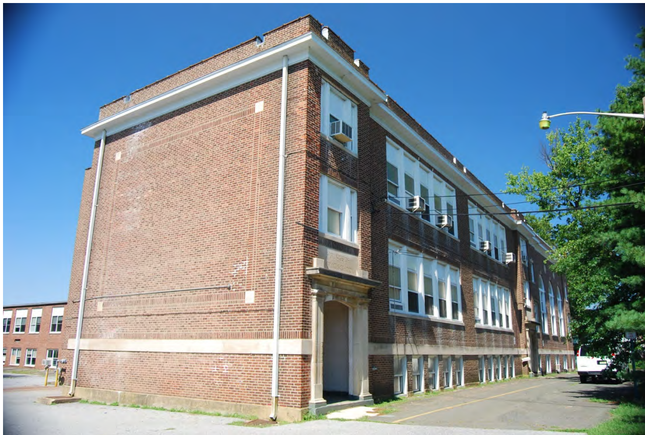
H-6. Looking S at N (side) and Et (main) elevations of 1927 section of Springside Public School.
