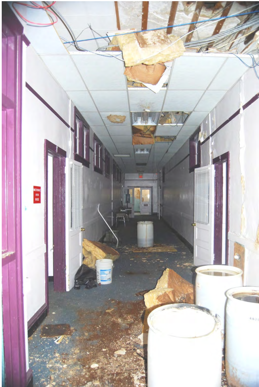
H-18. Looking S is third floor corridor of 1915 school
