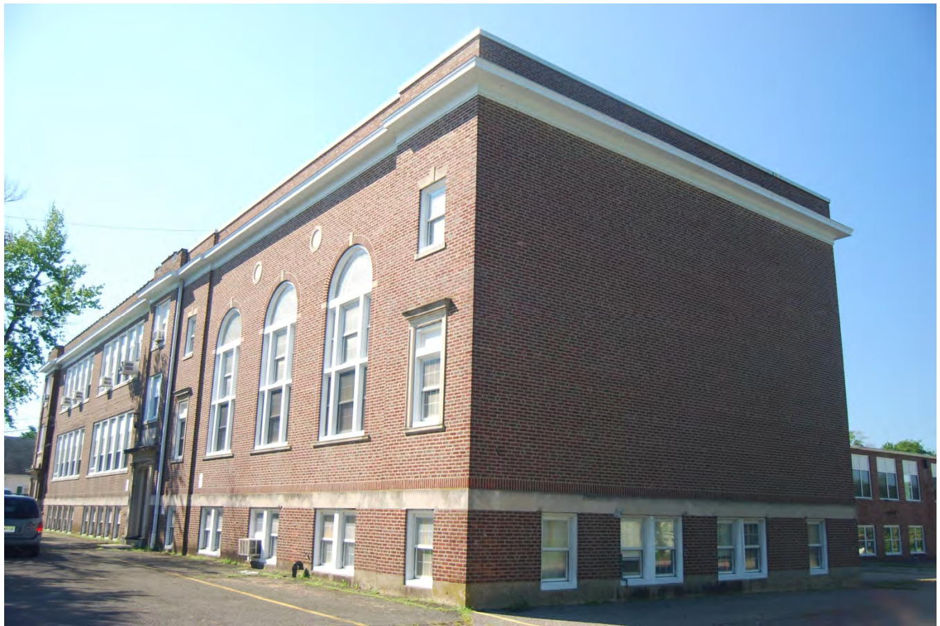
H-4. Looking N at S (side) and E (main) elevations of 1915 section of Springside Public School.
