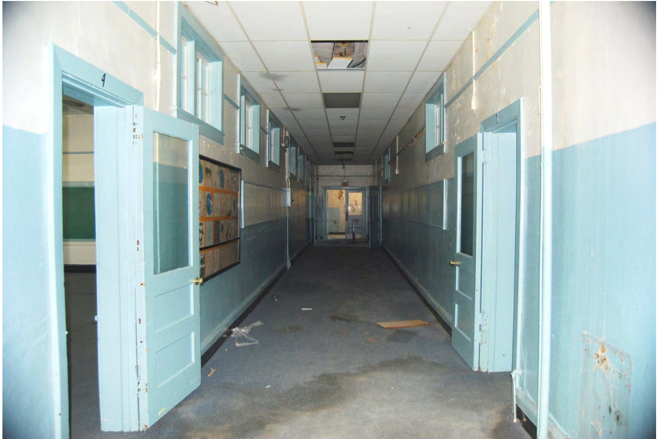
H-14. Looking S along second floor corridor in 1915 section of school.
