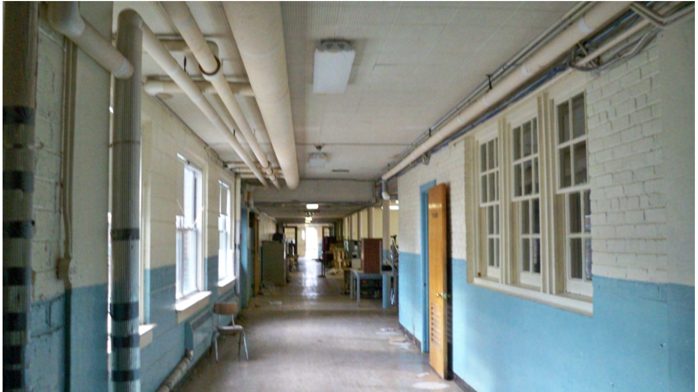
H-12.Looking S in corridor between 1927 kitchen and 1952 wing, ground floor
