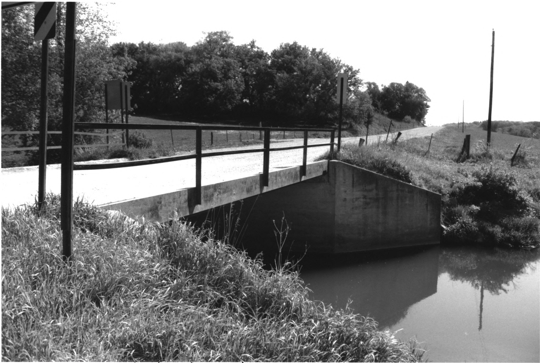
Nansen Agricultural Historic District Bridge no. 20502 (non-contributing), GD-HOL-043 Goodhue Co., Mn 013354-1
