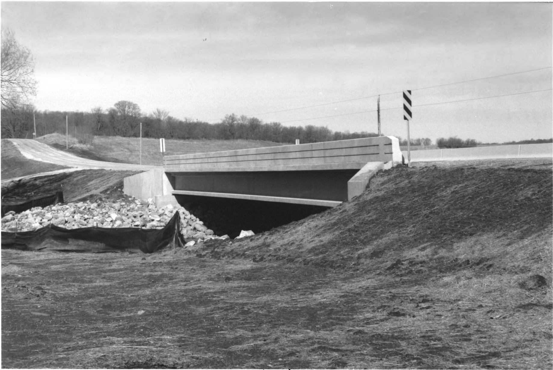
Nansen Agricultural Historic District Bridge # 25578 (non-contributing) 6D-WAR-27 Goodhue Co., Mn 013329-14A/15
