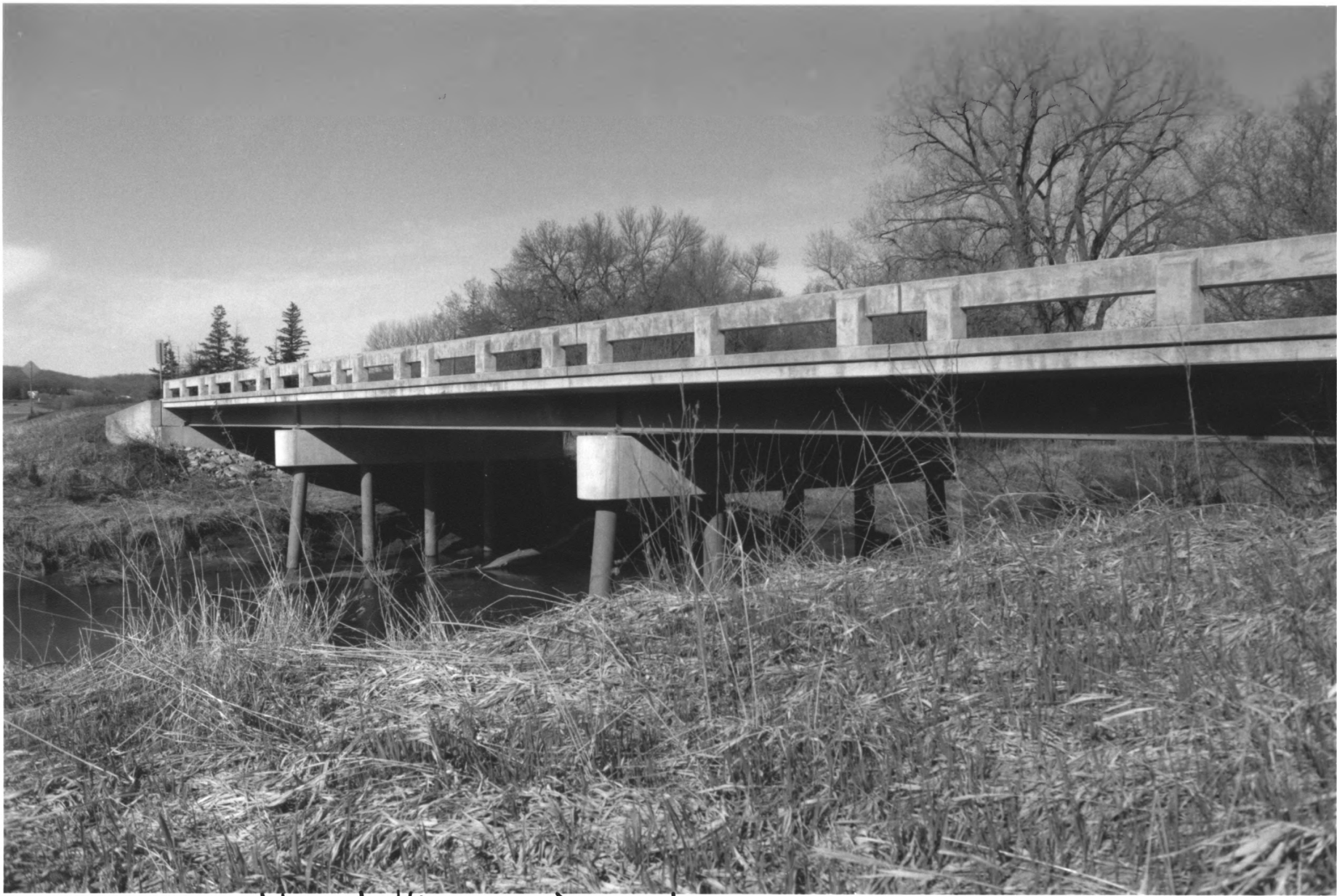
Nansen Agricultural Historic District Bridge # 25509 (non-contributing) 6D-WAR-025 Goodhue Co., MN 013329-9A110
