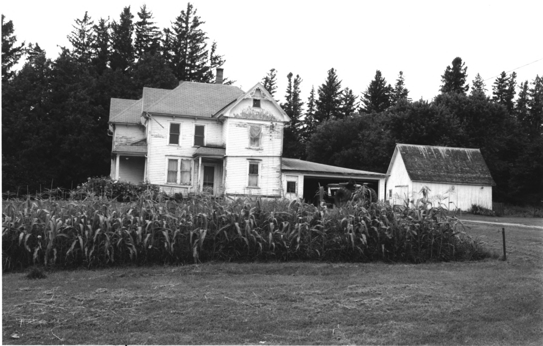
Nansen Agricultural Historic District Martin S. Gjellum Farm, GD-HOL-045 Goodhue Co., mn 013417-16A/17
