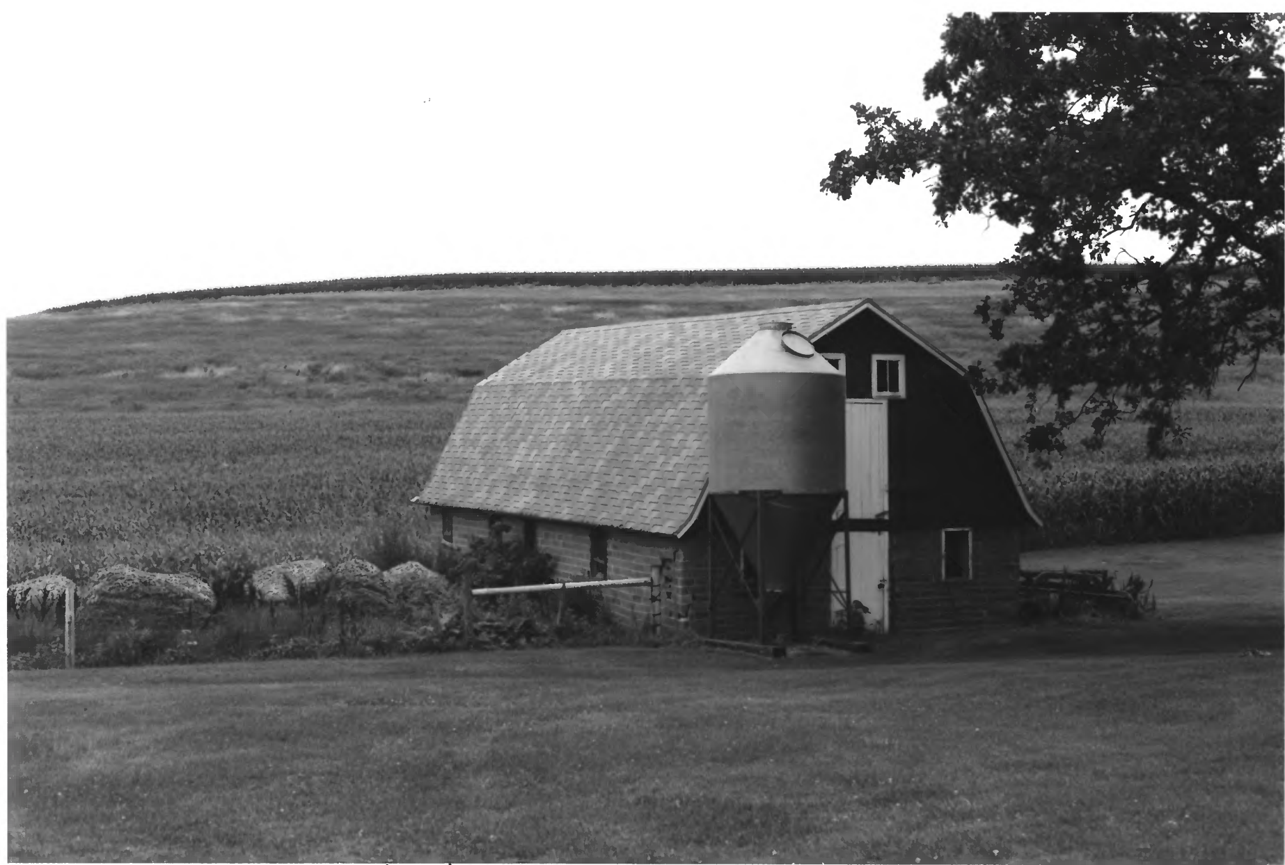
Nansen Agricultural Historic District Martin A. Flom Farm, GD-HOL-030 Goodhue Co., Mn 013413-10/10A
