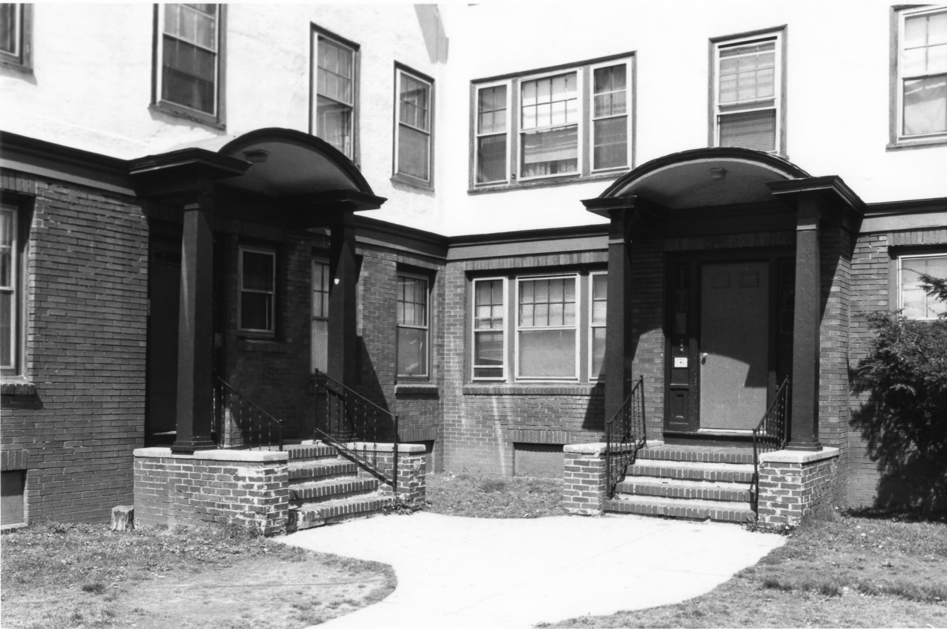
Ontario Apartments Providence City., Prov., R.I. Photo # 2 of 9
