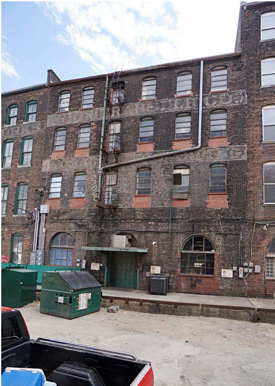
Figure 24: North façade, view facing southeast.
