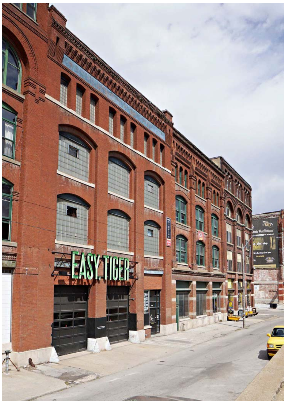
Figure 17: South façade with streetscape, view facing northeast.
