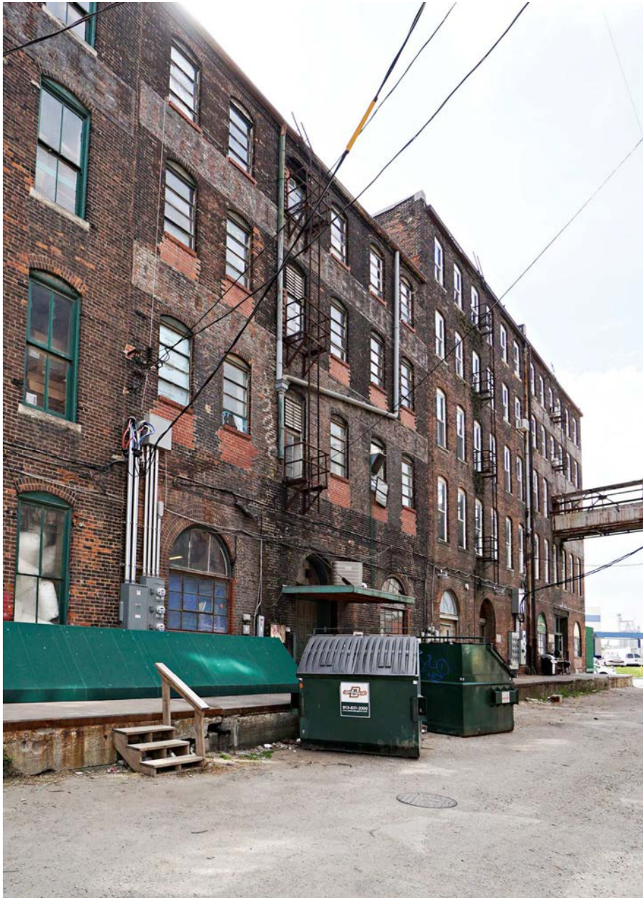
Figure 23: North façade, view facing southwest.
