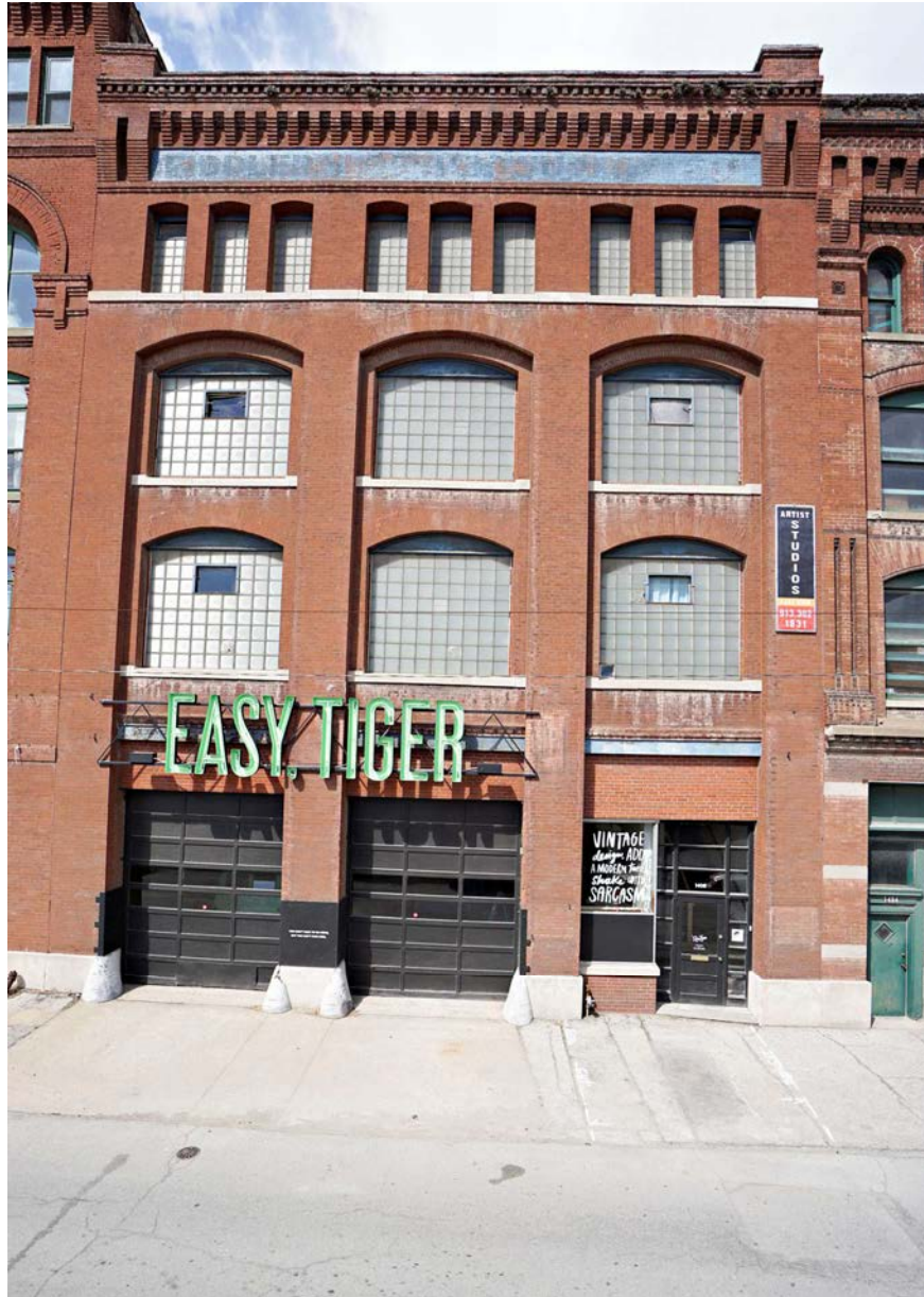
Figure 18: South façade, view facing north.
