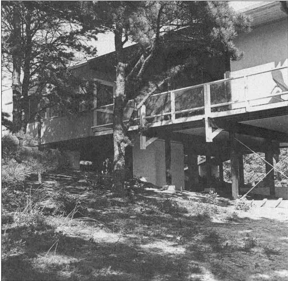
View looking at northeast west elevation
