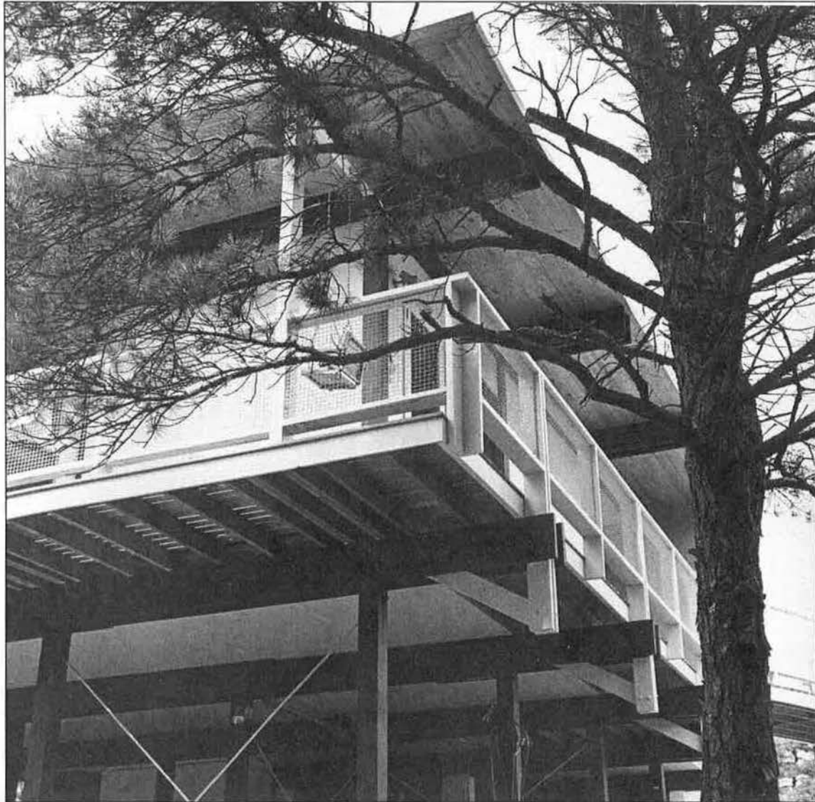
View looking at northwest at facade and south elevation
