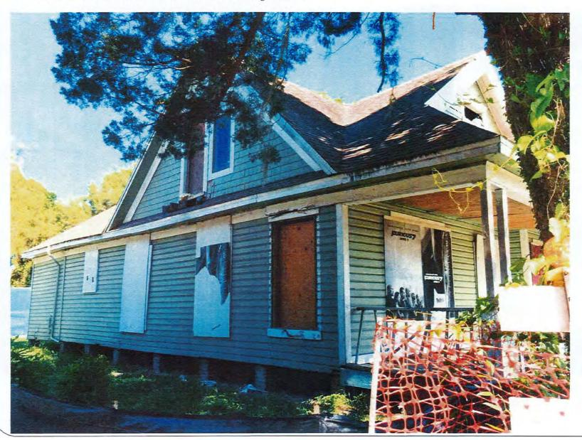
Southwest side rear of house, showing proximity and placement of the other two Morgan St. houses. Brick pier foundation covered with sand.
