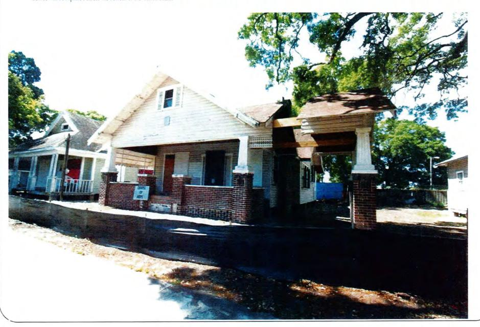
• North side of house, showing north end of porte cochere gable and missing steps to porch from porte cochere. Noted brick repair to exterior chimney and porch using old bricks and new brick masonry piers. Note poor condition of wood windows which will be restored.
