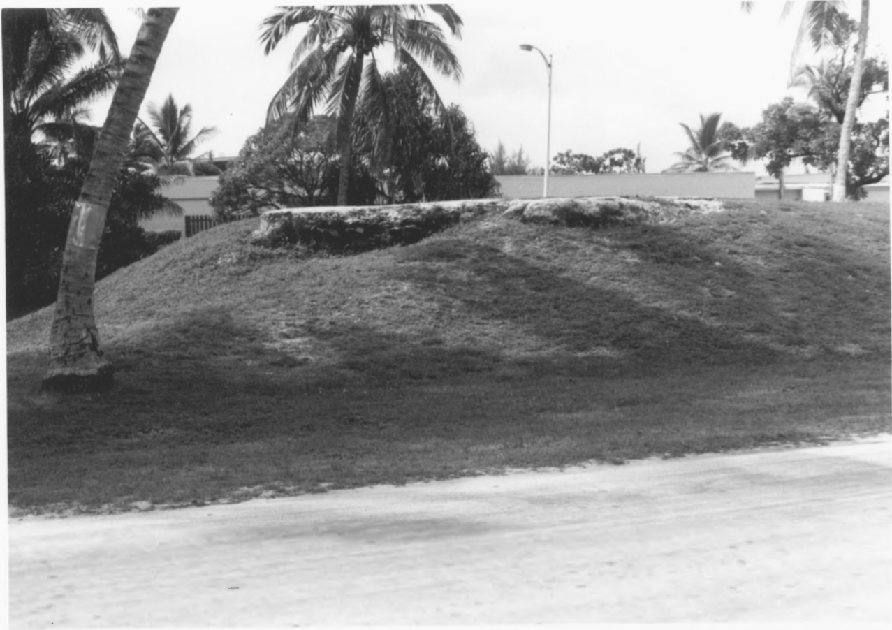
10. Japanese twin-mount, dual-purpose 127mm gun emplacement at the north end of Kwajalein Island, one of the last positions to be captured. Because of the island's low elevation, the Japanese constructed mounds for these weapons. This is called "Bunker Hill."
