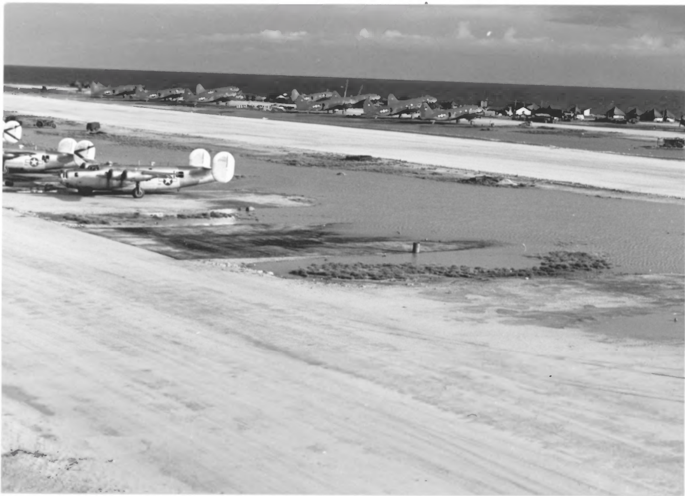
3. Seventh Air Force bomber field constructed on top of Japanese field on Kwajalein Island. Note the absence of vegetation.
