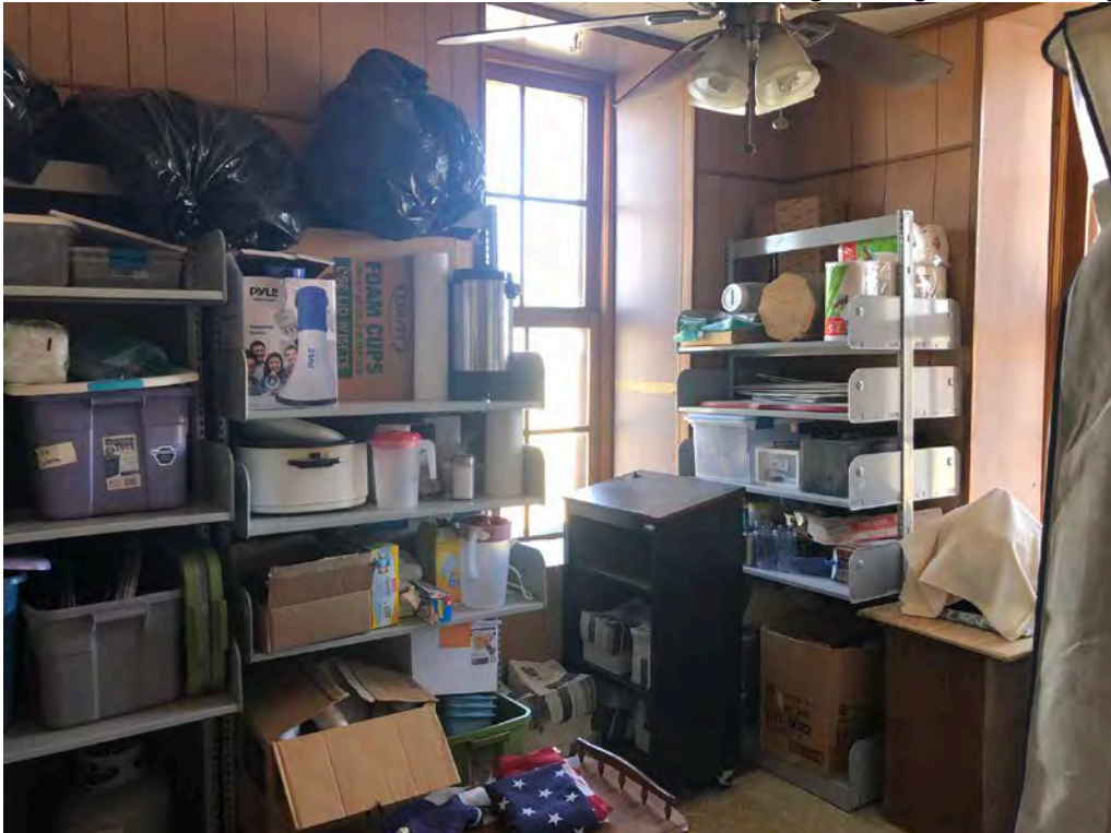
Photo 8: A small office is on the south side of the 1909 building in the gable end. (May 18, 2019)
