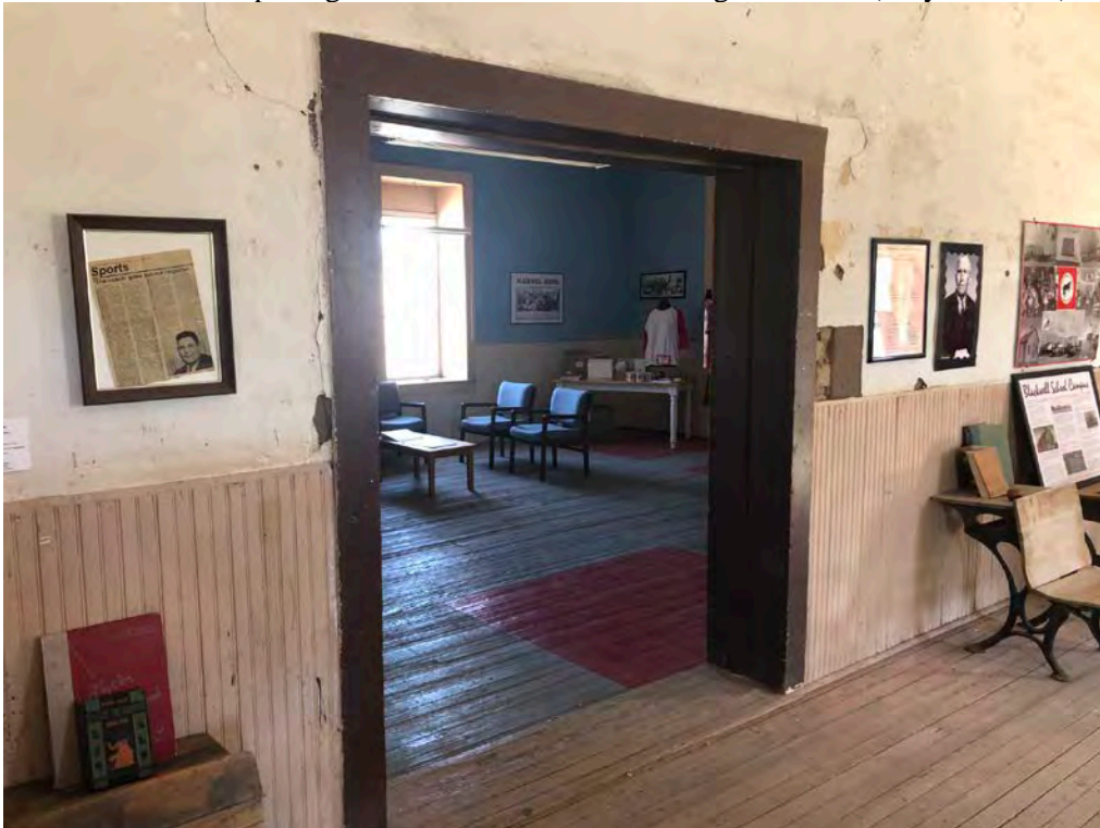
Photo 10: Interior opening between classrooms. Looking northeast. (May 18, 2019)
