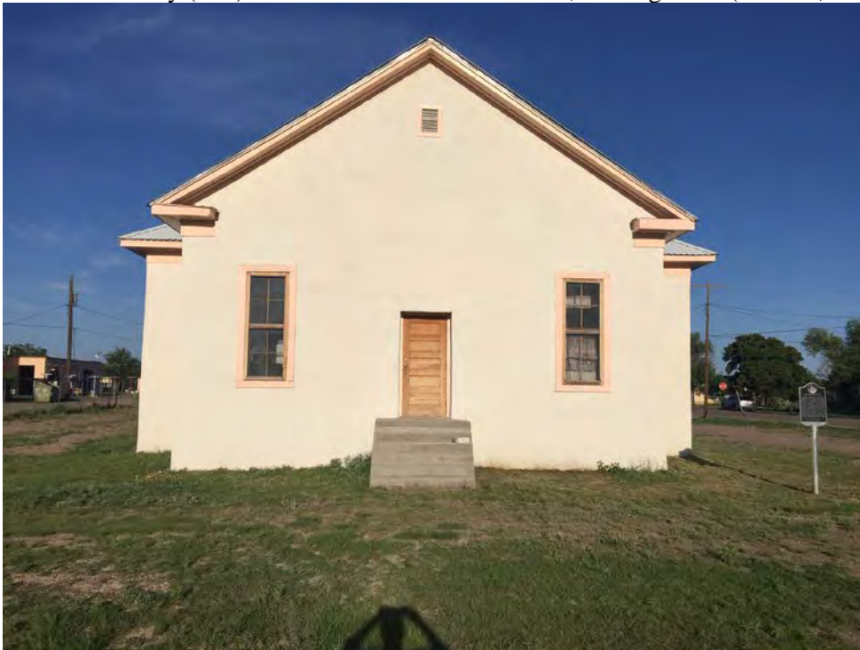
Photo 2: Primary (east) elevation of 1909 schoolhouse, looking west. (June 14, 2019)
