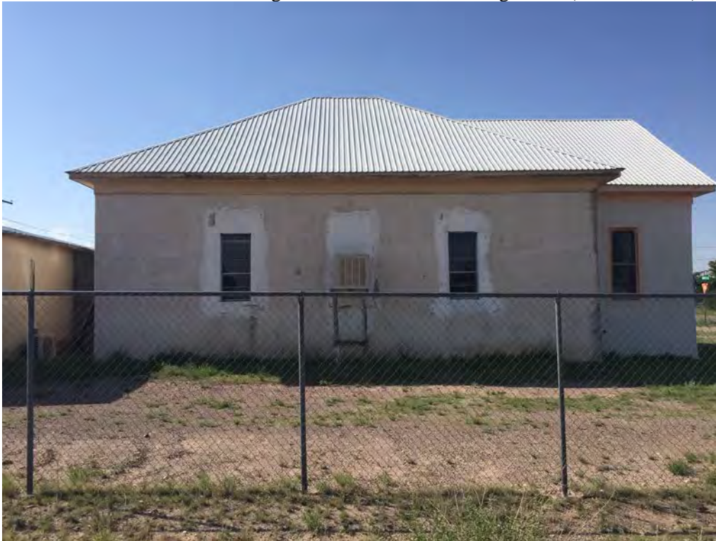
Photo 5: South elevation showing 1909 schoolhouse, looking north. (June 14, 2019)
