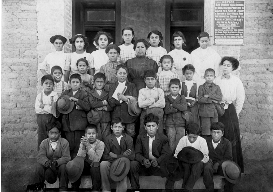
Figure 5: Mary Shannon's class (c. 1910) standing at the front entrance. The exterior was plastered, and entry vestibule enclosed within five years of the photograph. Source: Blackwell School Alliance
