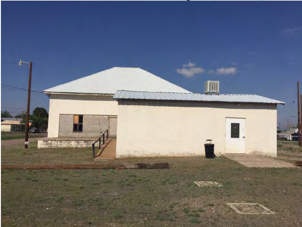
Photo 4: West elevation of 1909 schoolhouse, looking east. (June 14, 2019)
