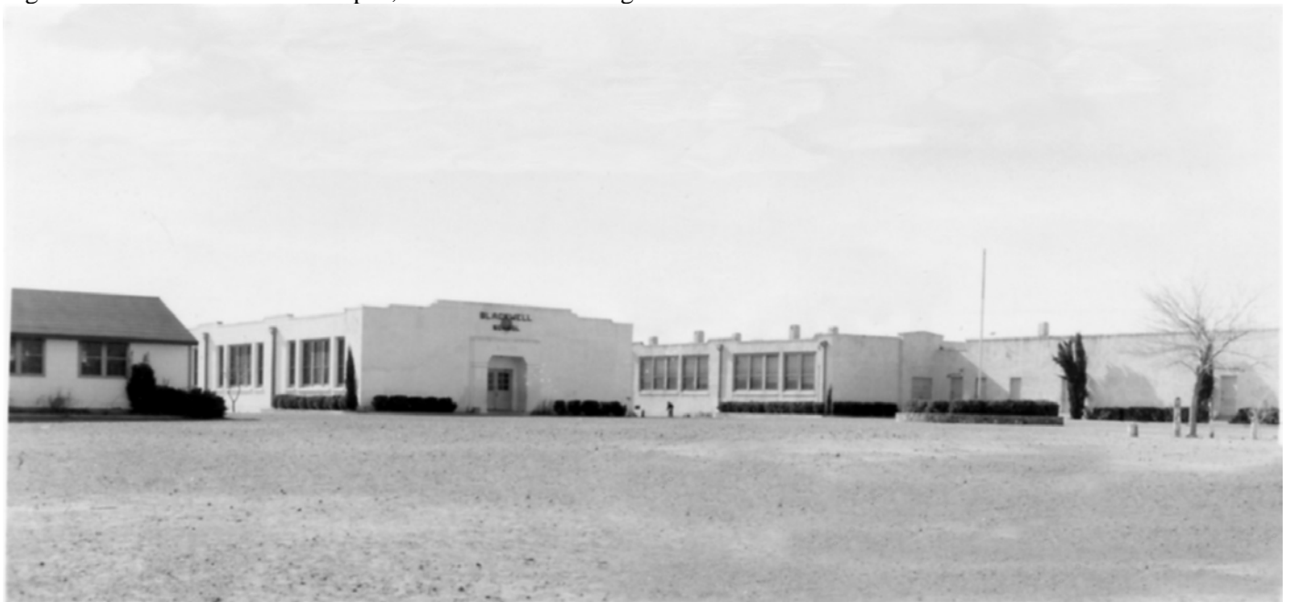
Figure 8: Blackwell School Campus, c. 1950. The buildings shown were razed in 1969.
