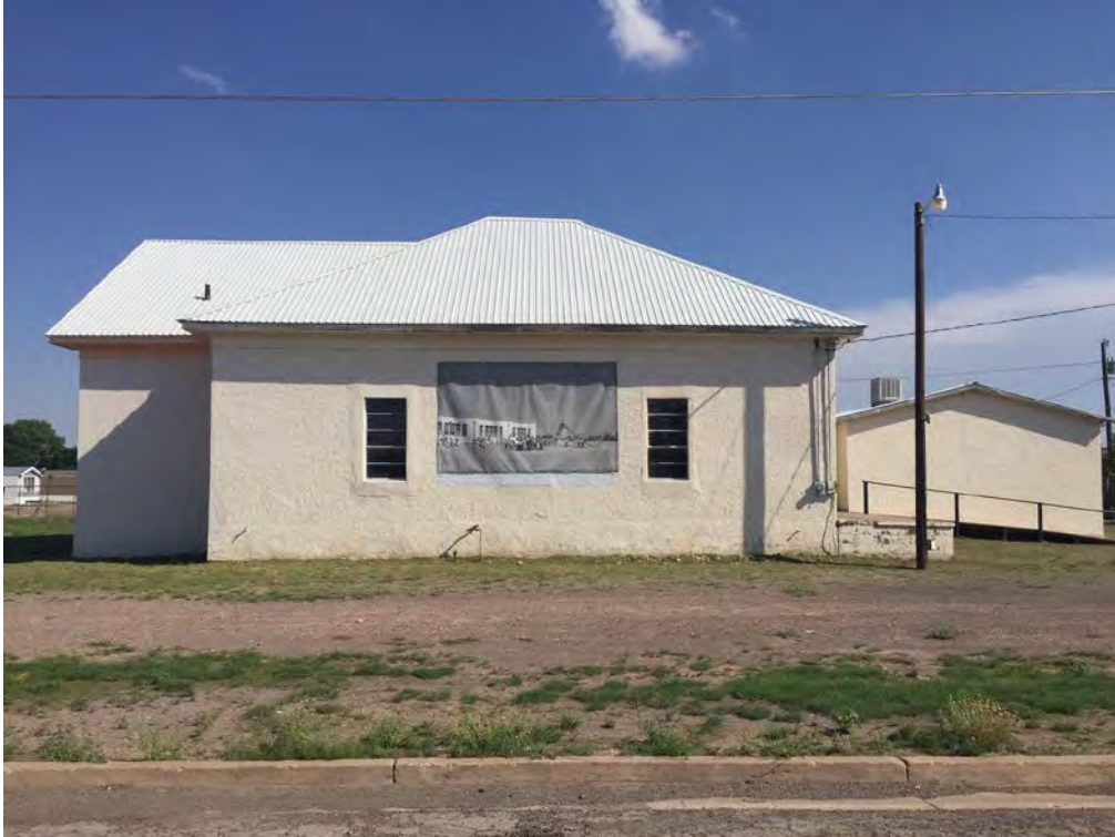
Photo 3: North elevation of 1909 schoolhouse, looking south. (June 14, 2019)
