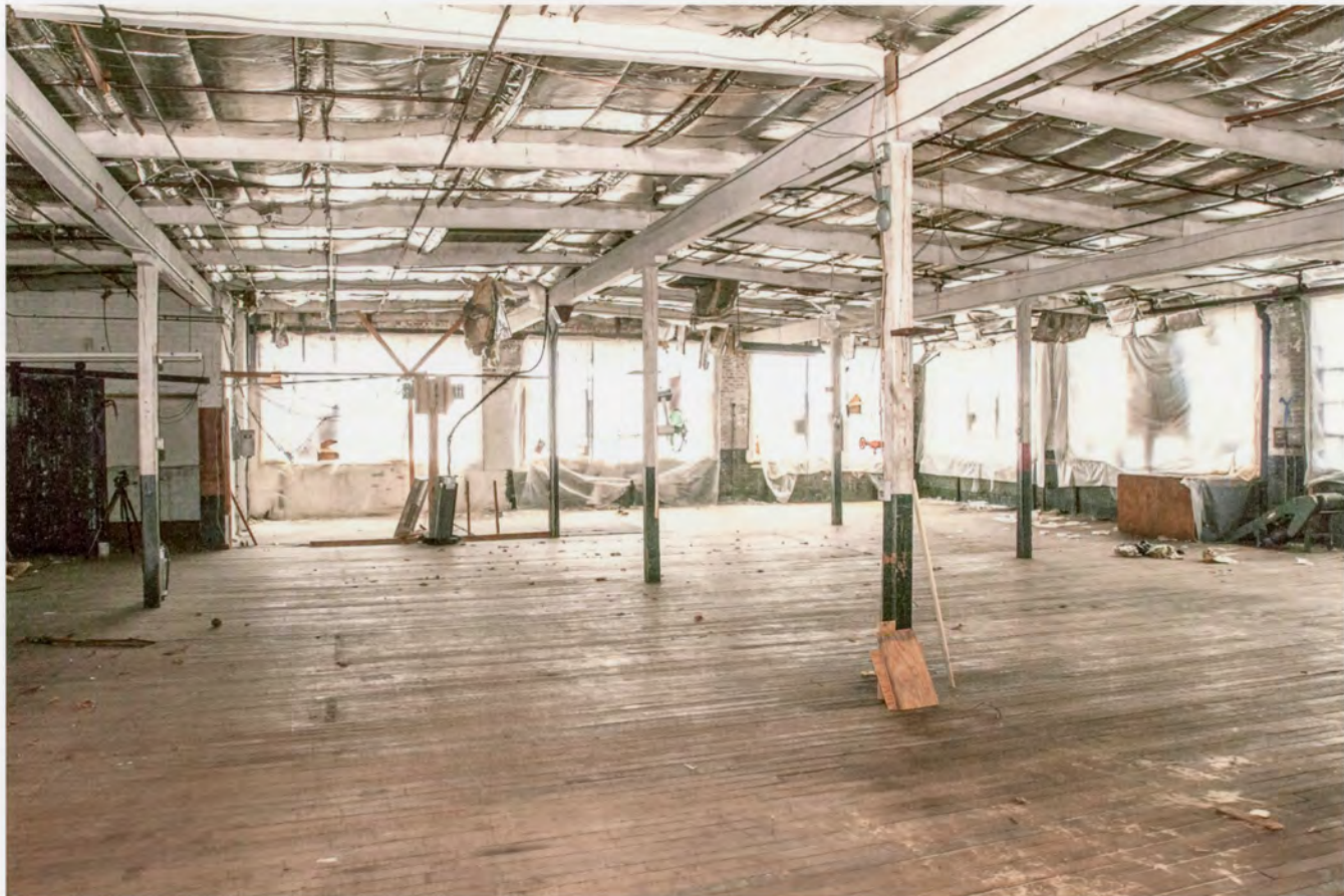
Photo 14. Le Roy Shirt Co., Norwalk, Fairfield County, Connecticut. Second floor interior view east. August 5, 2011 Tod Bryant
