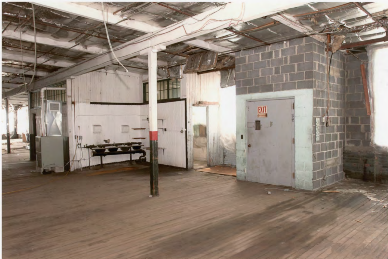
Photo 16. Le Roy Shirt Co., Norwalk, Fairfield County, Connecticut. Second floor interior view northeast showing sinks, locker room and elevator. August 5, 2011 Tod Bryant
