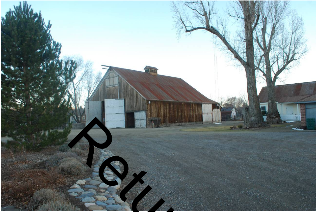
Photograph 5 – Barn, viewed from central driveway, looking southeast.
