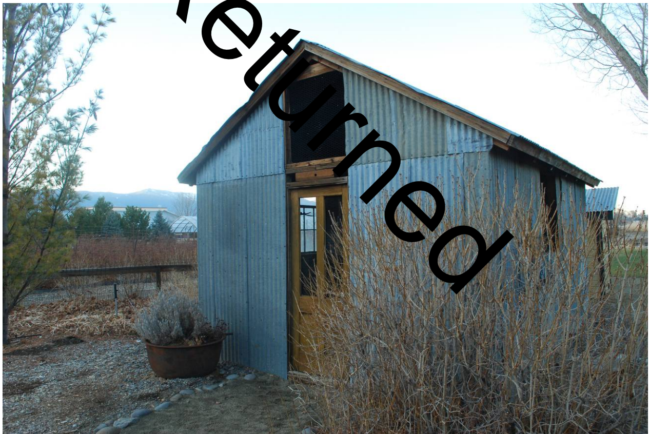
Photograph 115 – Workshop, south façade, looking northwest.
