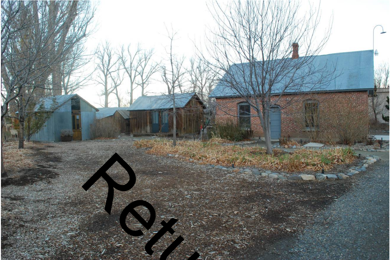
Photograph 2 – Example of cluster arrangement, showing Creamery (right), Bunk Shed (center), and Workshop (left), looking northeast.
