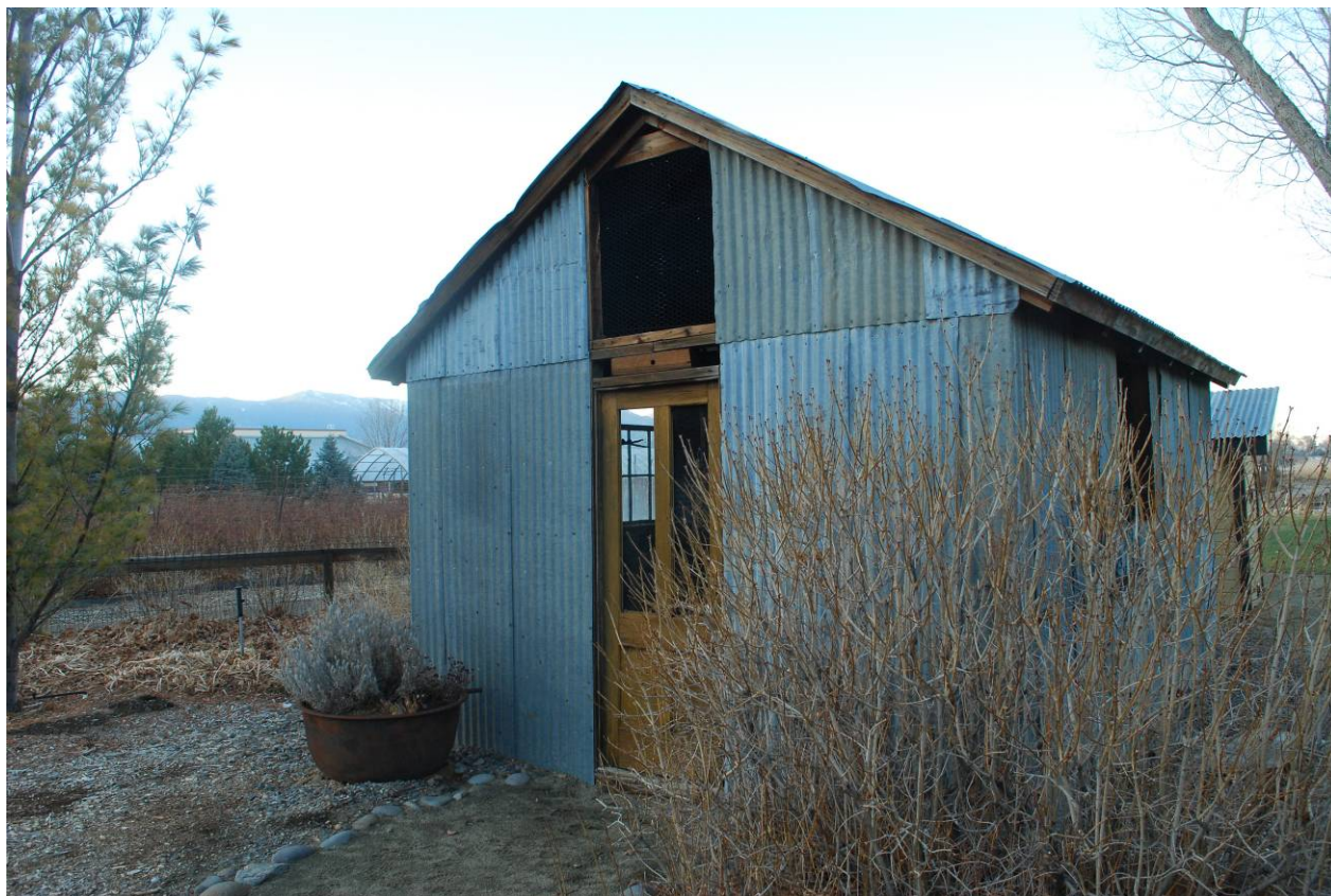
Photograph 15 – Workshop, south façade, looking northwest.
