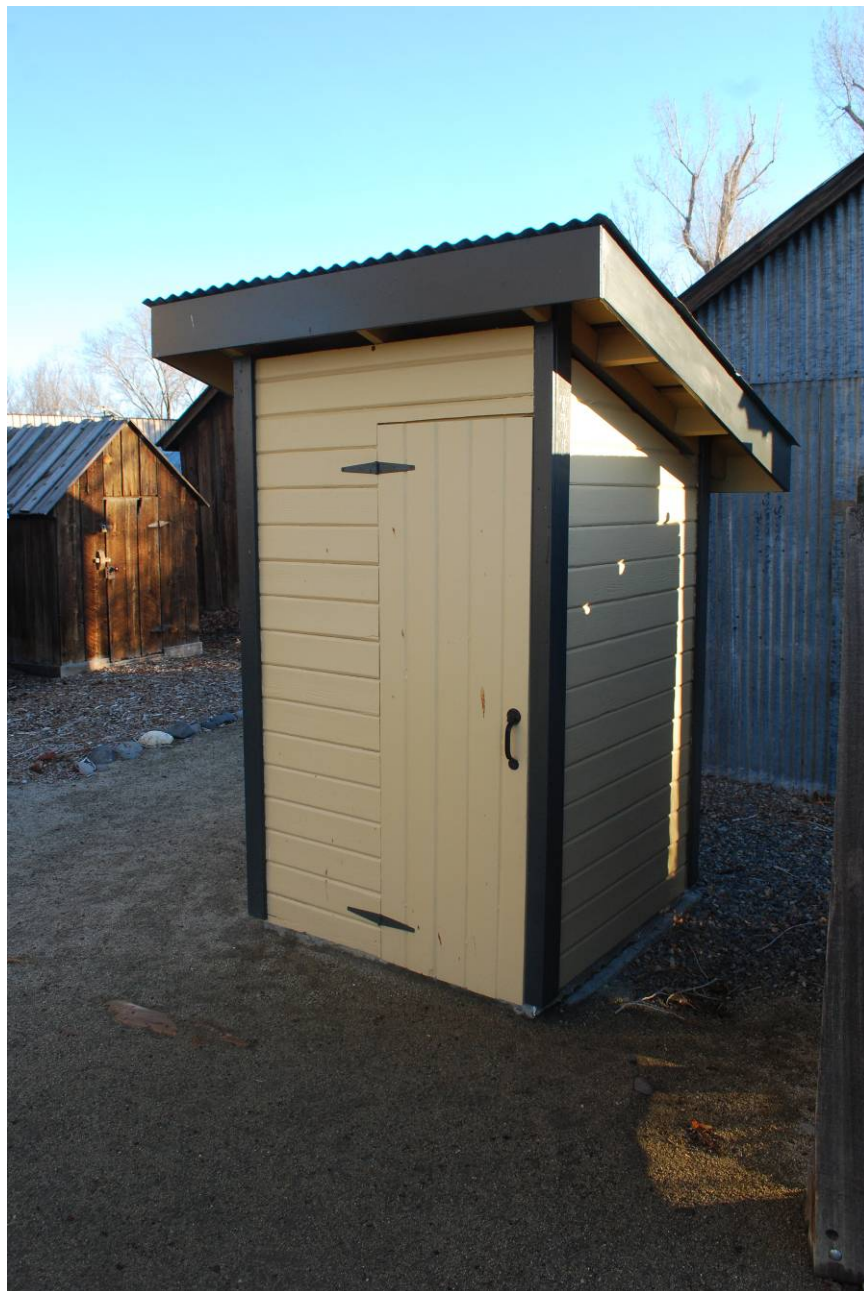
Photograph 17 – WPA Privy north façade, looking southeast.
