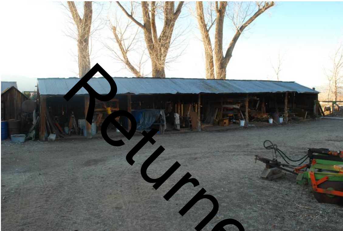
Photograph 148 – Large Loafing Shed, east façade, looking west.
