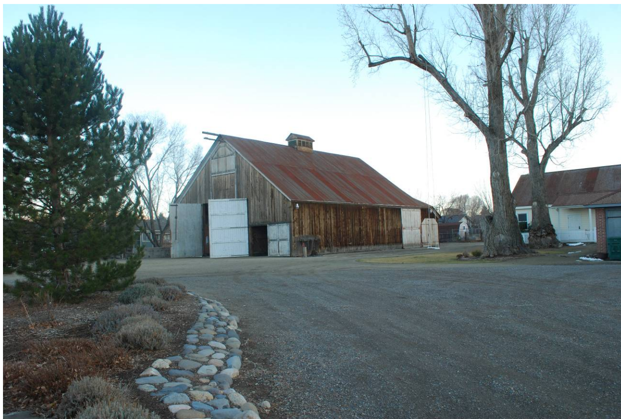
Photograph 5 – Barn, viewed from central driveway, looking southeast.
