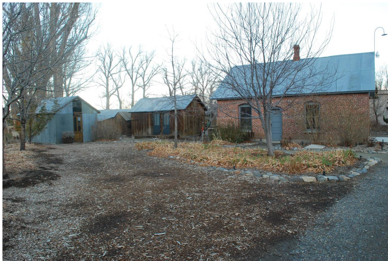
Photograph 2 – Example of cluster arrangement, showing Creamery (right), Bunk Shed (center), and Workshop (left), looking northeast.
