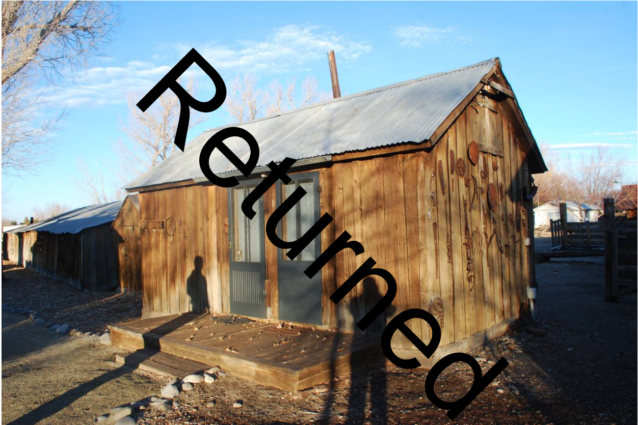
Photograph 10 – Bunk Shed, west façade and south elevation, looking northeast.
