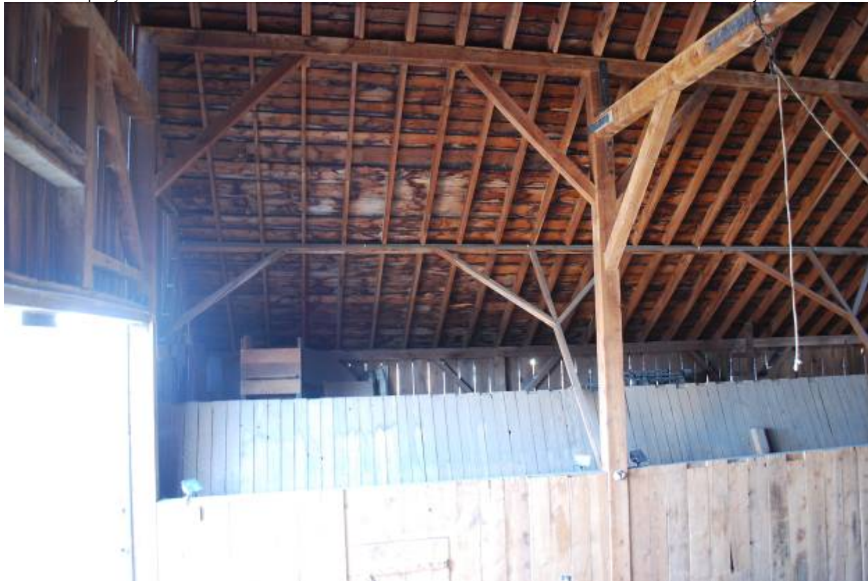
Photograph 27 – Barn roof framing system, showing dropped tie beam (upper right and left) and unique angled truss bracing system along secondary (lower) purlin.
