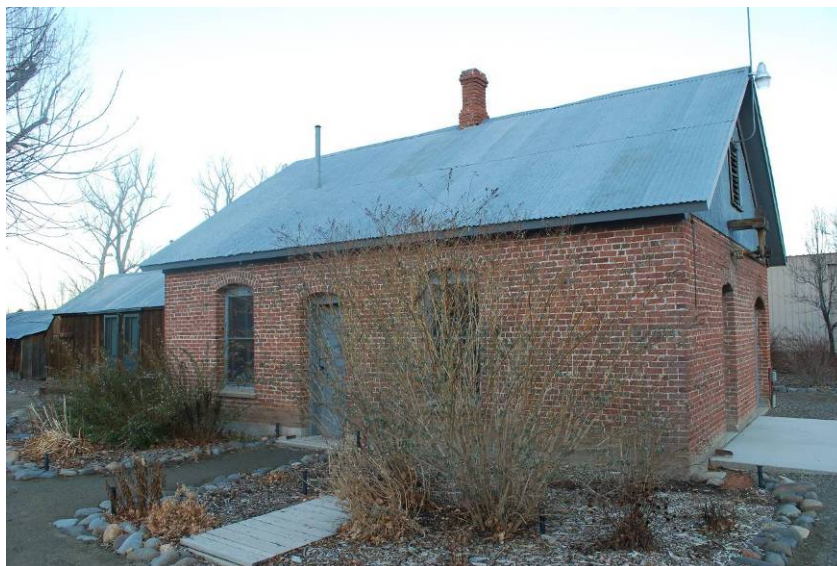
Photograph 9 – Creamery, west elevation, looking northeast. Note the belt-driven assembly in the gable end above the entrance (far right). The bunk shed can be seen at the far left behind (north of) the Creamery.
