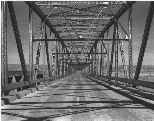
Photograph 0002. Yellowstone River Bridge. View to the east.
