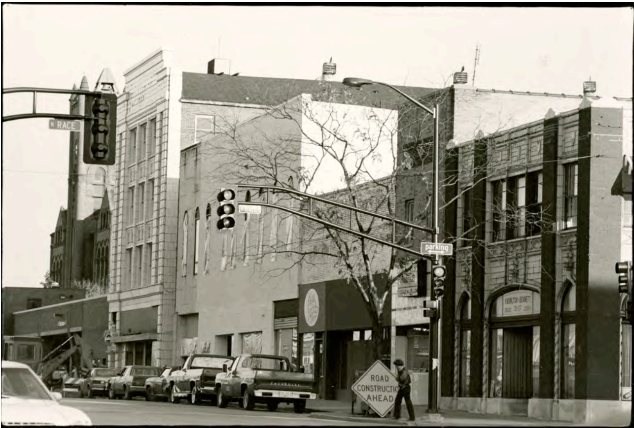
6. C 1985 looking east at south side W Main
