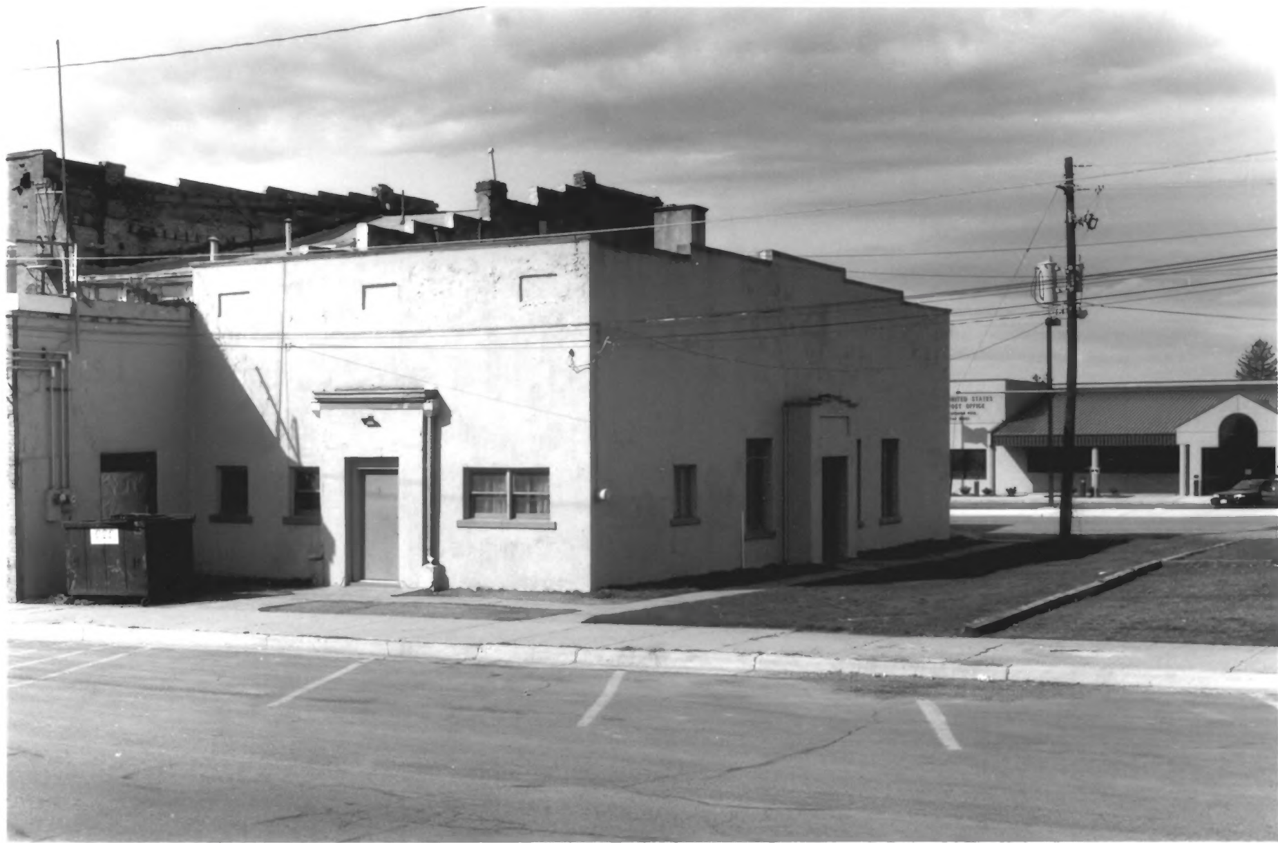
LEGION MEMORIAL BUILDING AMERICAN FORK, UTAH CO., UTAH PHOTO #1
