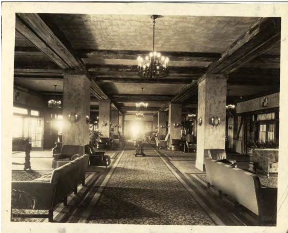
Figure 9. The hotel's lobby shortly after opening. Note rusticated woodwork, boxed beams, plaster ceiling and walls, and wall sconces, all of which are remain intact.
