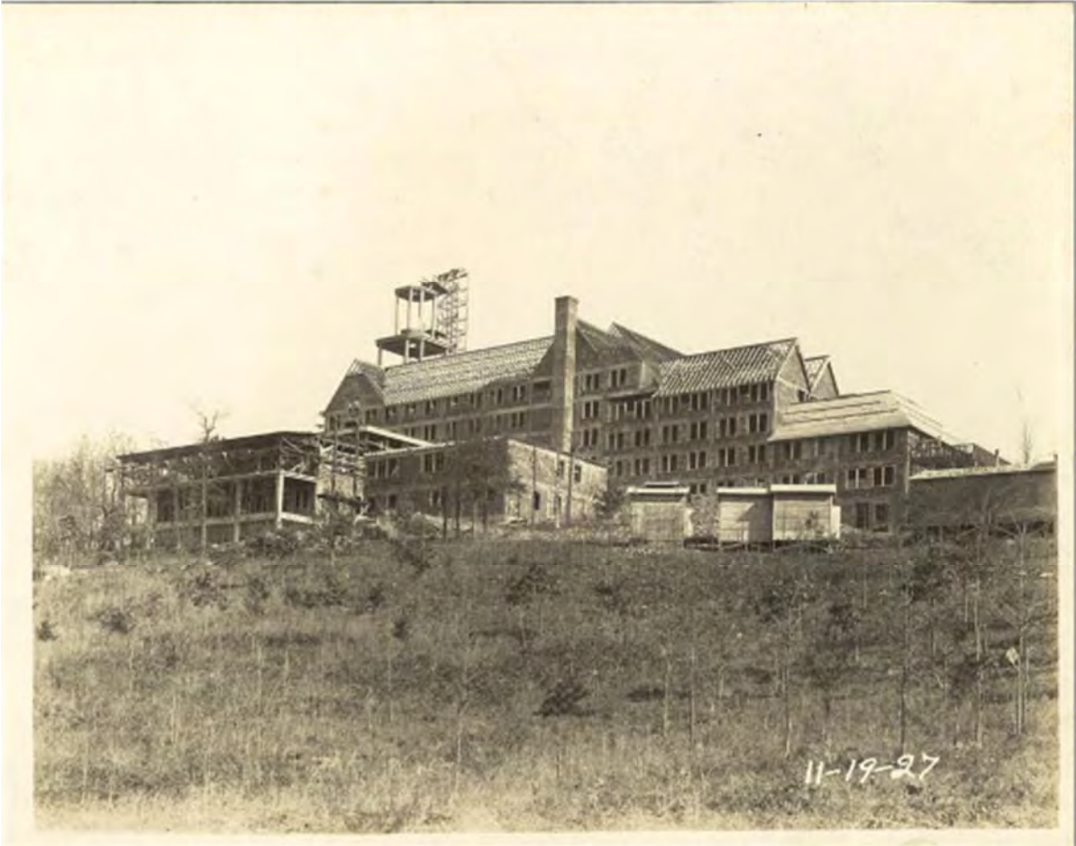
Figure 2. Lookout Mountain Hotel under construction in 1927.
