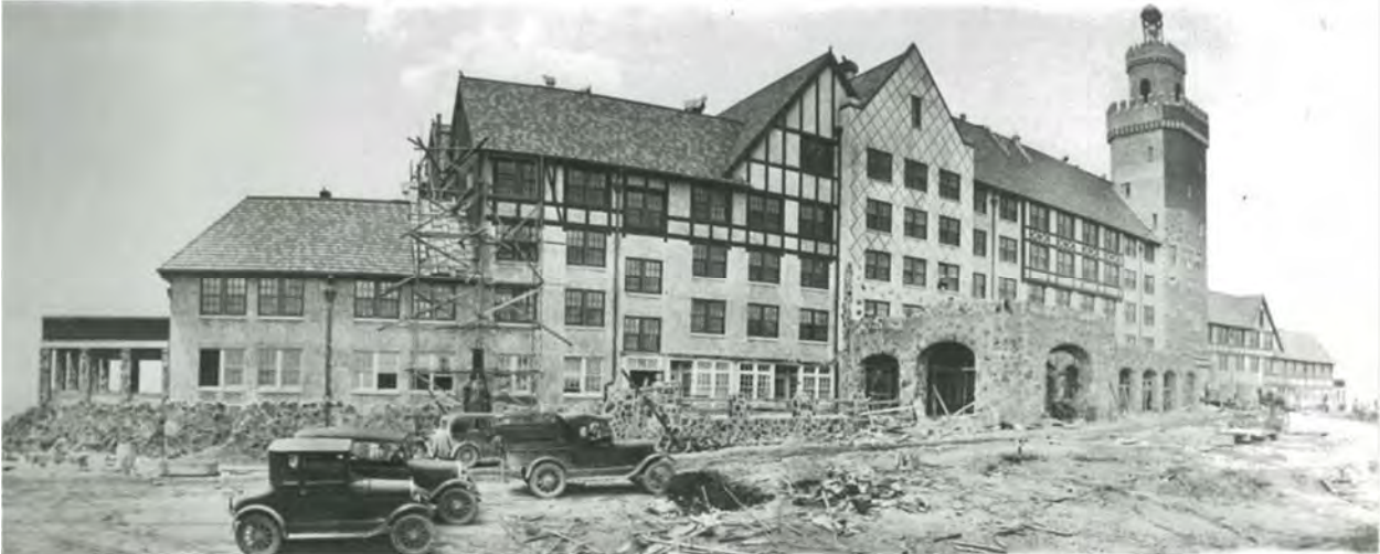
Figure 1. Lookout Mountain Hotel under construction in 1927.
