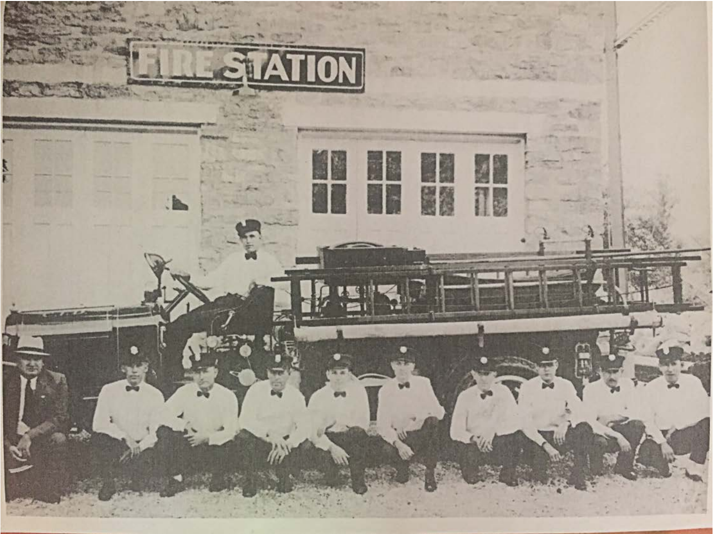
Figure 6: Historic photograph of the Old Fire Station, date unknown, showing original bay doors. Source: Brenda Owen, Chester, Illinois.
